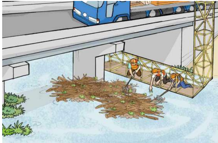
Figure 4-13 Removal of Drift Wood around Piers
