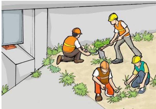
Figure 4-12 Removal of Grass and Shrubs near the Bridge
