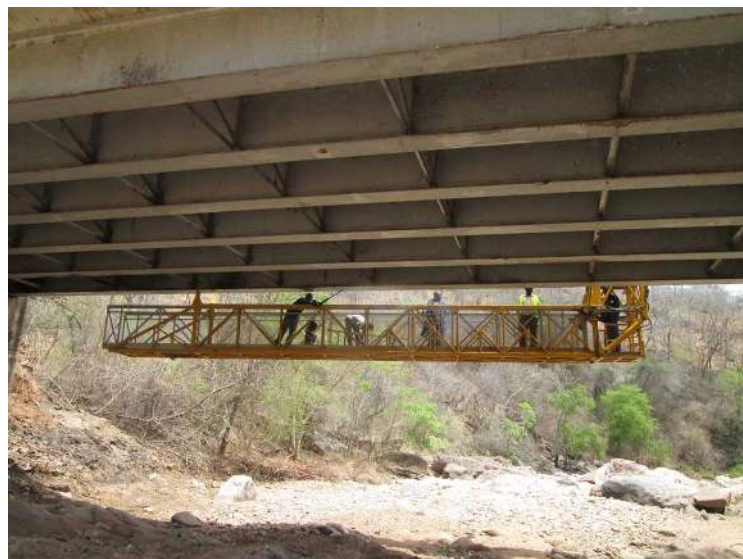
Photo 4-3 Cleaning of Steel Girder
