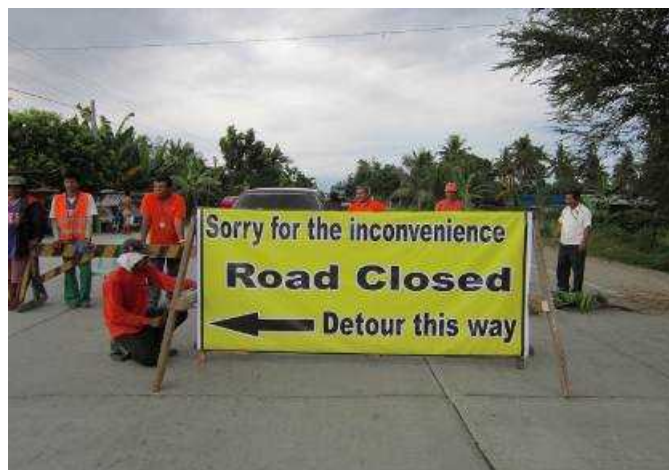
Photo 6-1 Warning signs and Barricades
