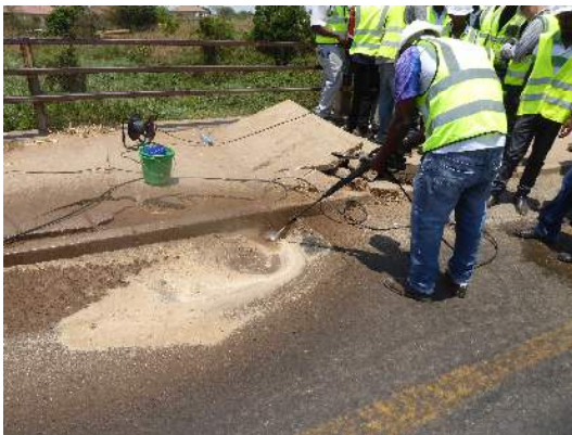
Photo 4-7 Cleaning of the Deck Slab and Its Drainage Inlet
