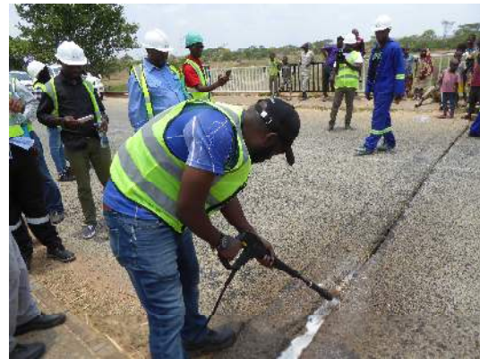
Photo 4-8 Cleaning expansion joint with high pressured water
