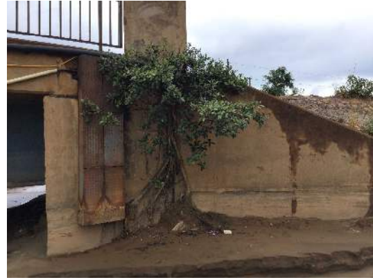
Photo 4-9 Vegetation on the Substructure
