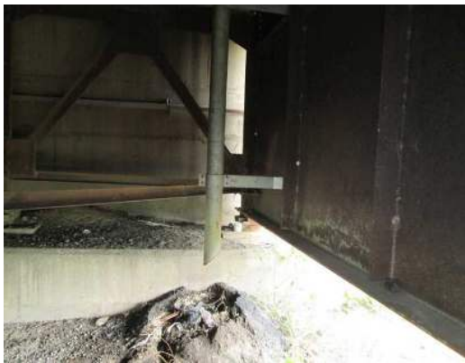
Photo 4-9 Accumulated dirt around abutment may hamper the drainage
