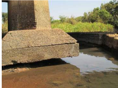
Photo 4-19 Exposed Pier Footing
