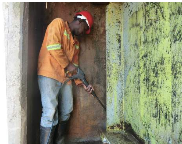
Photo 4-9 Accumulated dirt around abutment may hamper the drainage
