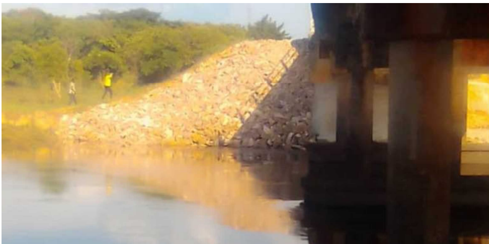
Photo 6-3 Repair around abutments
