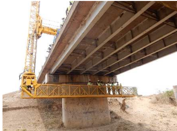
Photo 4-2 Cleaning using Inspection Vehicle
