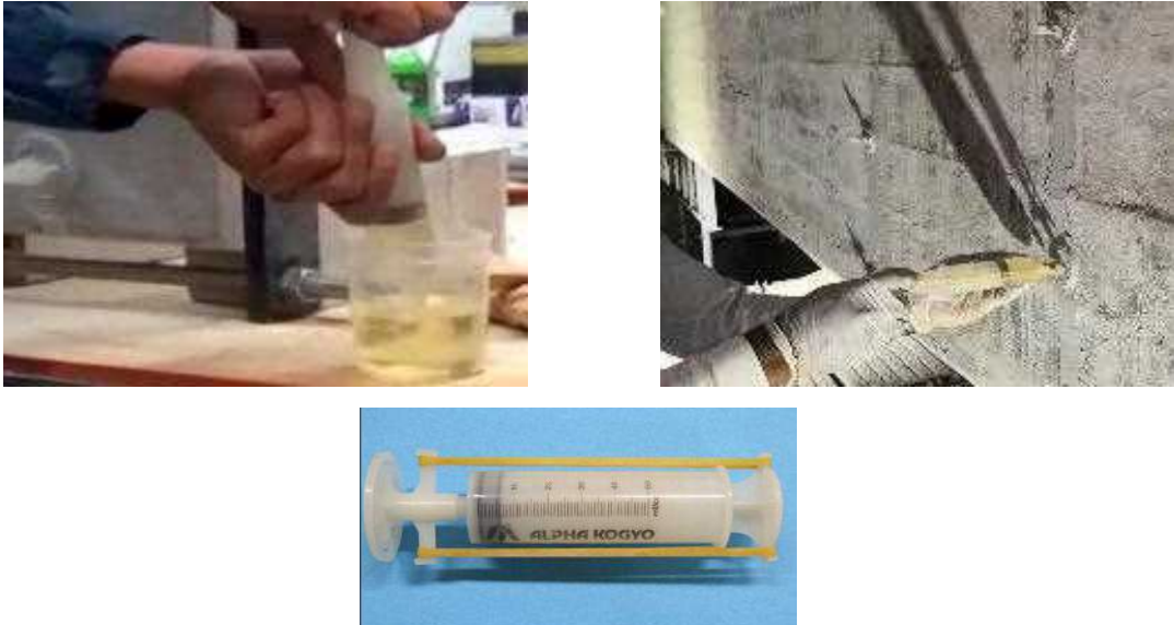
Figure 4-9 Crack Injection Method
