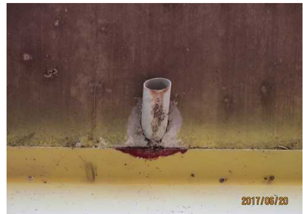
Photo 4-15 Deterioration at drain locations
