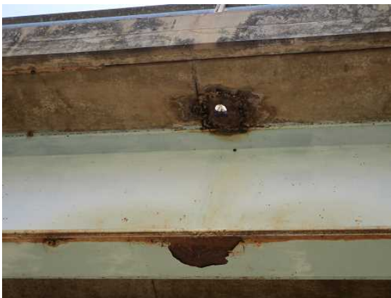
Photo 4-15 Deterioration at drain locations
