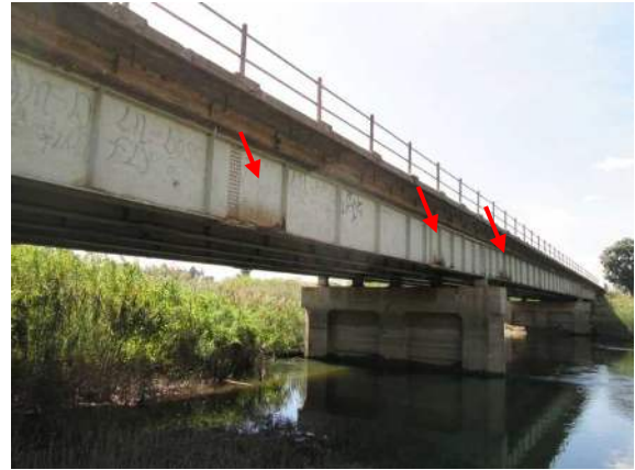
Photo 4-13 Deterioration at drain locations
