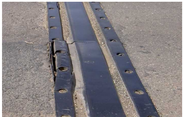
Figure 8-45 Rupture
