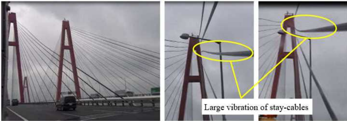
Figure 2-7-9 Example of rain vibration
