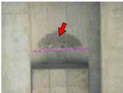
leakage from joints between primary and secondary floor slabs of continuous composite girders
