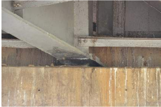
Figure 5-26 Inspect Rubber Bearing
