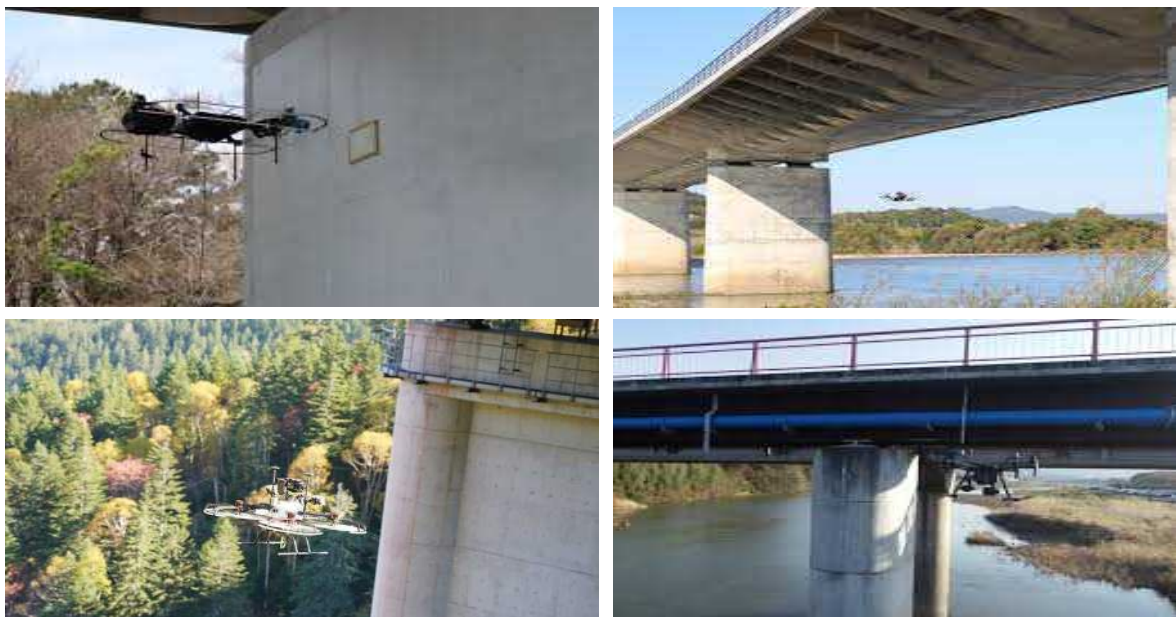
Photo 10-8 Status of bridge inspection by drone (Japan)
