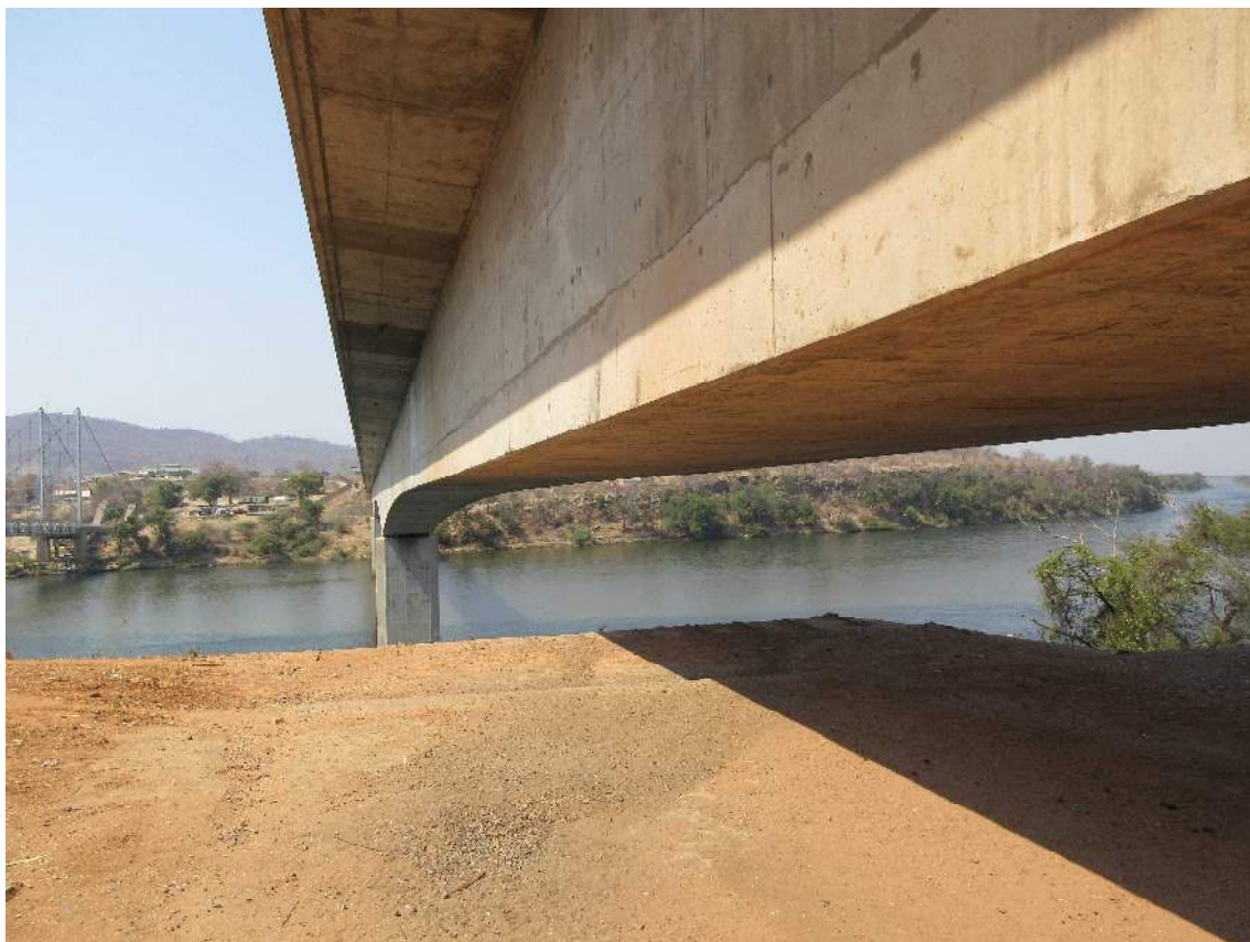
Figure 1-2-1 Photo of Chirundu Bridge
