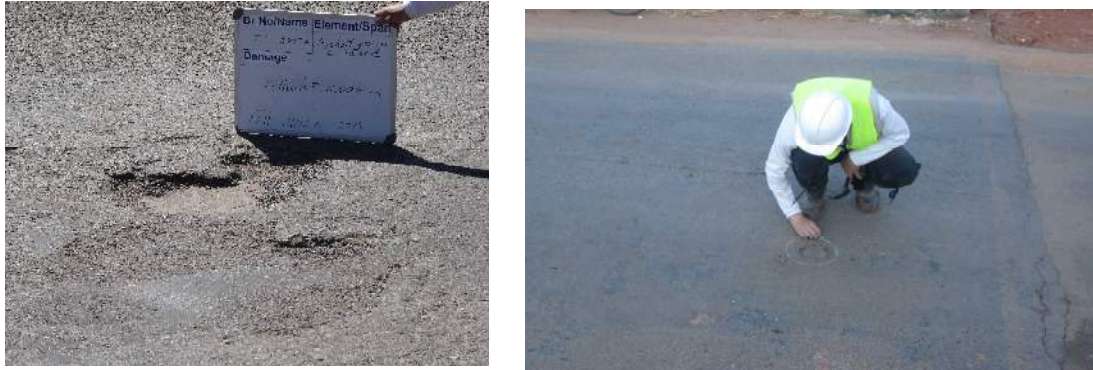
Figure 5-7 Inspect of the Pavement
