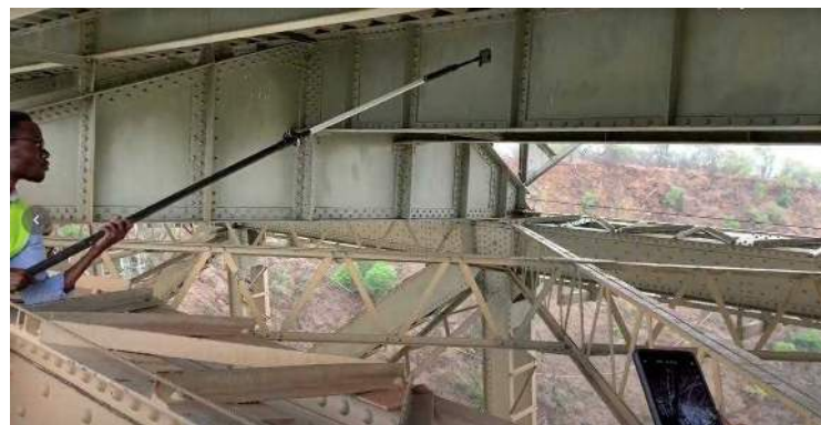
Photo 10-17 Interior areas of bridge capture using 360 camera mounted on range pole
