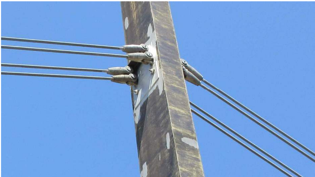
Figure 2-7-3 Stay cable anchor in Luangwa Bridge (tower side)
