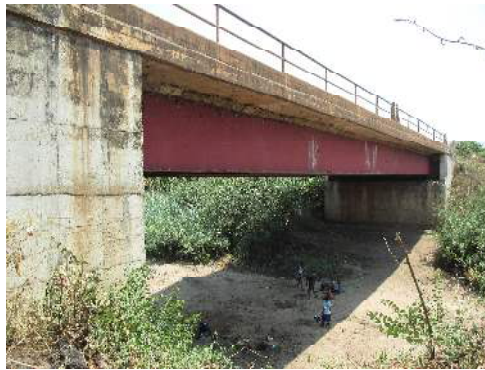
Figure 5-20 Inspect Entire Steel Structure
