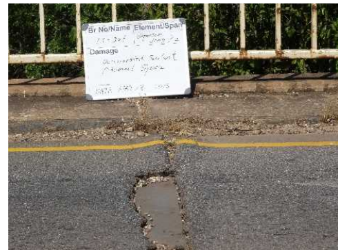
Figure 8-49 Deteriorated Sealant
