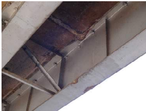
Figure 5-21 Inspect Center of Span
