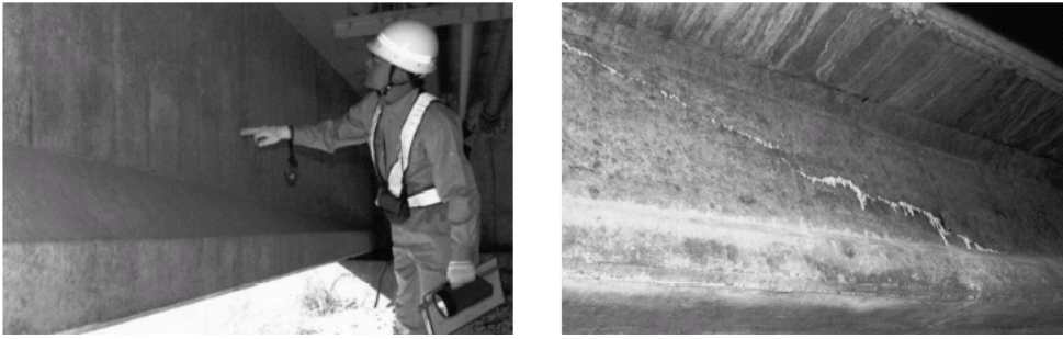
Figure 5-13 Inspect Concrete Girder at 1/4 Point of Span
