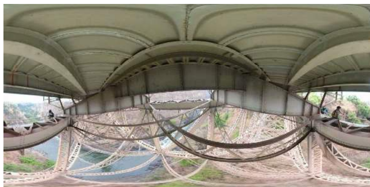
Photo 10-18 Raw 360 image of an interior section of bridge
