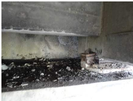
Figure 5-28 Inspect Anchor Bolts of Bearings
