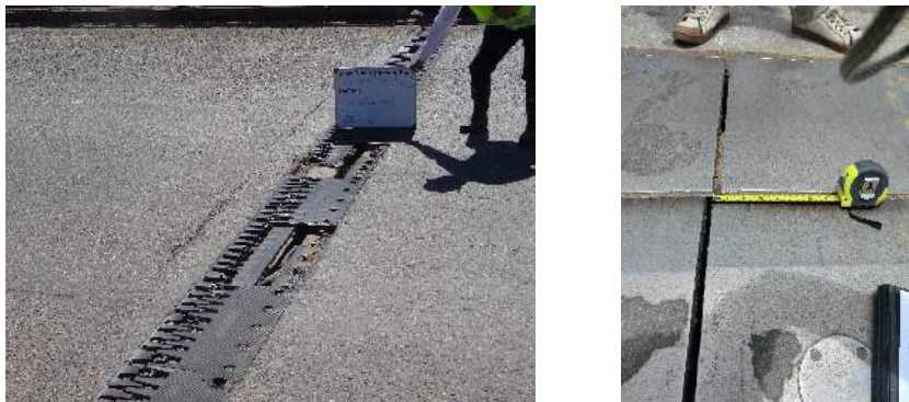
Figure 5-8 Inspect Expansion Joint
