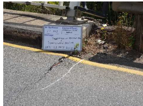
Figure 8-48 Difference in Elevation
