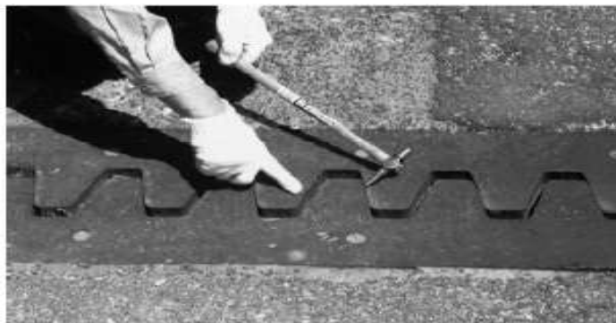
Figure 8-40 Difference in Elevation
