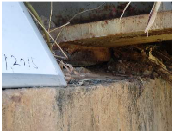
Figure 5-27 Inspect Bearing Mortar
