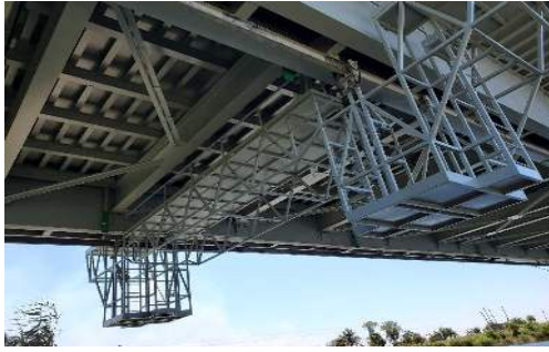
Cable-stayed bridge (Mozambique)
