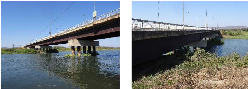
Figure 5-5 Inspection Side View
