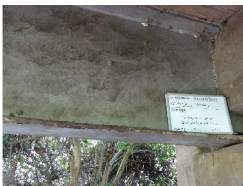
Figure 5-22 Inspect Ends of Girders
