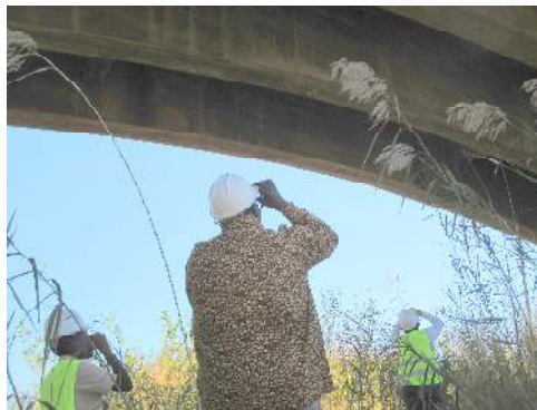
Figure 5-11 Inspect Concrete Girder (Center of Span)
