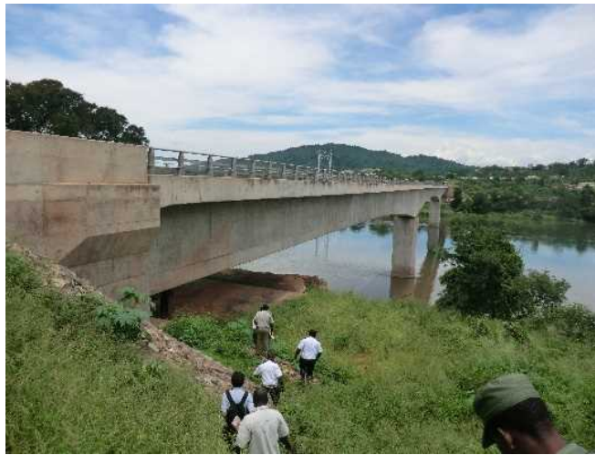
Figure 1-1-1 PC BOX Bridge
