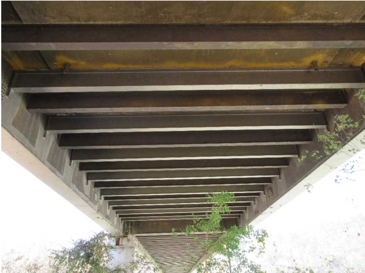
Figure 2-7-5 Two Box girders in Luangwa Bridge
