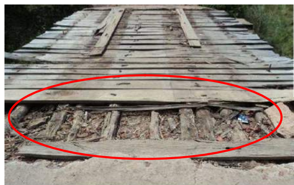
Figure 8-20 Disconnection of Timber Deck
