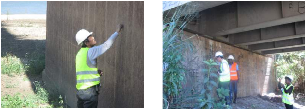
Figure 5-17 Inspect Abutments and Piers
