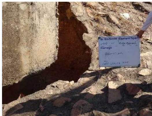
Figure 8-34 Bank Erosion
