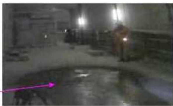
leakage from the upper slab and dripping-down to the lower slab
