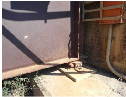
Figure 5-23 Inspect Supporting Points of Structure Steel
