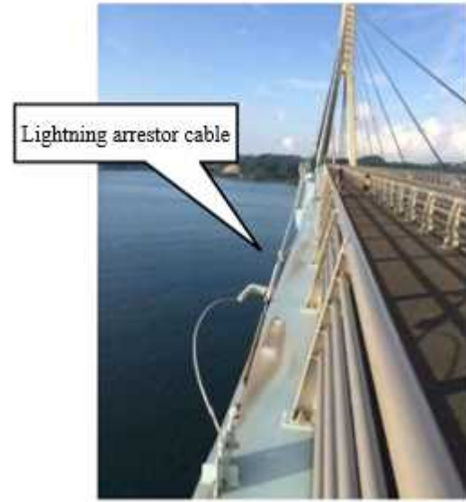
Figure 2-7-13 Example of lightning arrester cable installation
