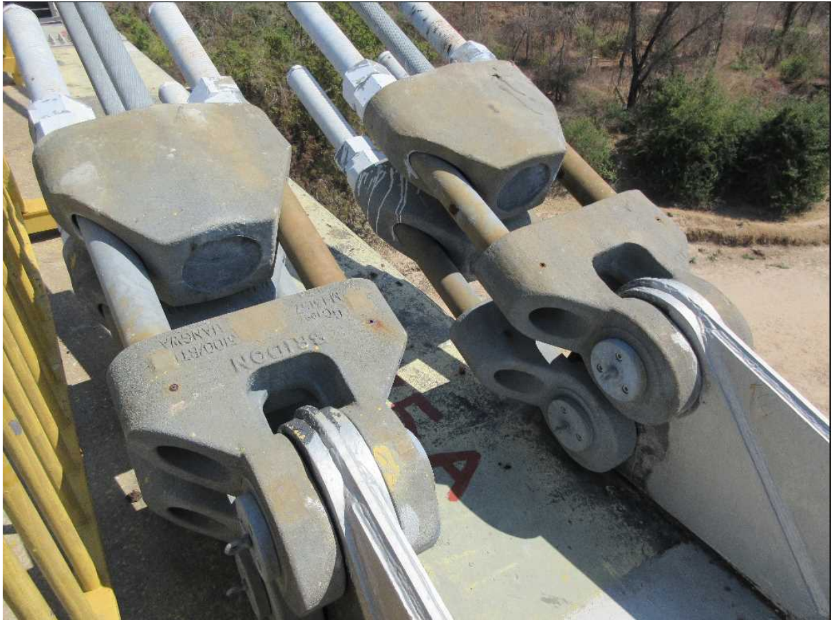
Figure 2-7-2 Stay cable anchor in Luangwa Bridge (girder side)
