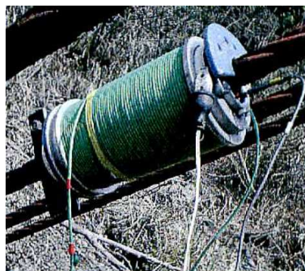
Figure 3-4-3 Inspection Device of Main Flux Method
