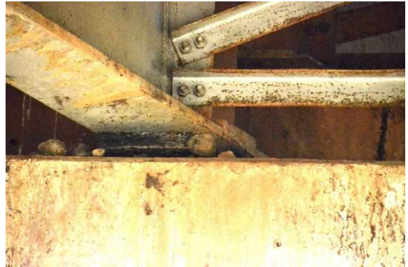
Figure 8-24 Bulging Bearing
