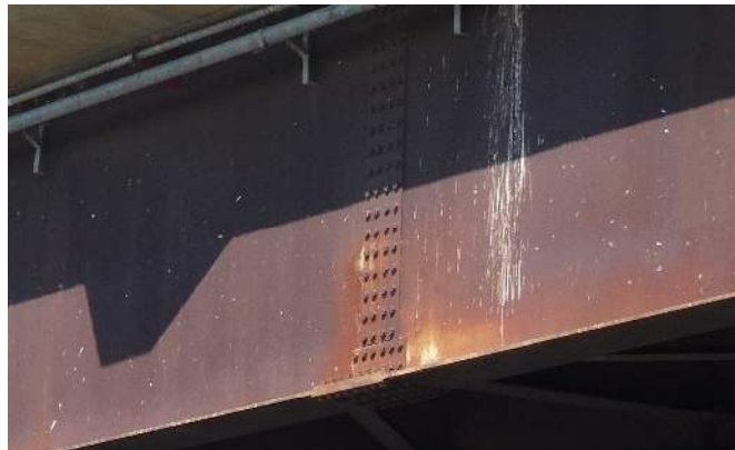
Figure 5-24 Inspect Splice Plates of Steel Structure
