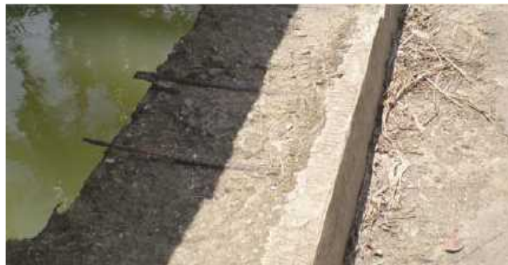
Figure 5-6 Inspection the Curb
