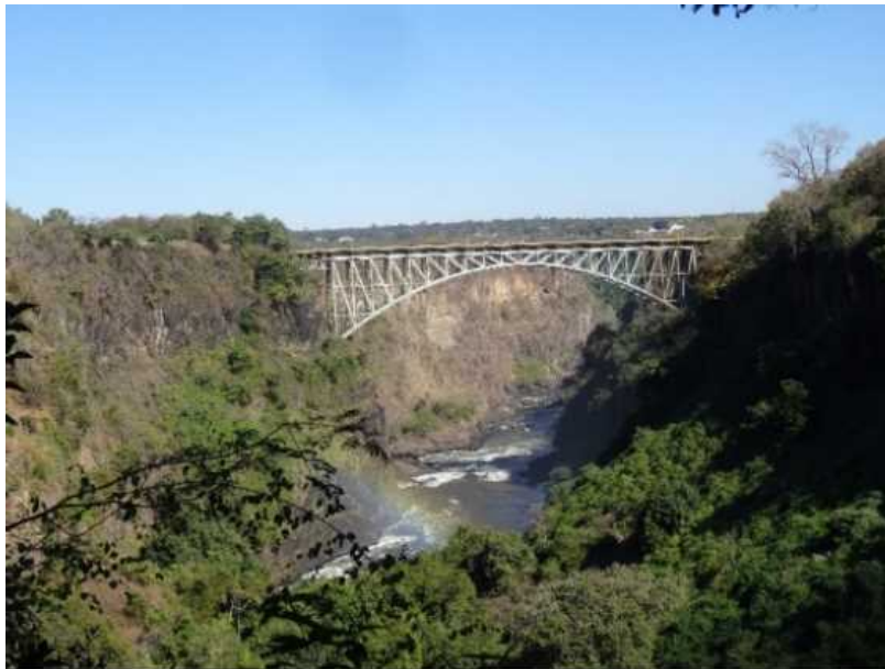
Figure 4-1-1 Steel Arch Bridge
