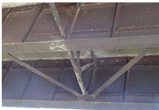
Figure 5-25 Inspect Cross Beam
