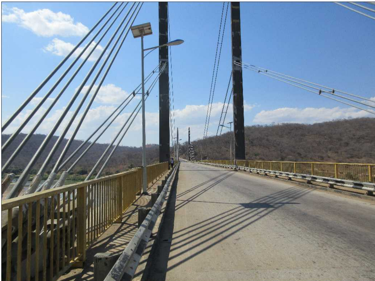
Figure 2-7-1 Stay cable in Luangwa Bridge
