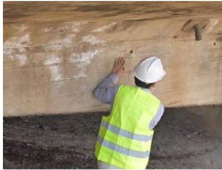
Figure 5-10 Inspect All Concrete Girders
