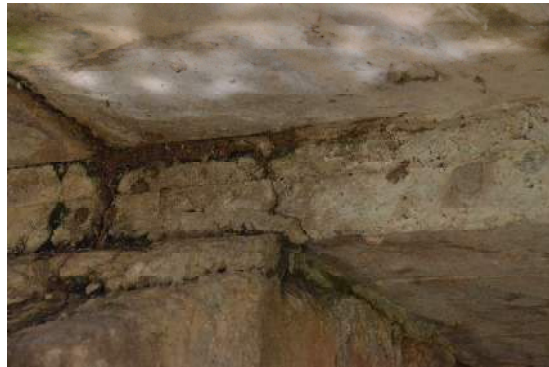
Figure 5-15 Inspect Concrete Girder at Supporting
