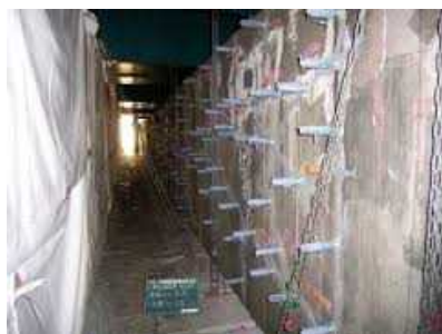
Figure 4-1 Crack Injection Method
