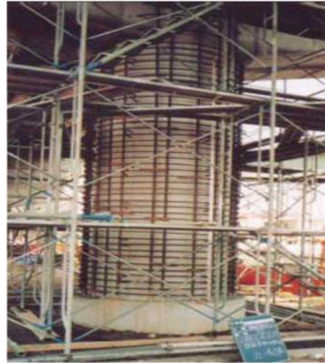
Photo 6-2 Concrete Jacket for Repair Pier
