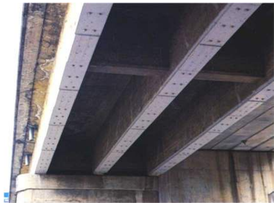
Figure 4-12 Repair of Concrete Girder by Steel Plate Bonding
