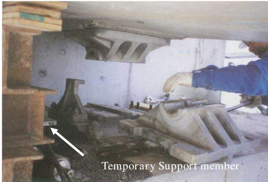
Photo 8-2 Sample of Replacement Bearing by Jack-up Girder
