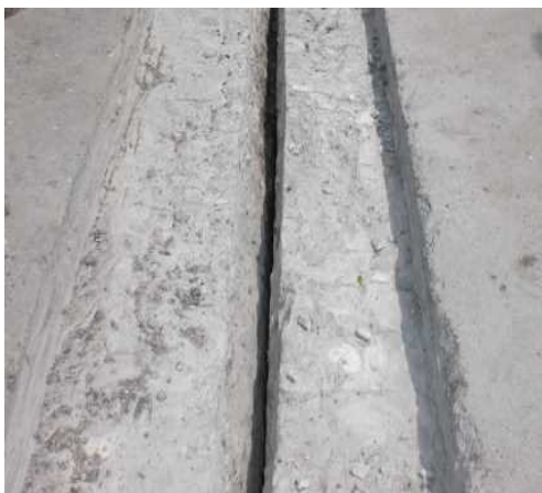
Photo 7-1 Cleaning of the gap
