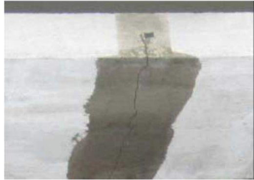
Photo 4-1 Epoxy Coating Penetrating into the Crack
