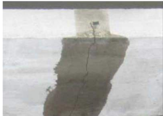
Photo 3-1 Epoxy Coating Penetrating into the Crack
