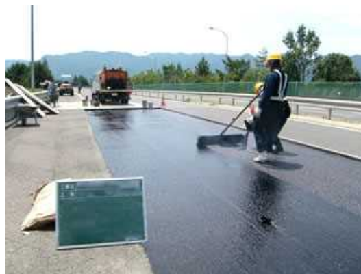
Photo 3-3 Asphalt Compound Membrane System
