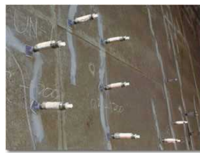
Figure 4-1 Crack Injection Method
