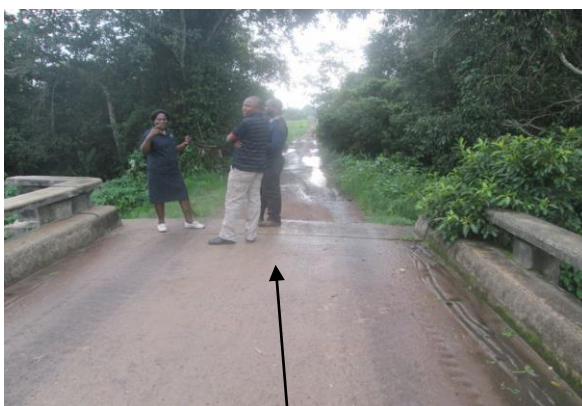
End of project road (Ch327+400) at Jimbe Bridge in Jimbe-Ikelenge District
