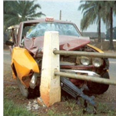
Badly designed bridge railing
