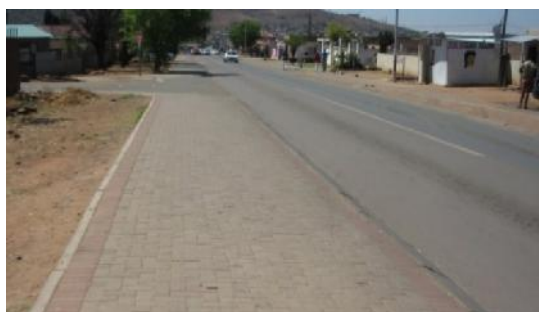
Figure 6-4: Wider than normal sidewalk
