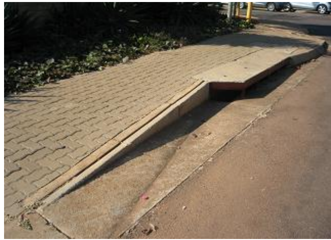
Figure 5-4: Kerb inlet
