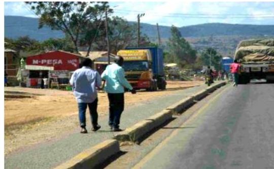
Segregated shoulder using barrier curb
