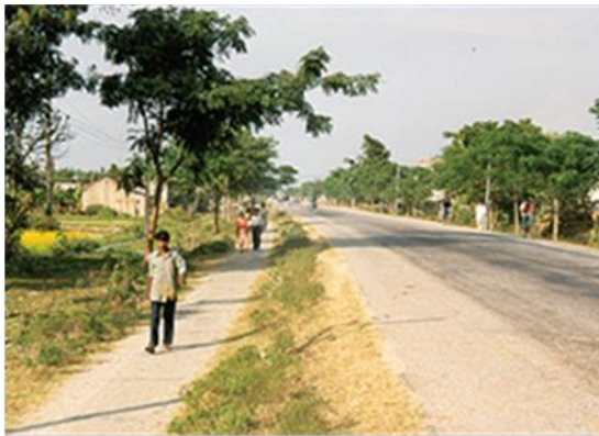
Segregated footpath off main road
