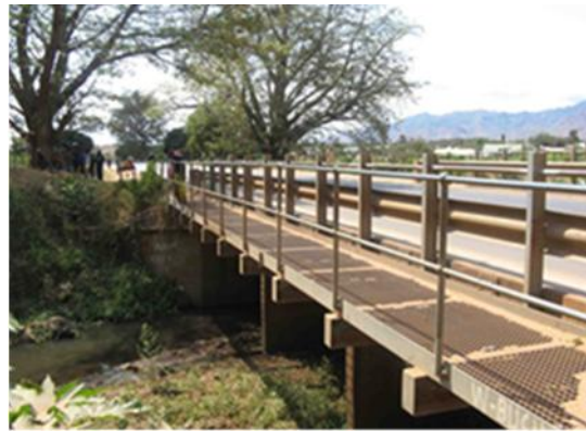
Segregated footpath on narrow bridge
