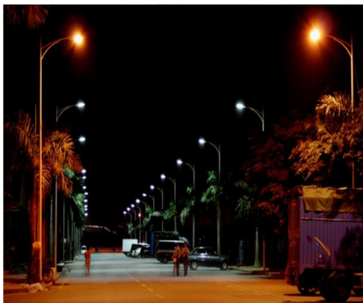
Figure 4-19: Sodium lamp (nearside) and LED (far side)
