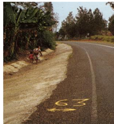
Well designed side drain
