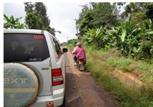
Figure 3-4: Typical problems encountered on rural roads
