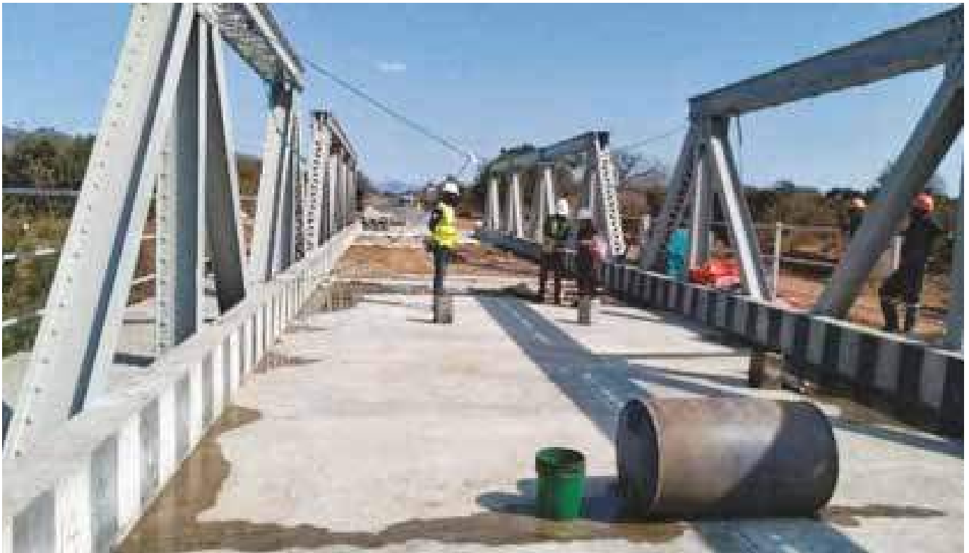
Figure 3.10: Repair works at Rufunsa Bridge in Lusaka Province
