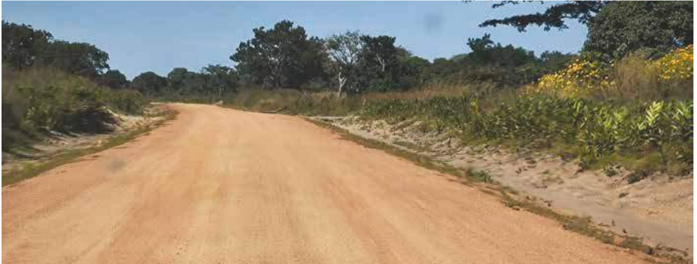
Figure 3.8: A completed primary feeder road under the maintenance phase in Samfya District in Luapula Province
