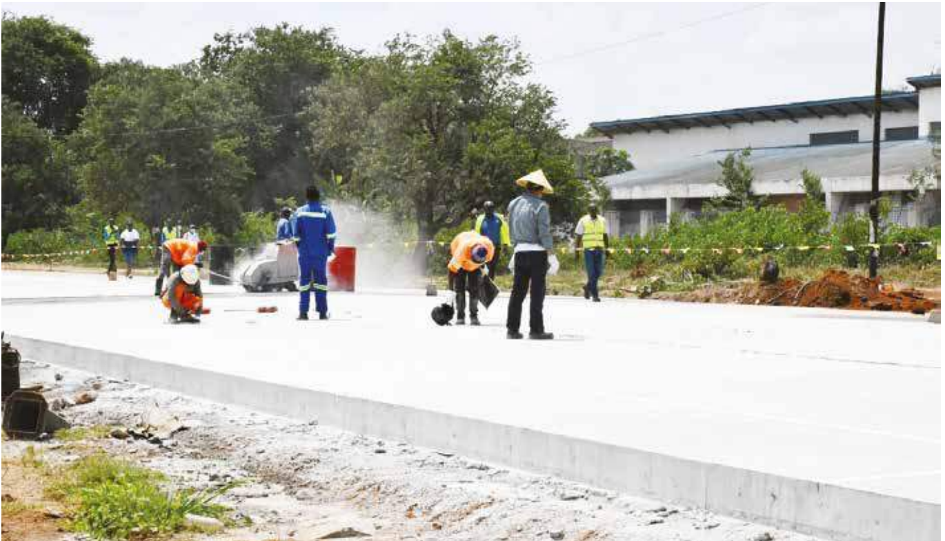
Figure 3.1: Construction works on the 2.5 kilometres dual carriageway in Ndola
