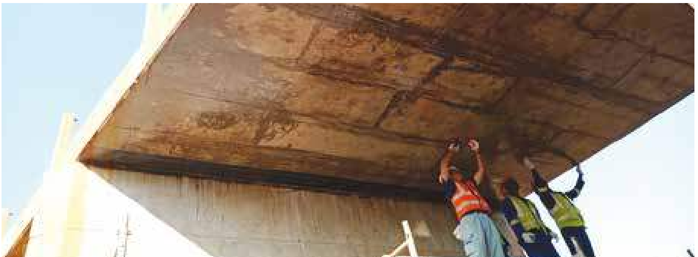
Figure 3.9: Repair works at Luena Bridge in Western Province
