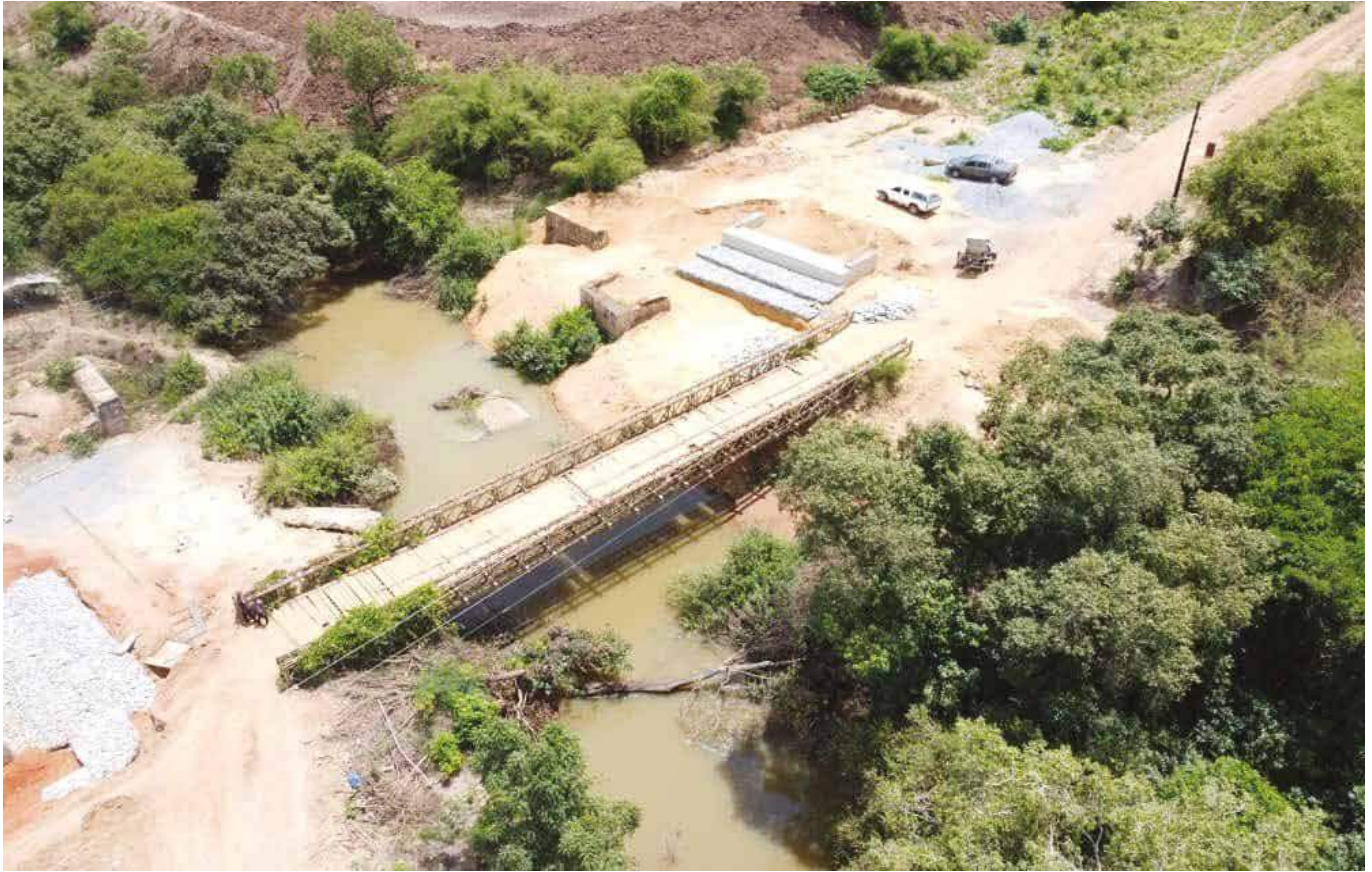
Figure 3.11: Luombwa Acrow Bridge under construction in Serenje District through Force Account
