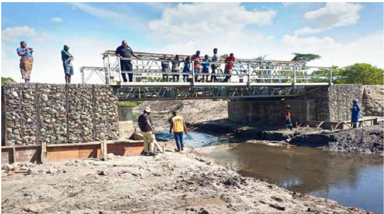
Figure 3.10: Kasombo ACROW Bridge in Kabompo District
