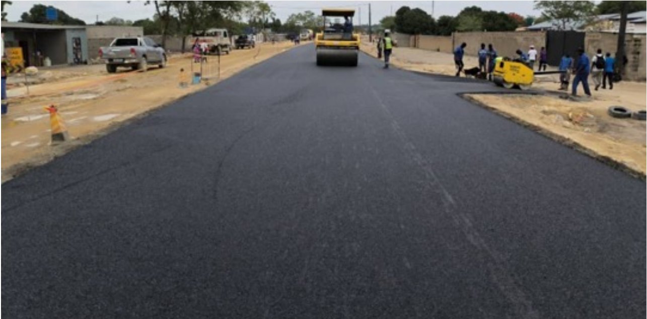
Figure: 3.7: Construction works under the Mongu-Limulunga Road Project
