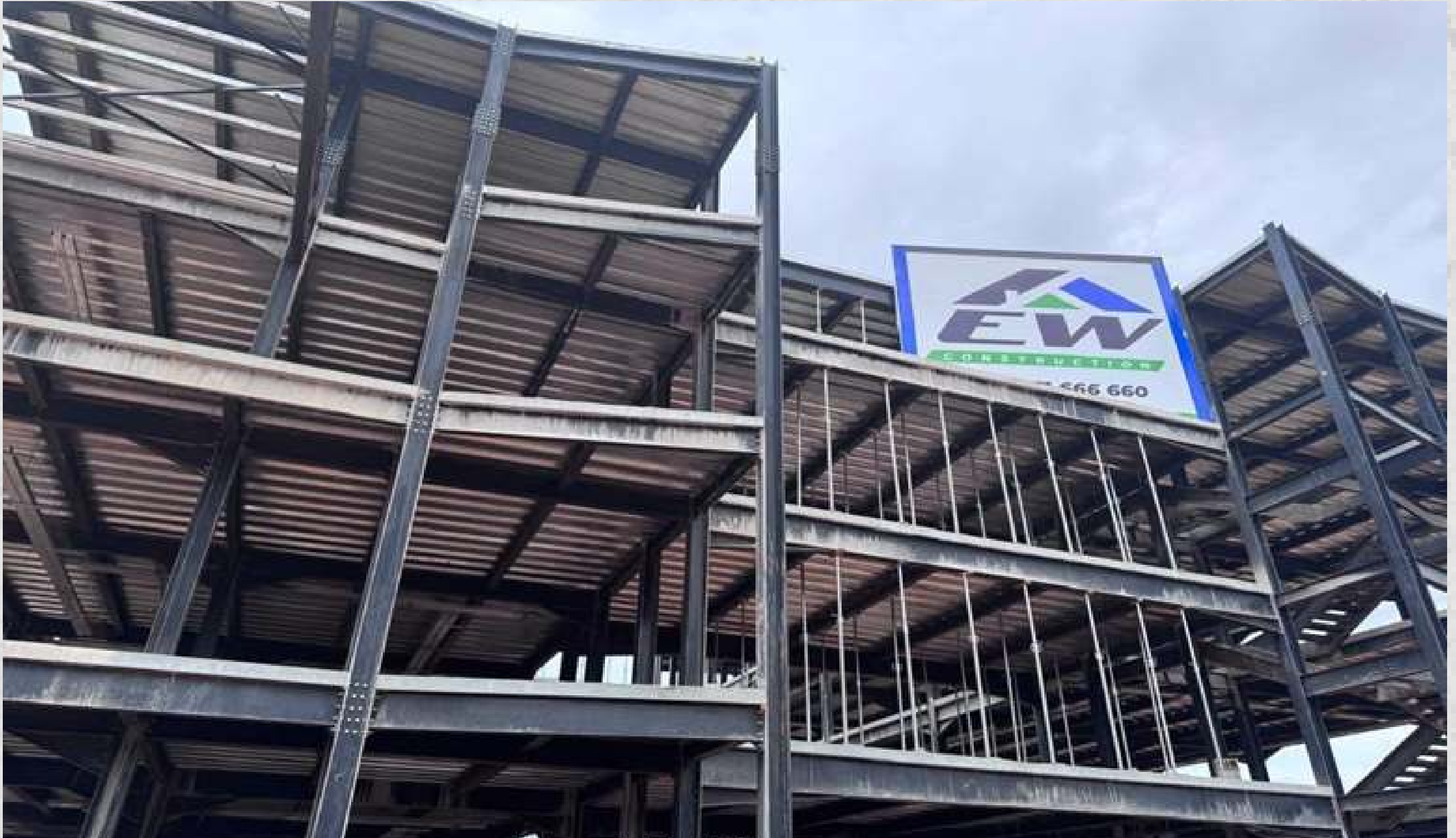
Kasumbalesa Border Post modernisation works in progress..
