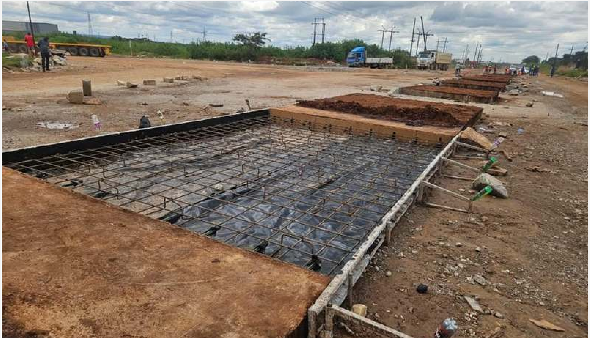
Concrete pavement works at Kalulushi - Sabina Junction.
