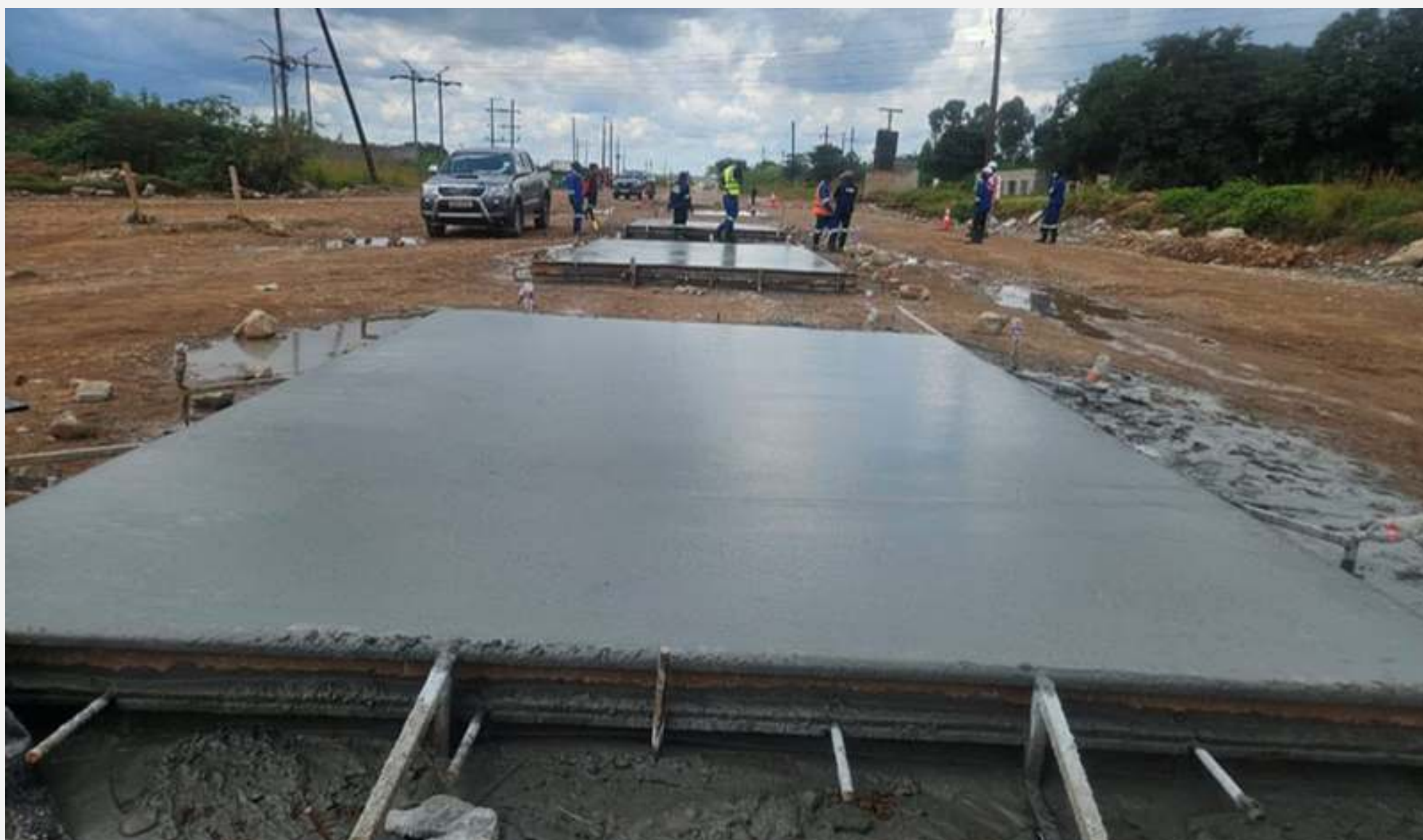
Concrete pavement works at Kalulushi-Sabina Junction.
