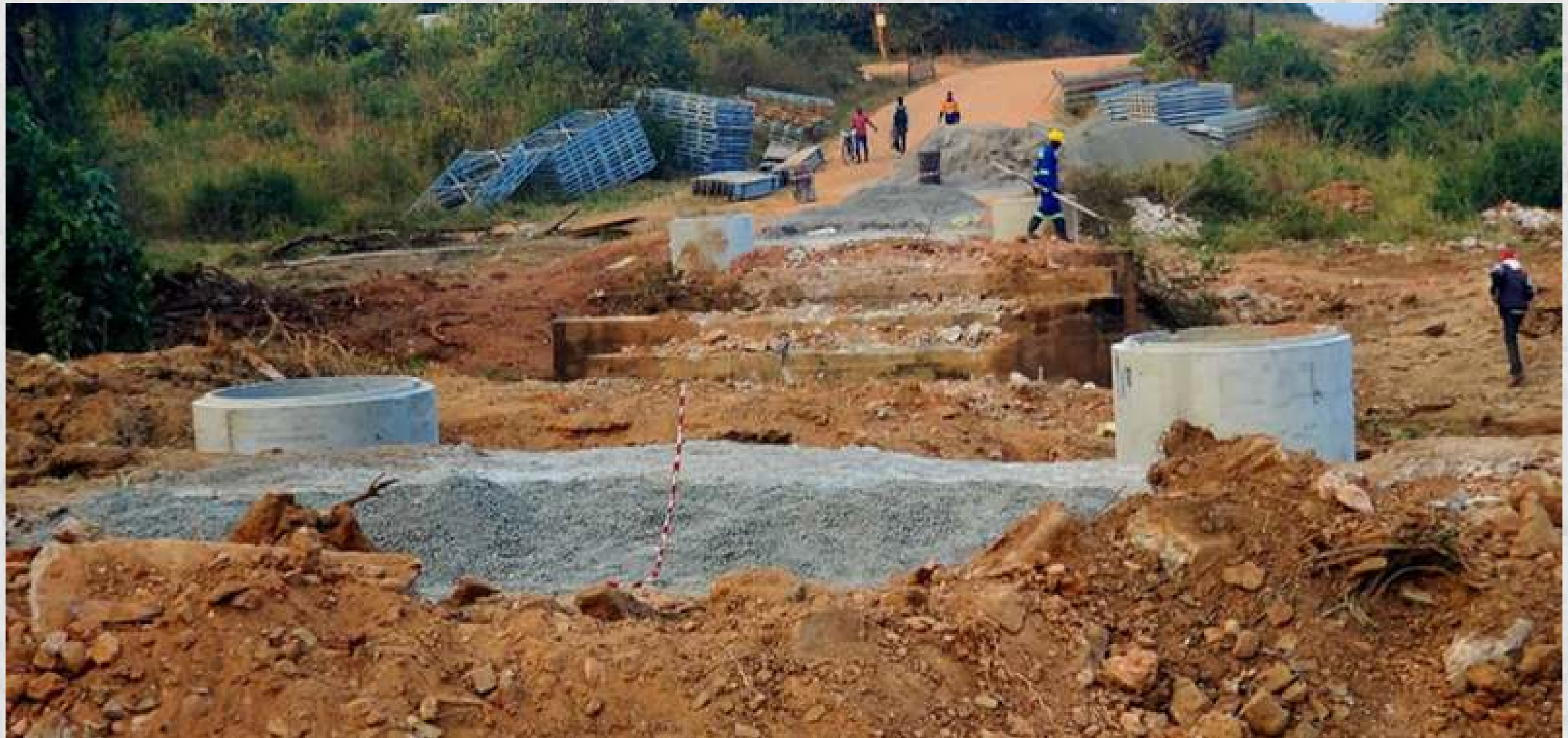
Construction of Mambulwe Emergency Acrow Bridge begins.
