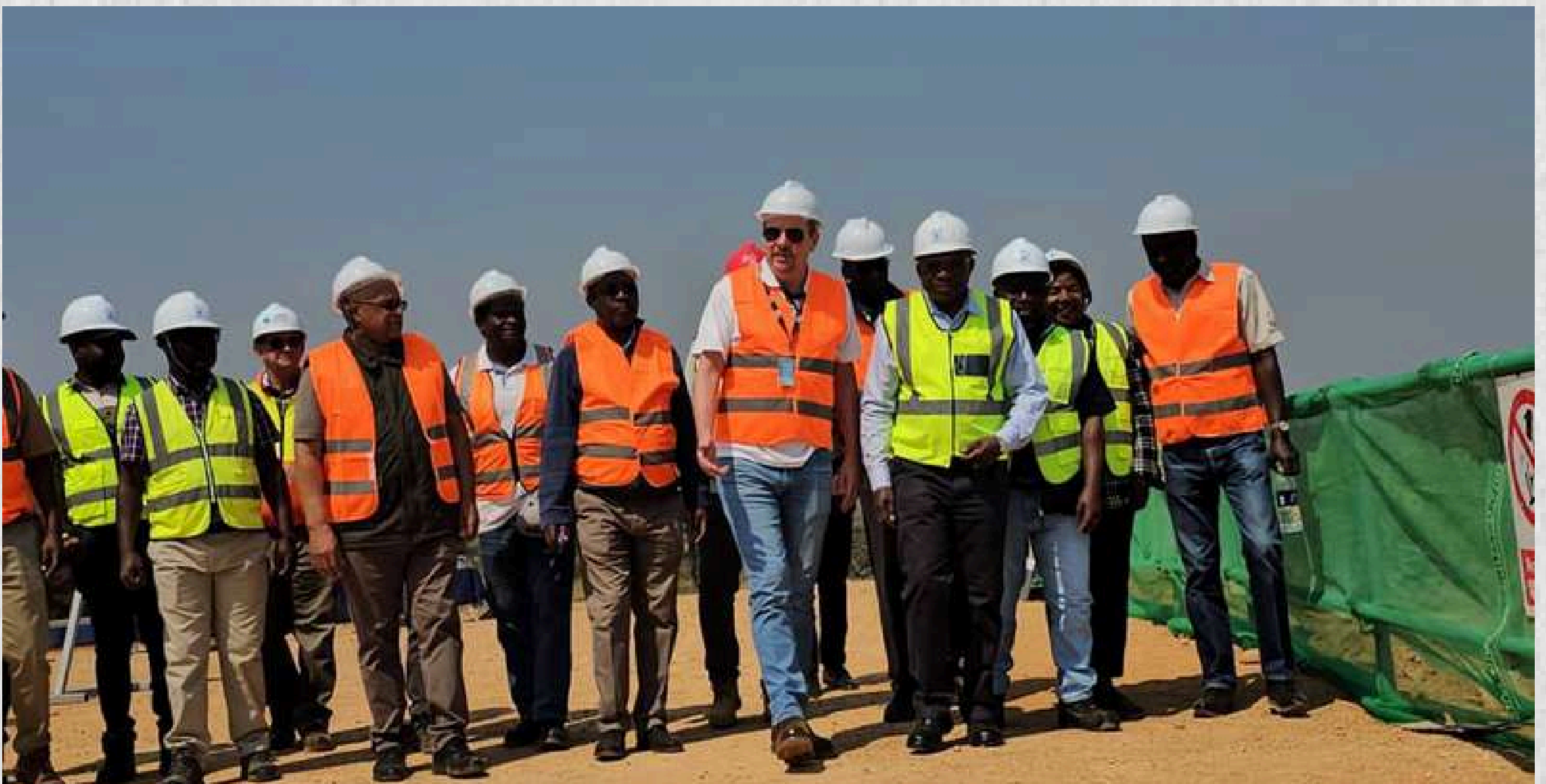
Infrastructure, Housing and Urban Development Minister, Hon. Eng. Charles Milupi led PPP Council, MIHUD and RDA Officials to inspect construction works of the Kasomeno-Mwenda Road and Bridge Project in Mwense District.
