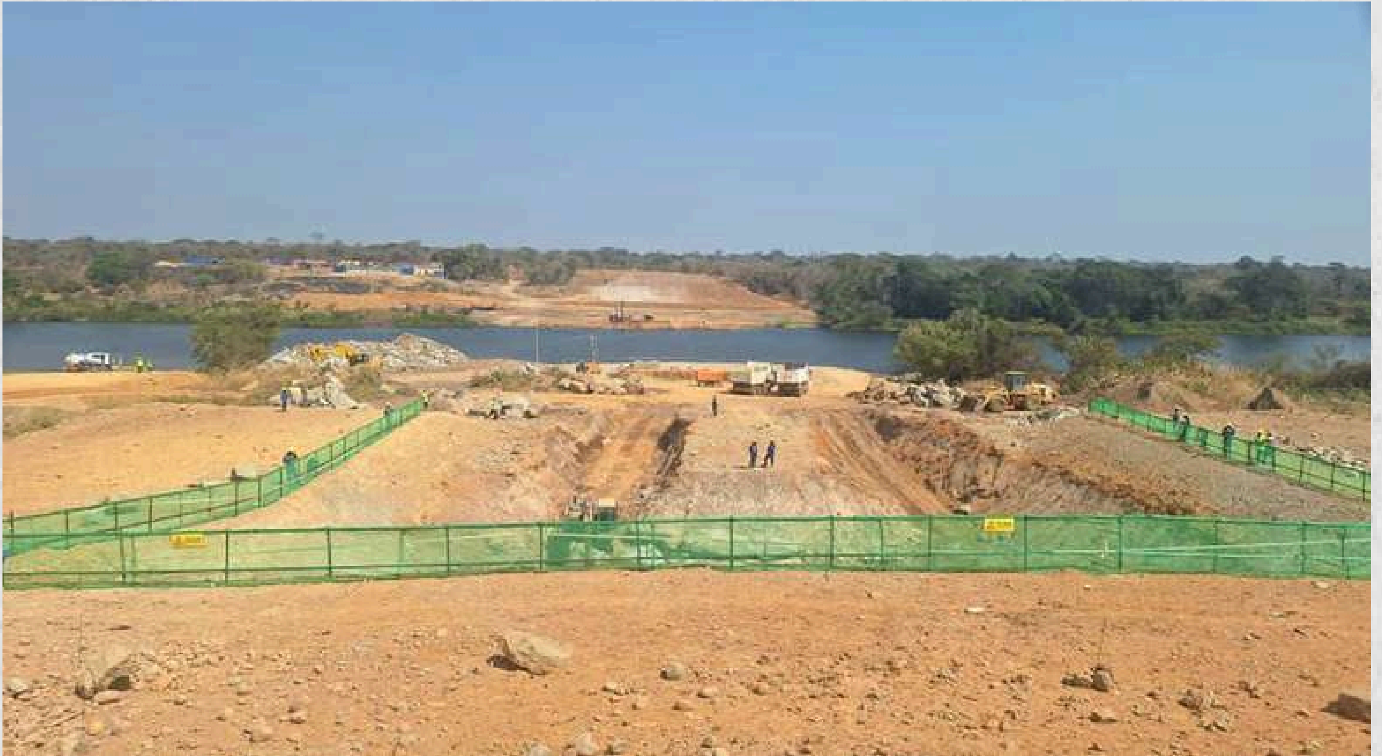
Preparatory works for the Kasomeno-Mwenda Road and Bridge.
