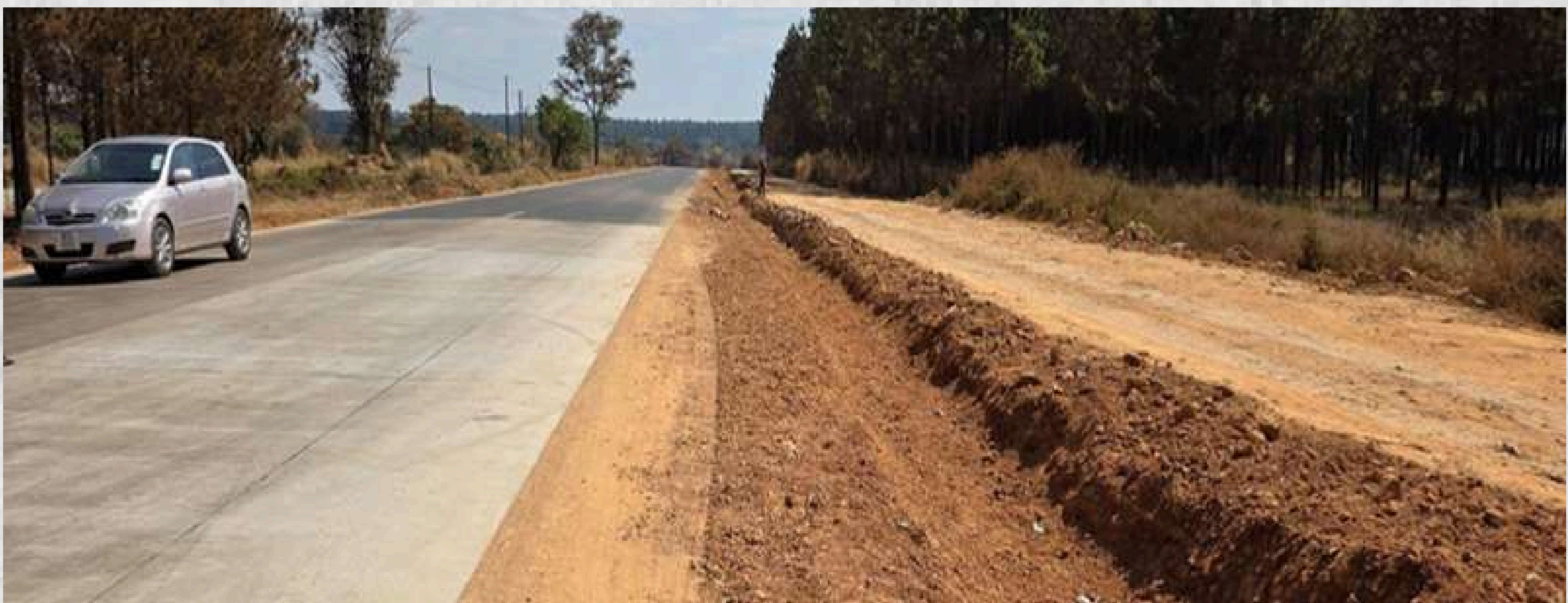
Rehabilitated section of the Ndola-Sakania-Mufulira Road.
