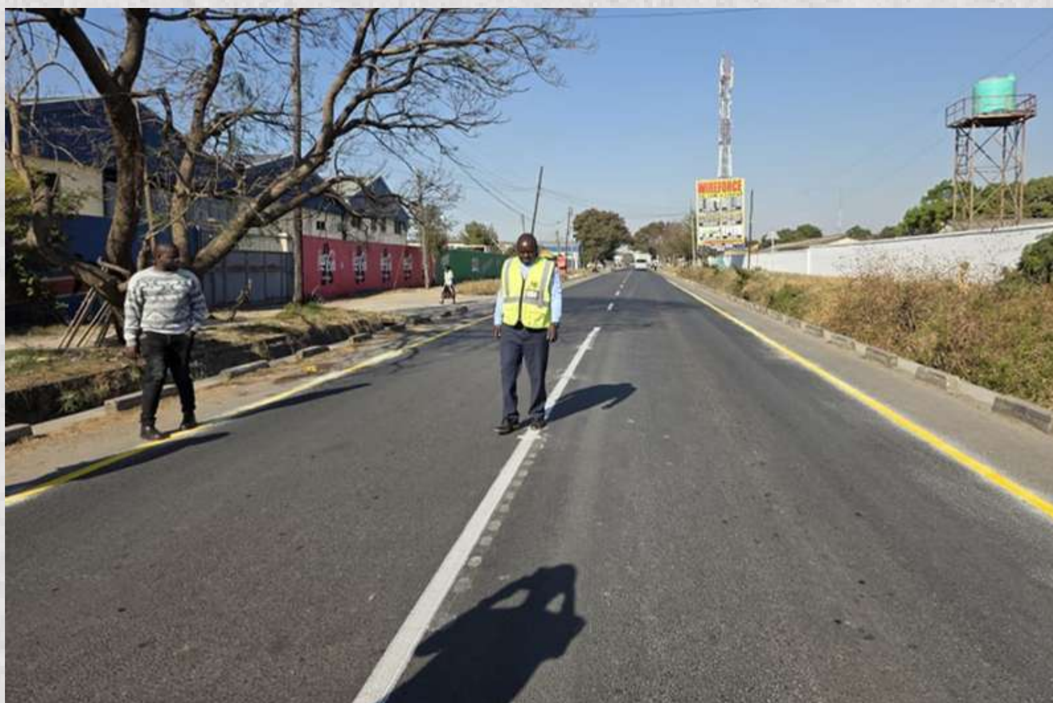
White road line- marking along Sheki -Sheki Road.
