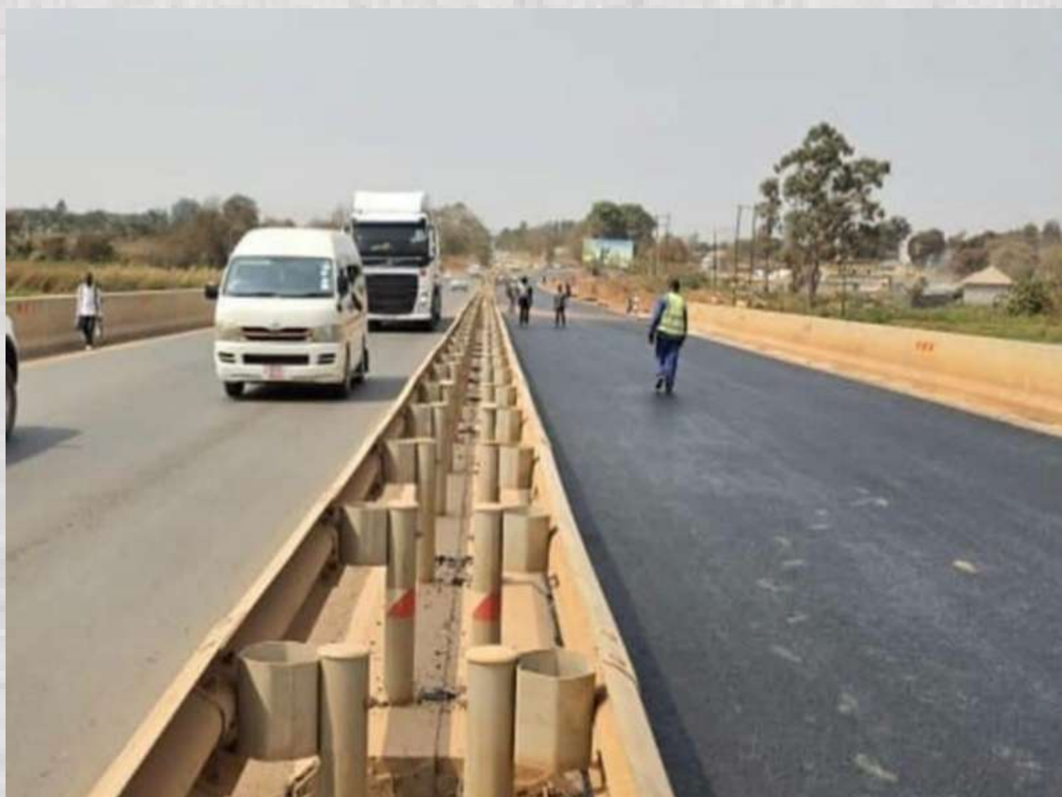
Asphalt pavement works at Kafubu Bridge.
