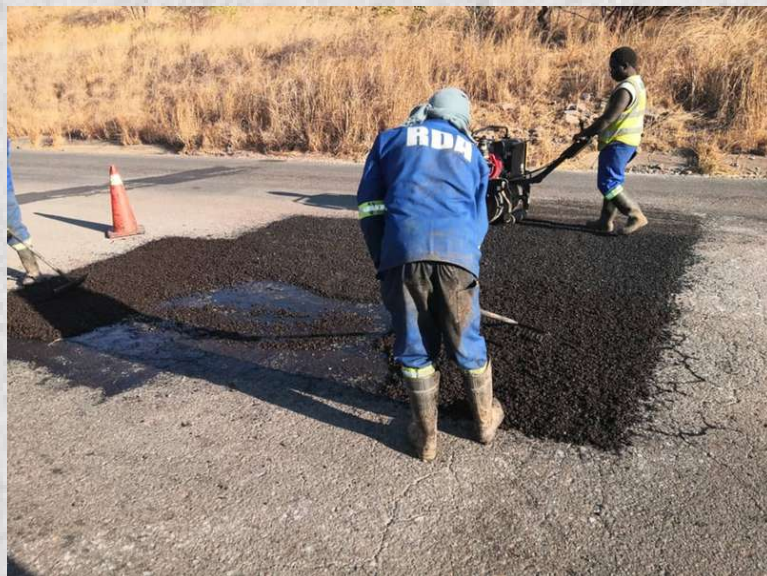
Compaction of the applied asphalt cement.
