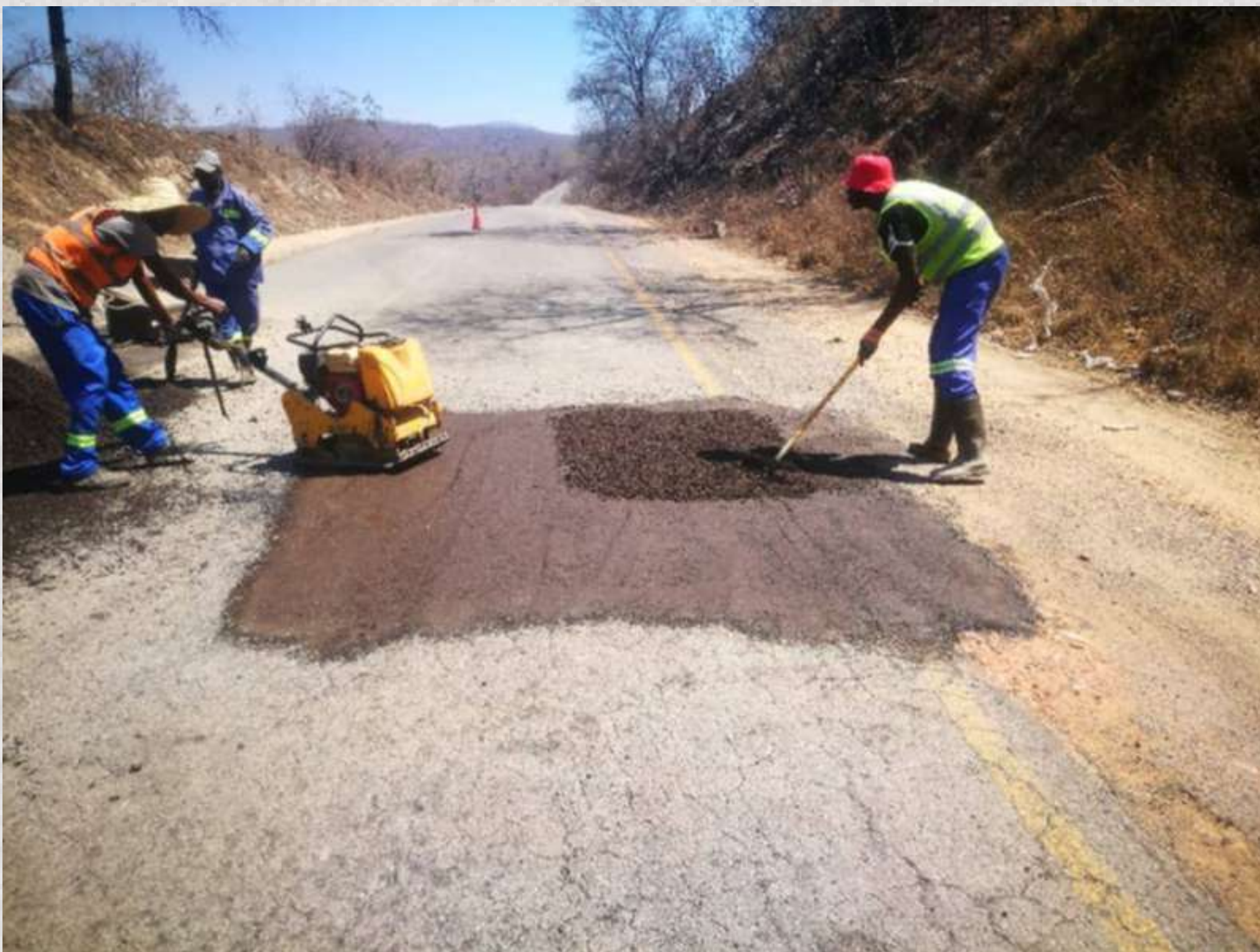
Compaction of the sealed pothole.
