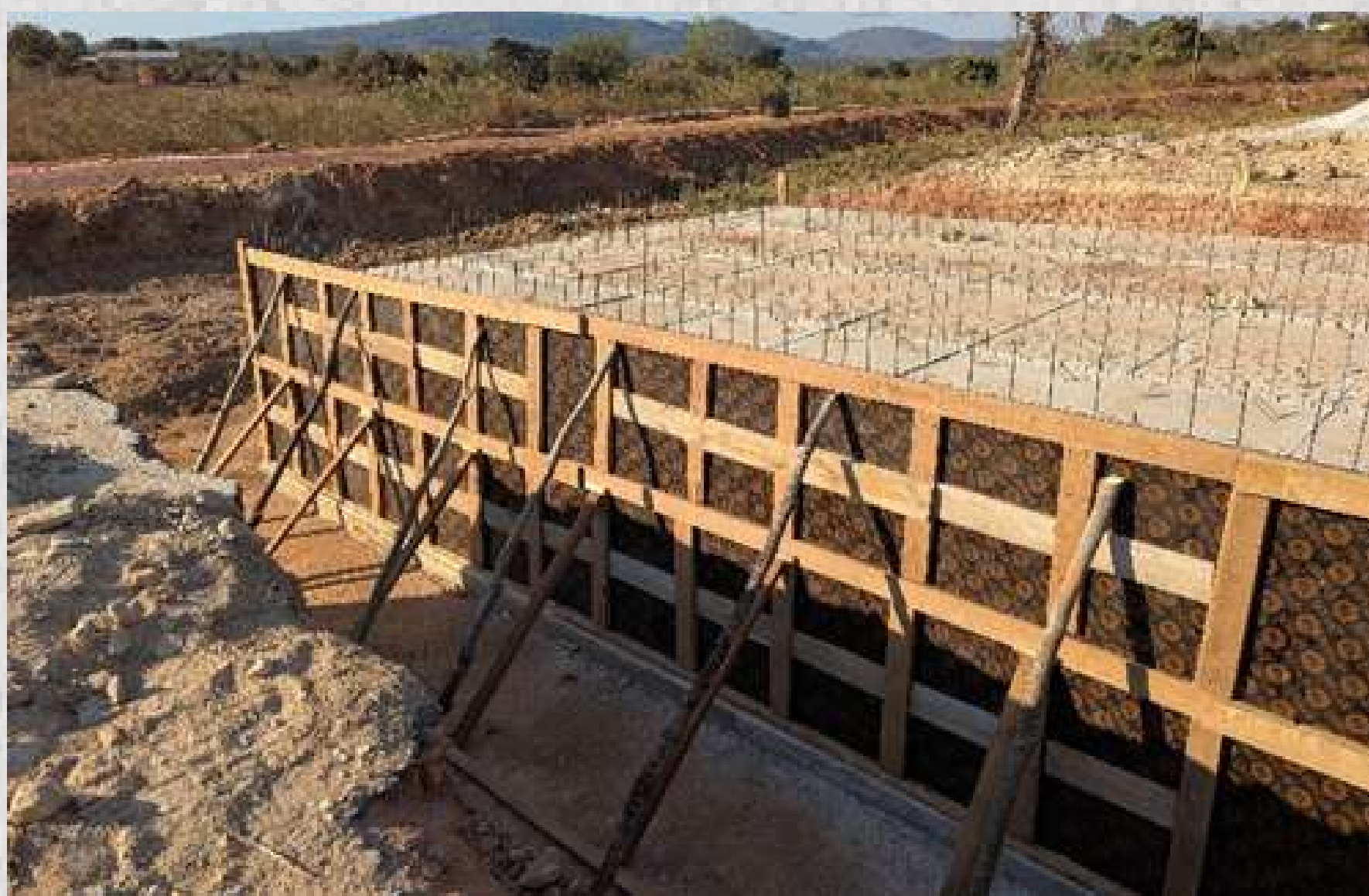
Kankumba Stream culvert works.
