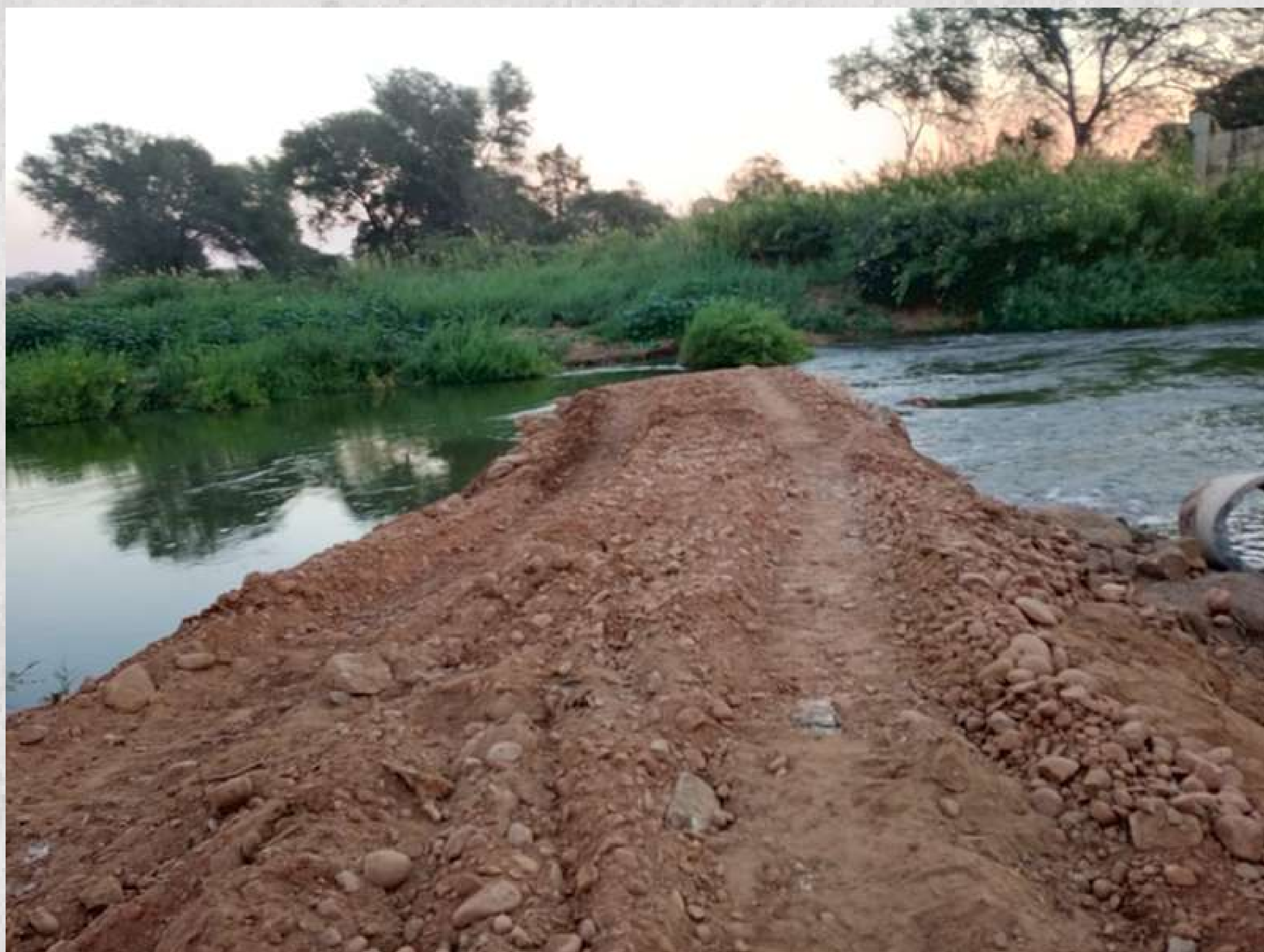
Progress of the temporary crossing with culvert installation ongoing.
