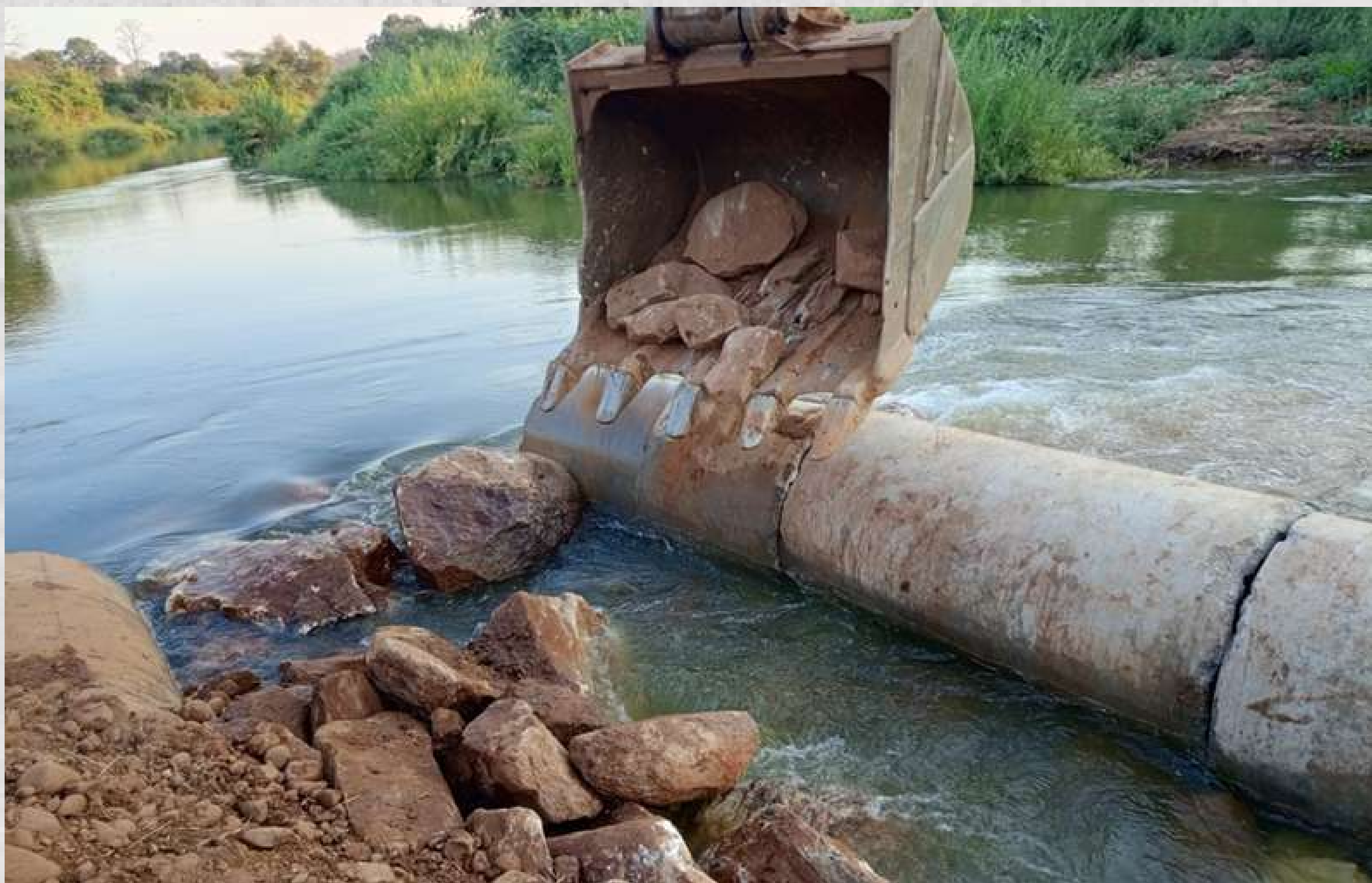
Installation of the fifth cell of the 900 mm culverts.
