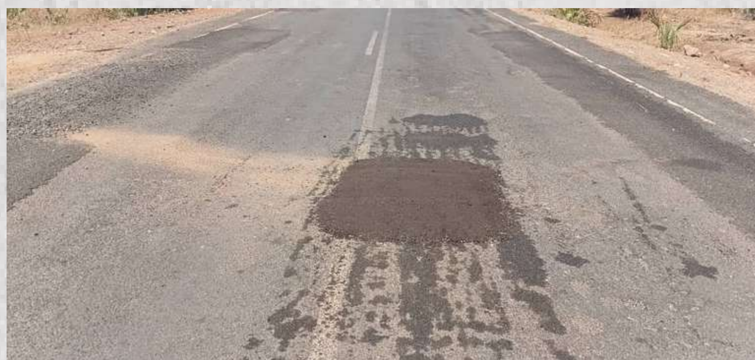
Stabilised and sealed pothole along Luangwa-Feira Road.
