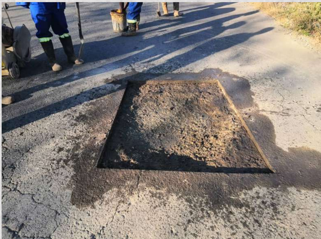
Shaped and cleaned Pothole.
