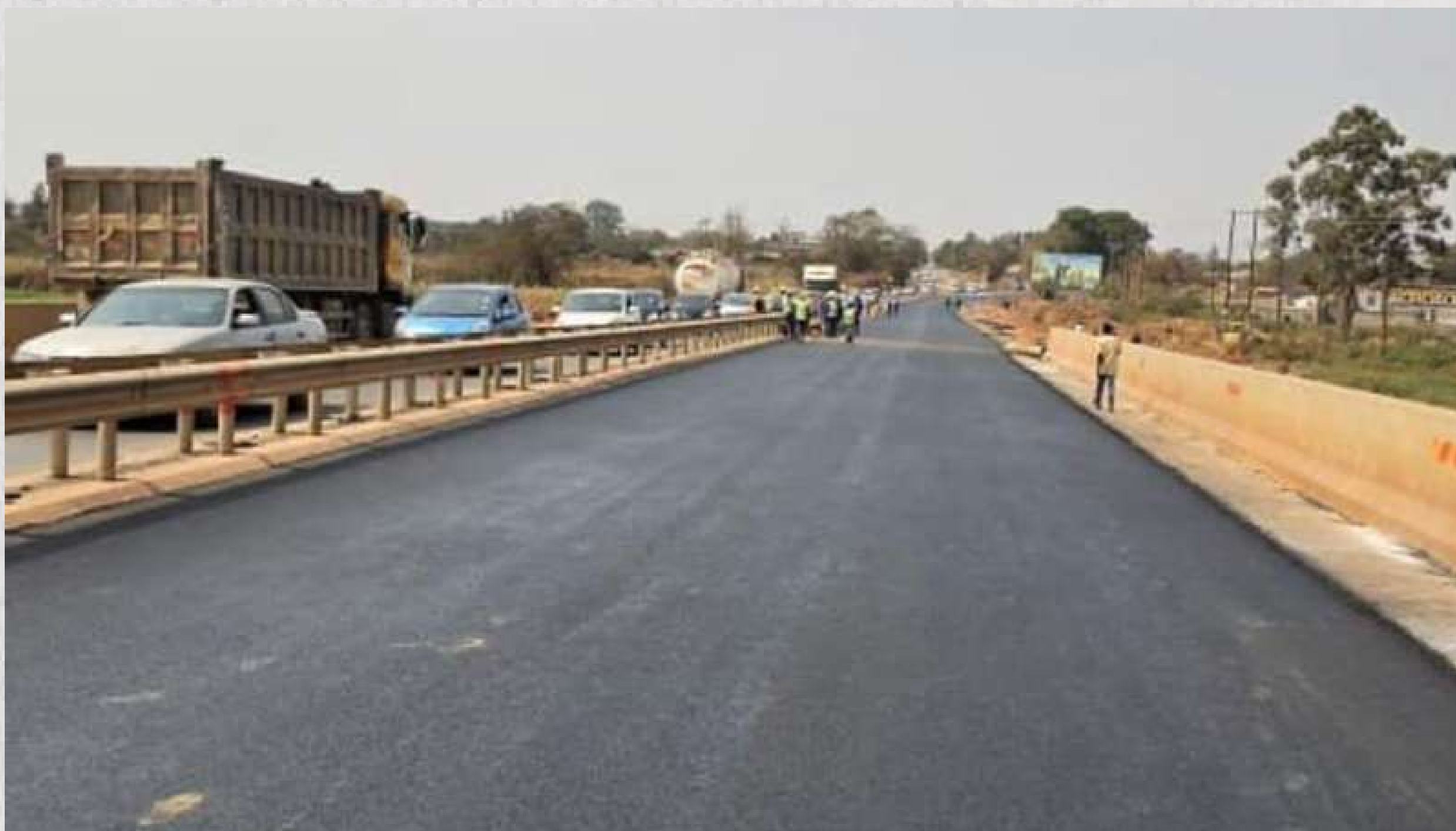
Asphalt pavement works at Kafubu Bridge.
