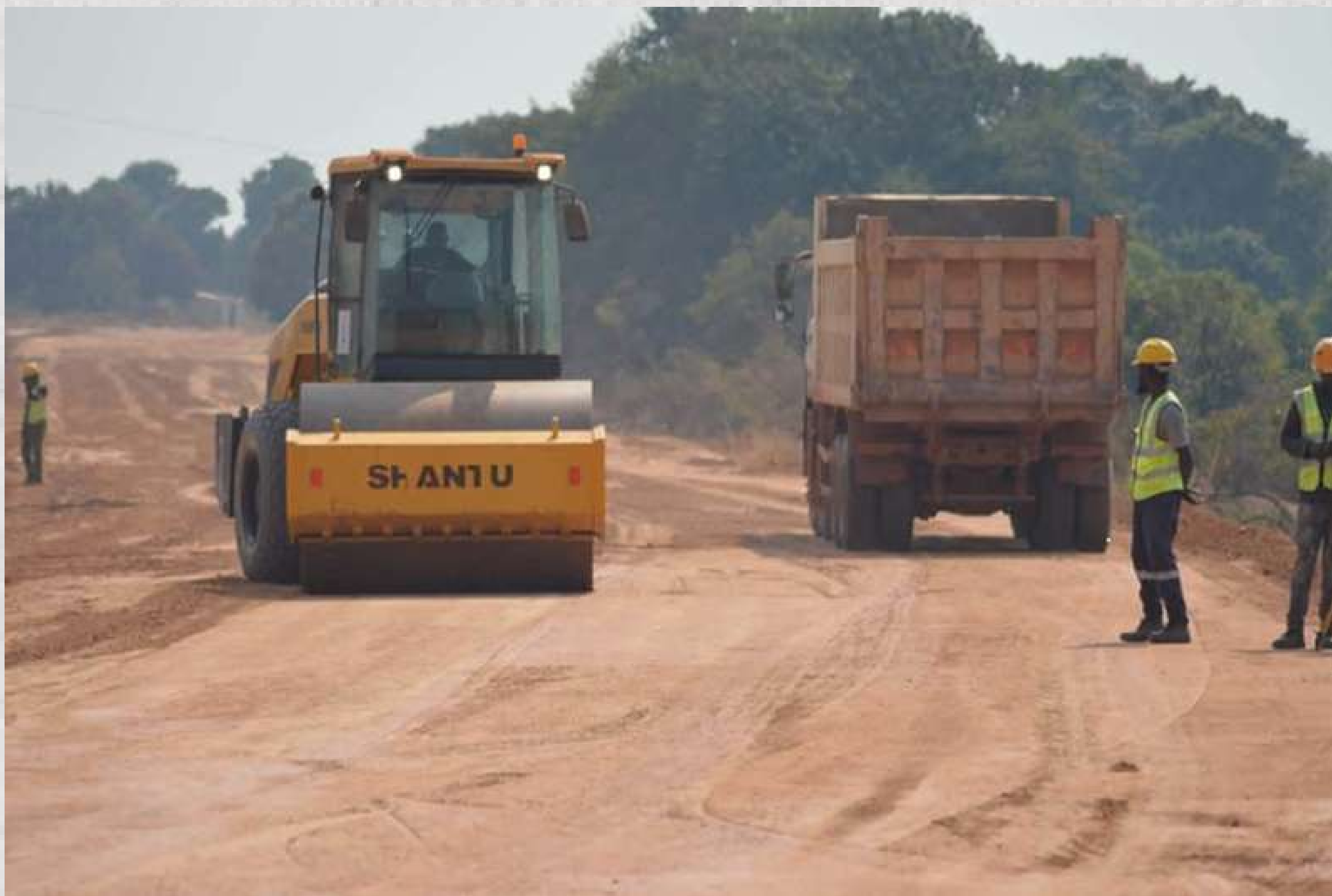
Ongoing works on the Samfya-Kasaba Road in Luapula Province.
