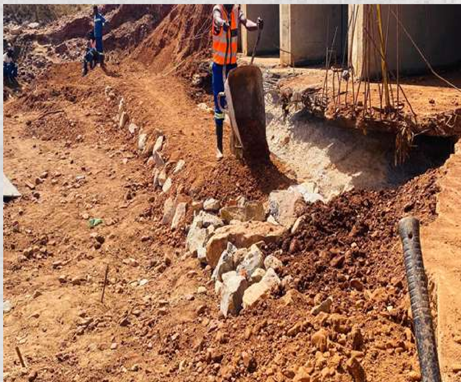
Placement of gravel over the stone layer.
