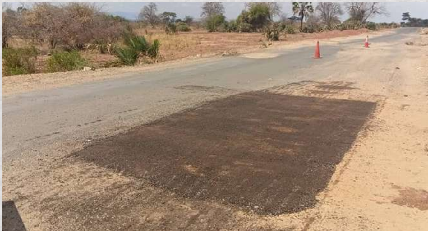
Stabilised and sealed potholes along Luangwa-Feira Road.
