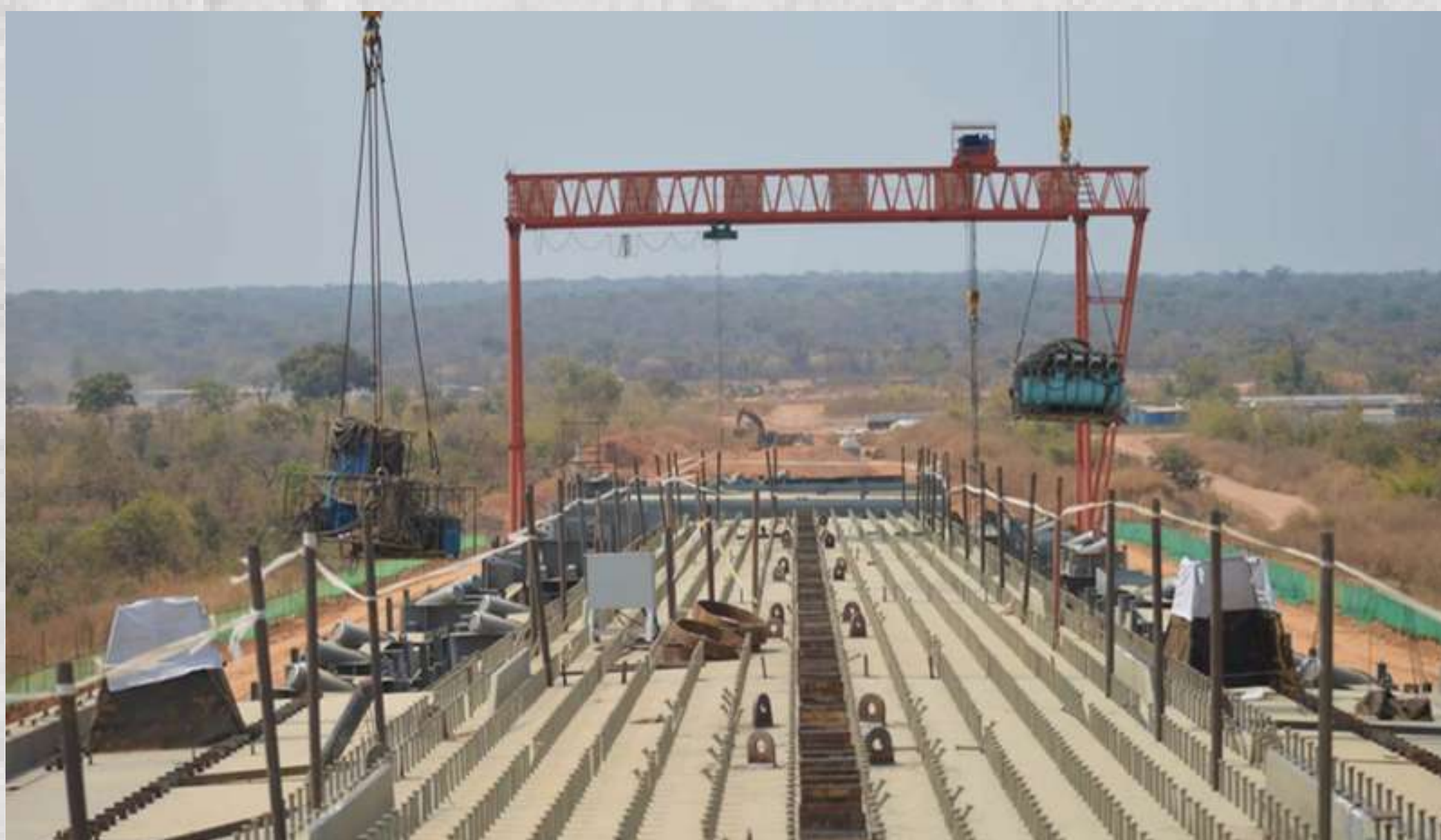
Works on the Kasomeno–Mwenda Road/Bridge Project.
