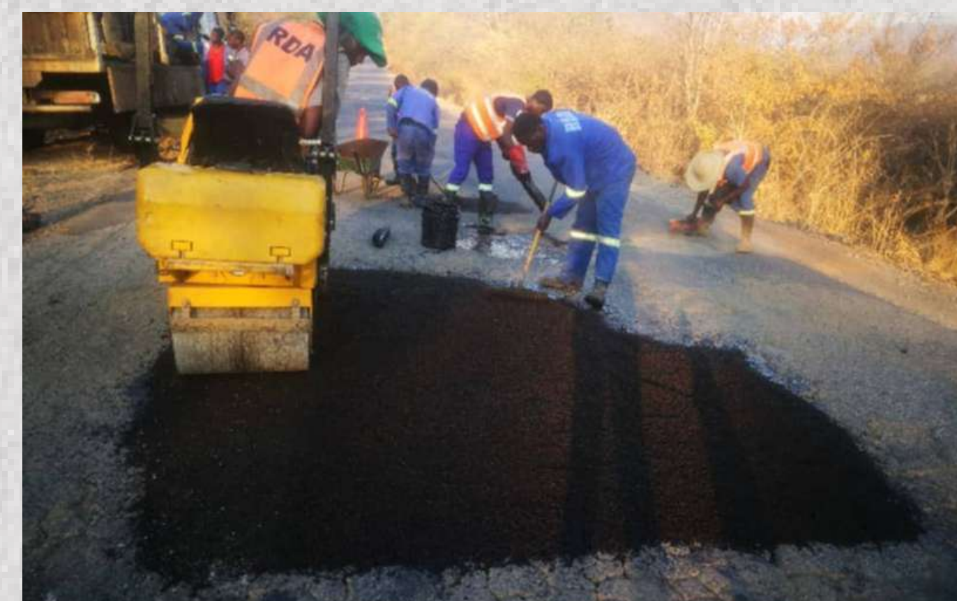
Sealed Potholes.
