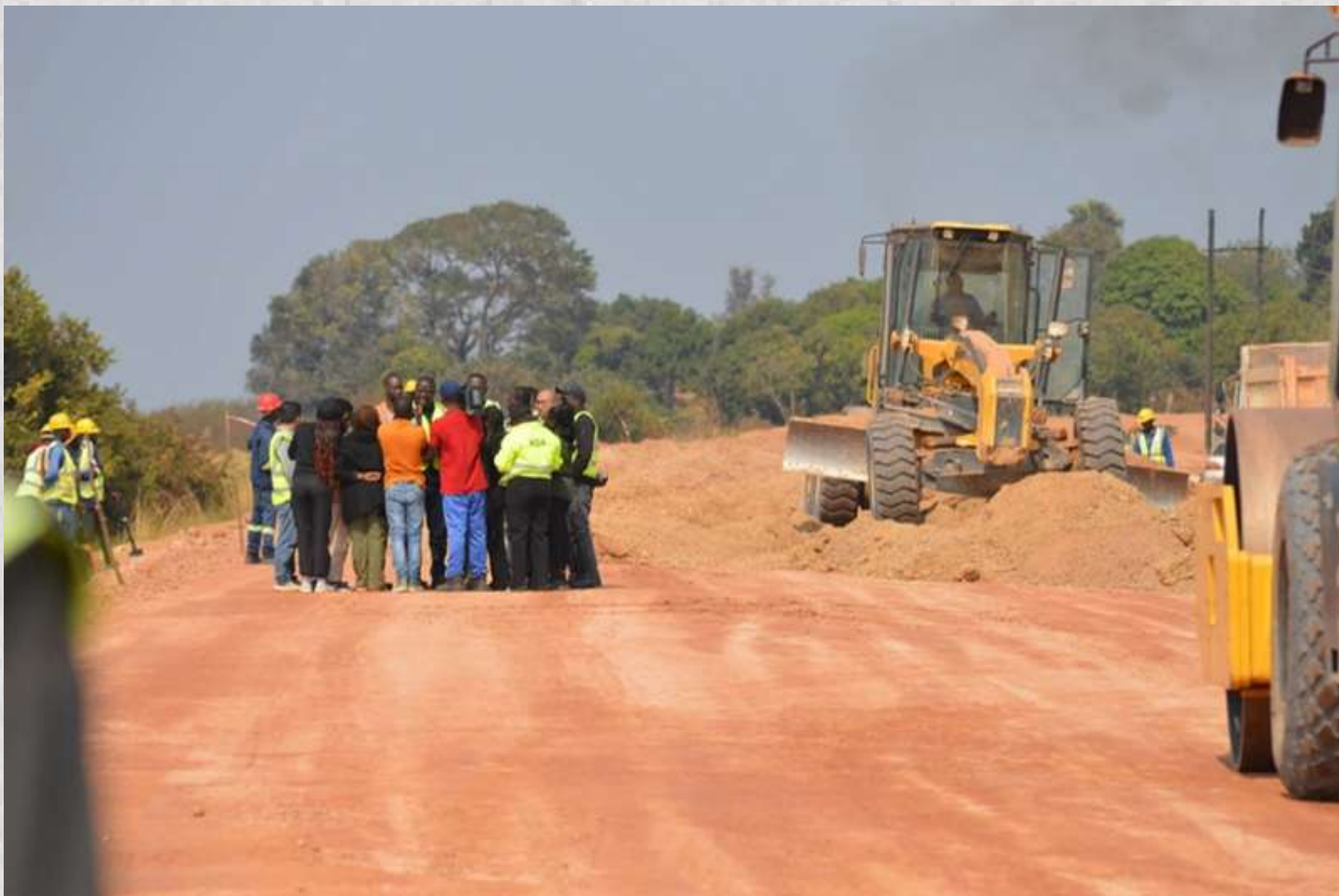
Media interview on site during the tour of the Samfya-Kasaba Road in Luapula Province.
