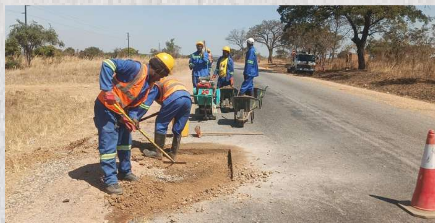
Cleaning off loose gravel of the shaped.
