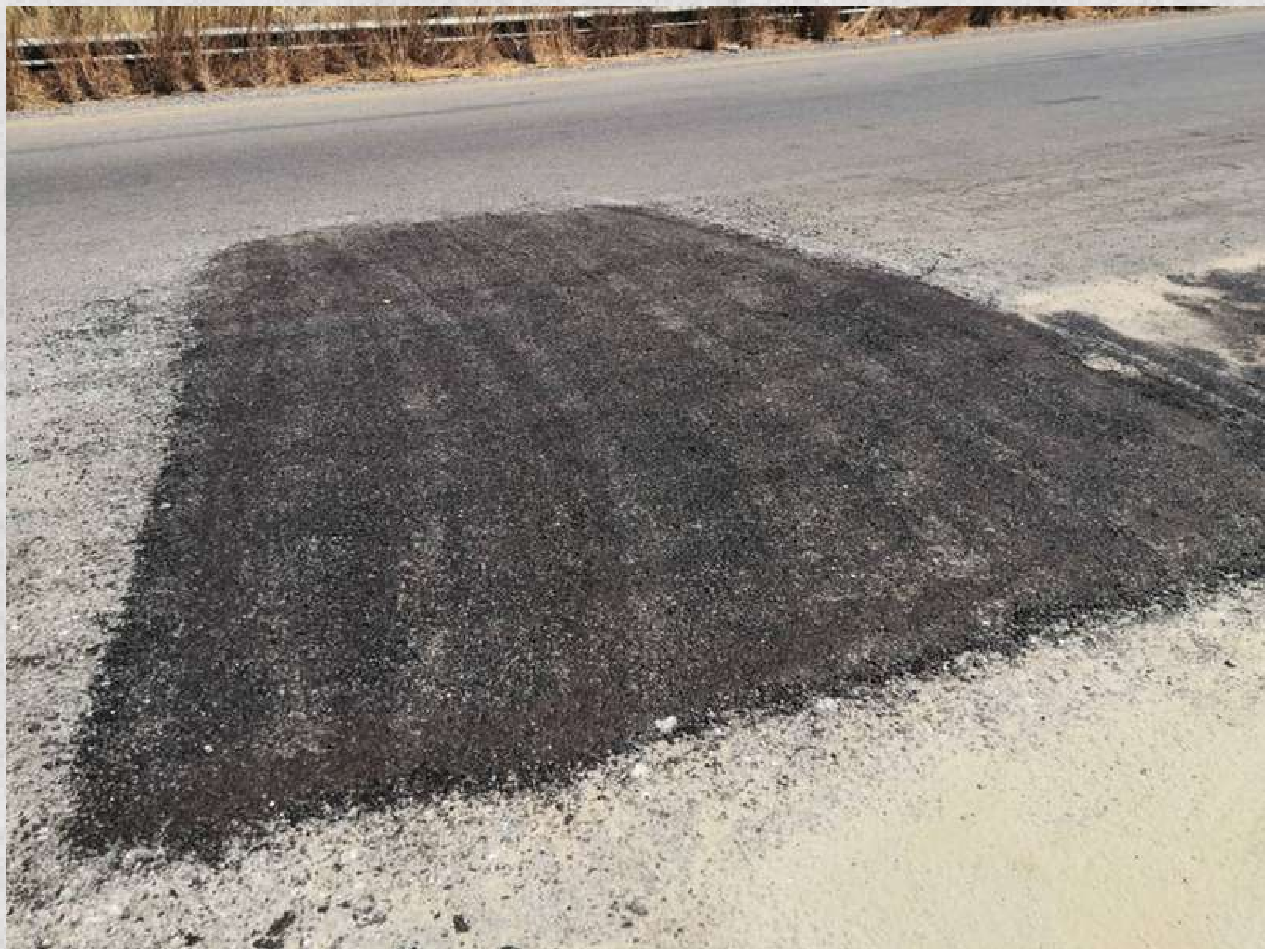
A sealed pothole.
