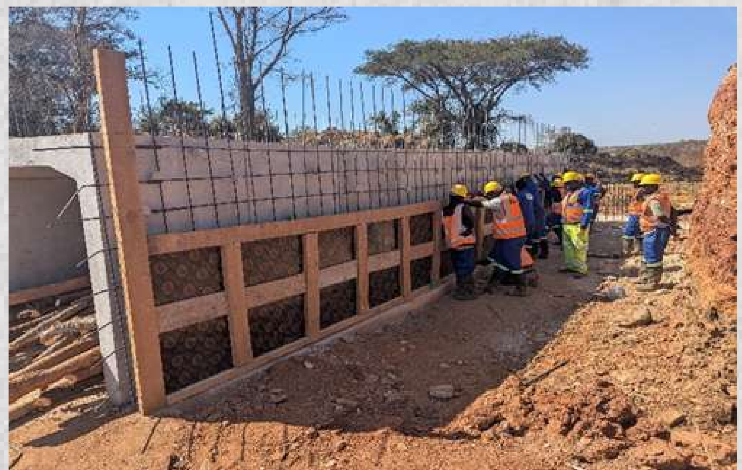
Form work preparations.
