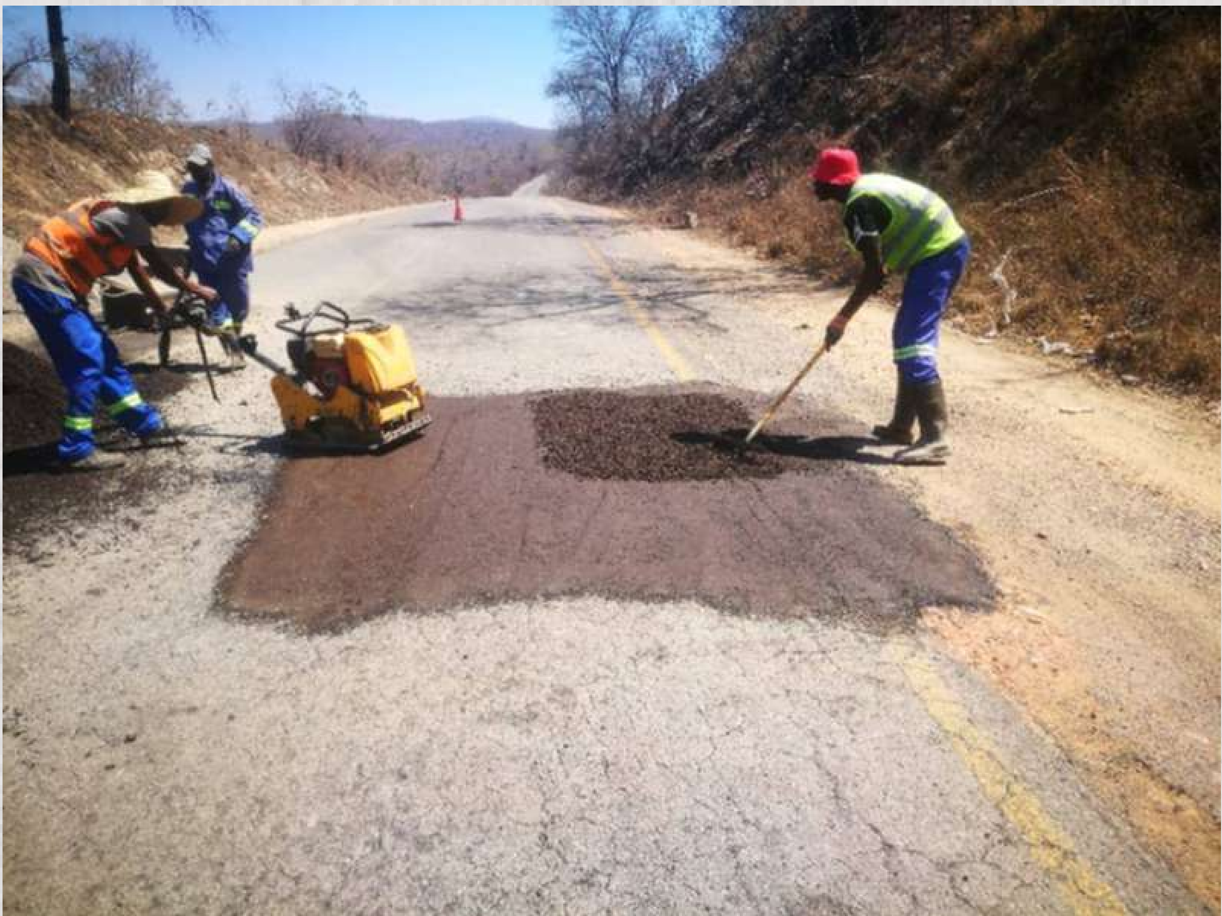
Compaction of the sealed pothole.
