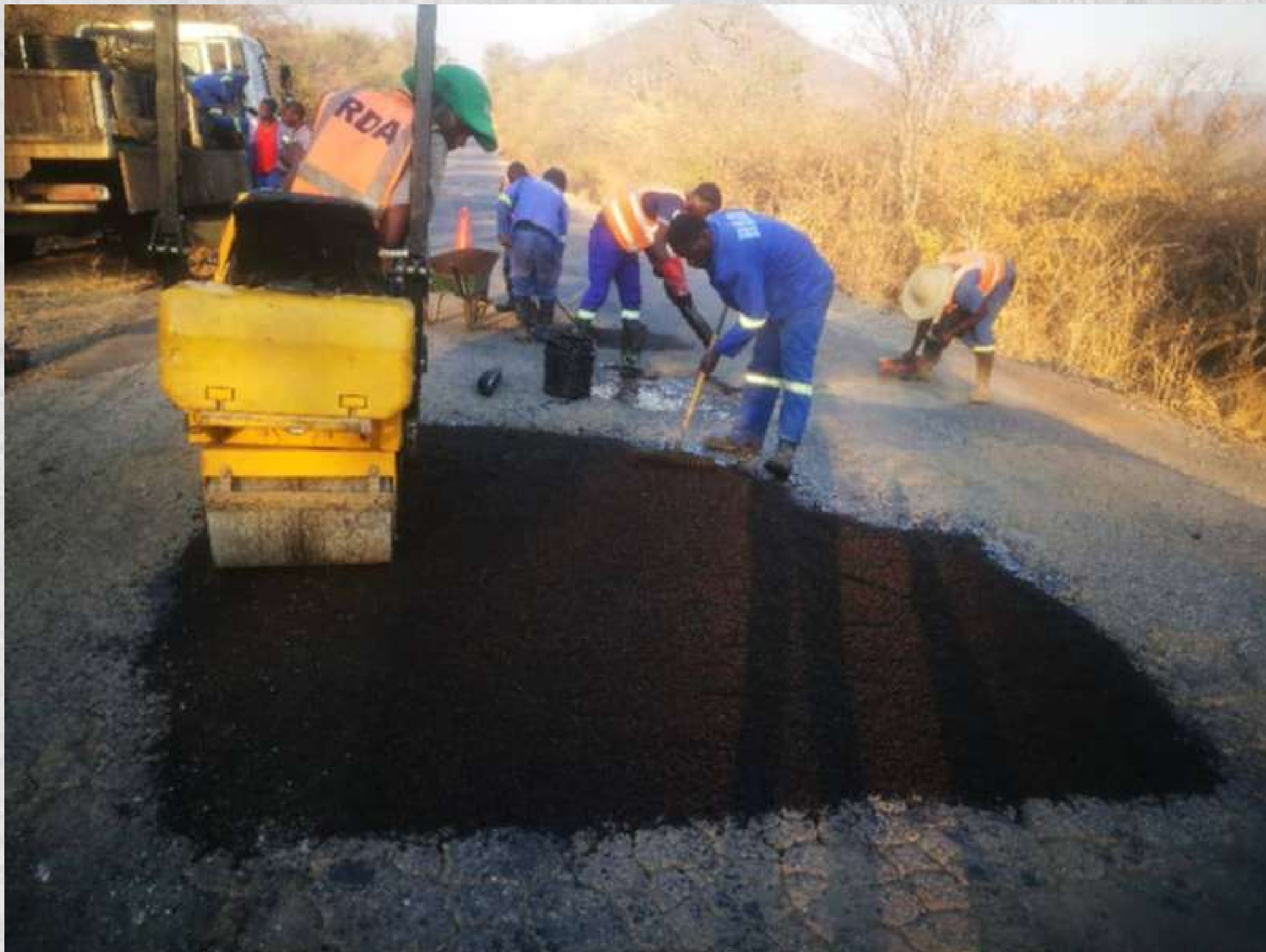
Sealed Potholes
