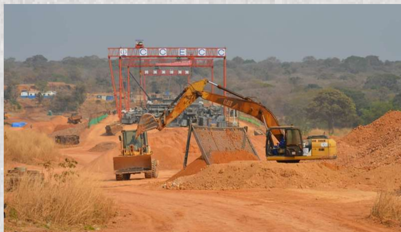
Works on the Kasomeno–Mwenda Road/Bridge Project.
