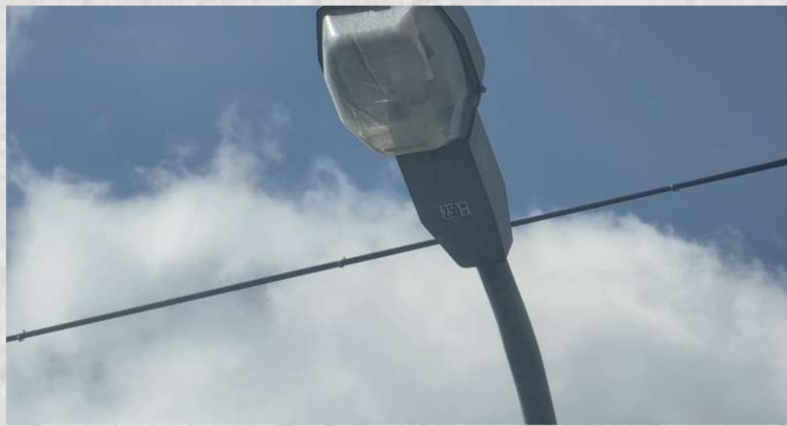
One of the streetlight at the bridge.
