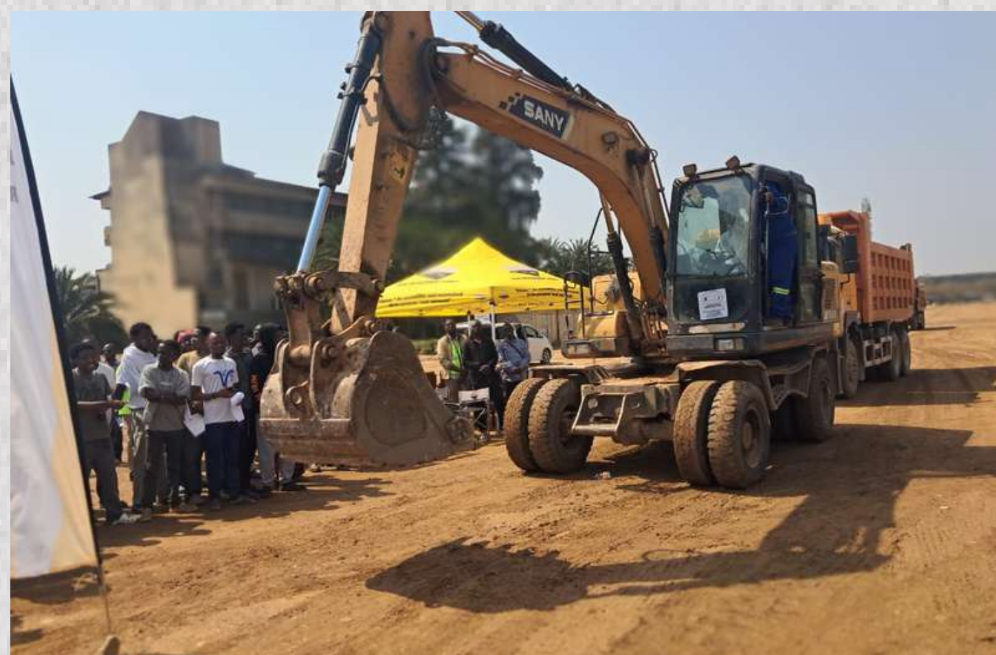
Symbolic groundbreaking of works at UNZA.
