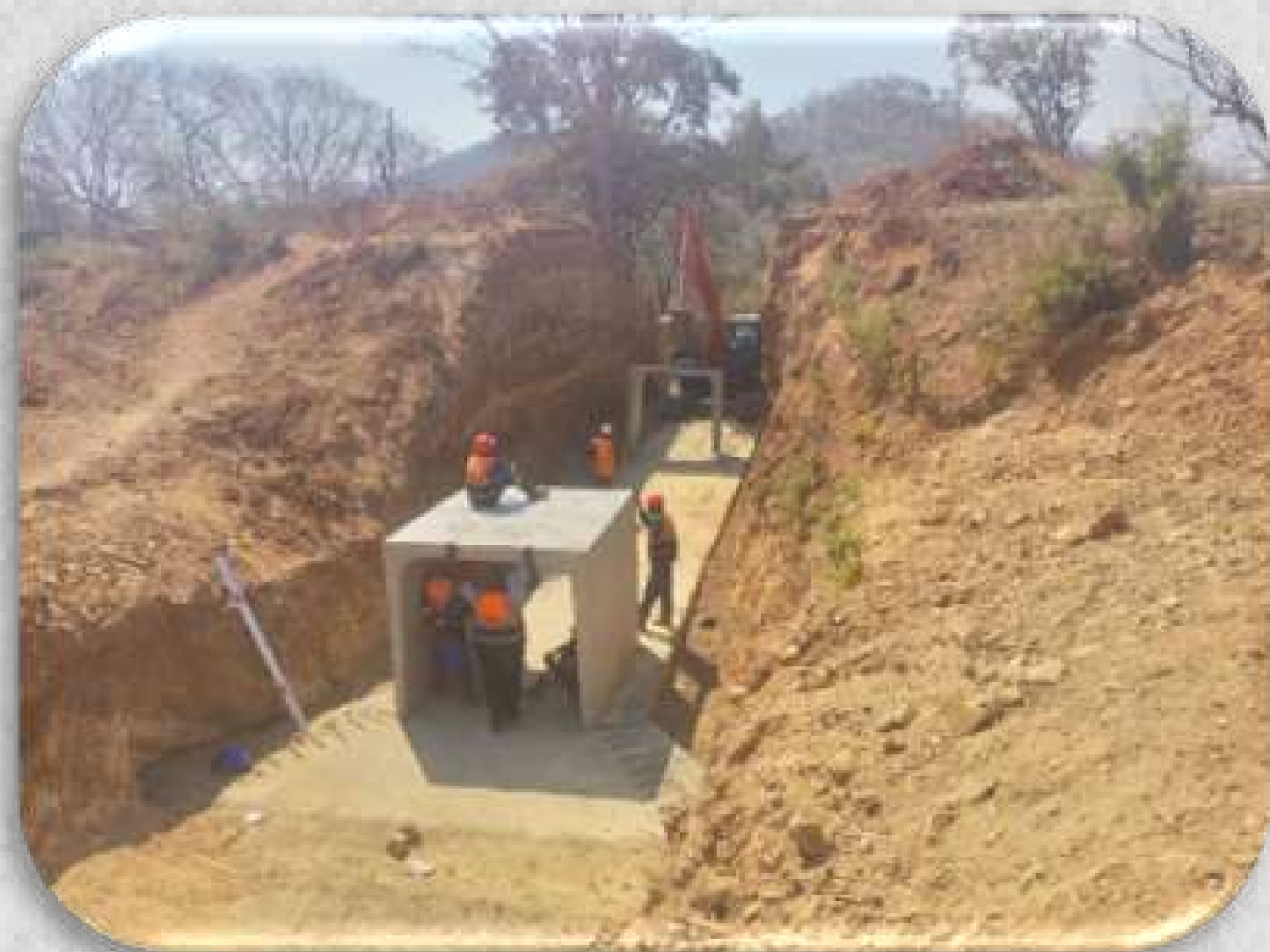
Installation of 1.8m x 1.8m Box Culverts.
