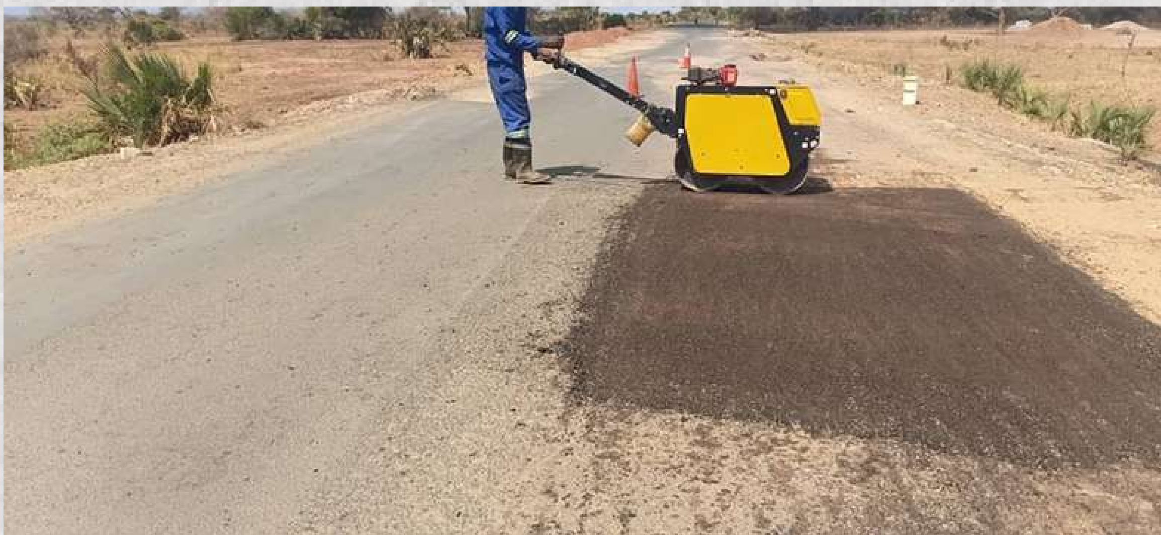
Compaction of stabilised pothole along Luangwa-Feira Road.
