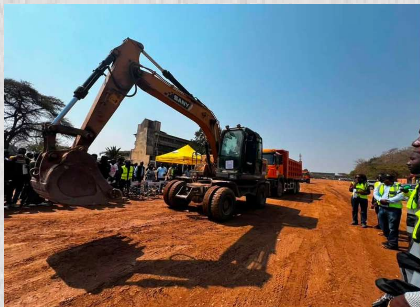
Symbolic groundbreaking of works at UNZA.
