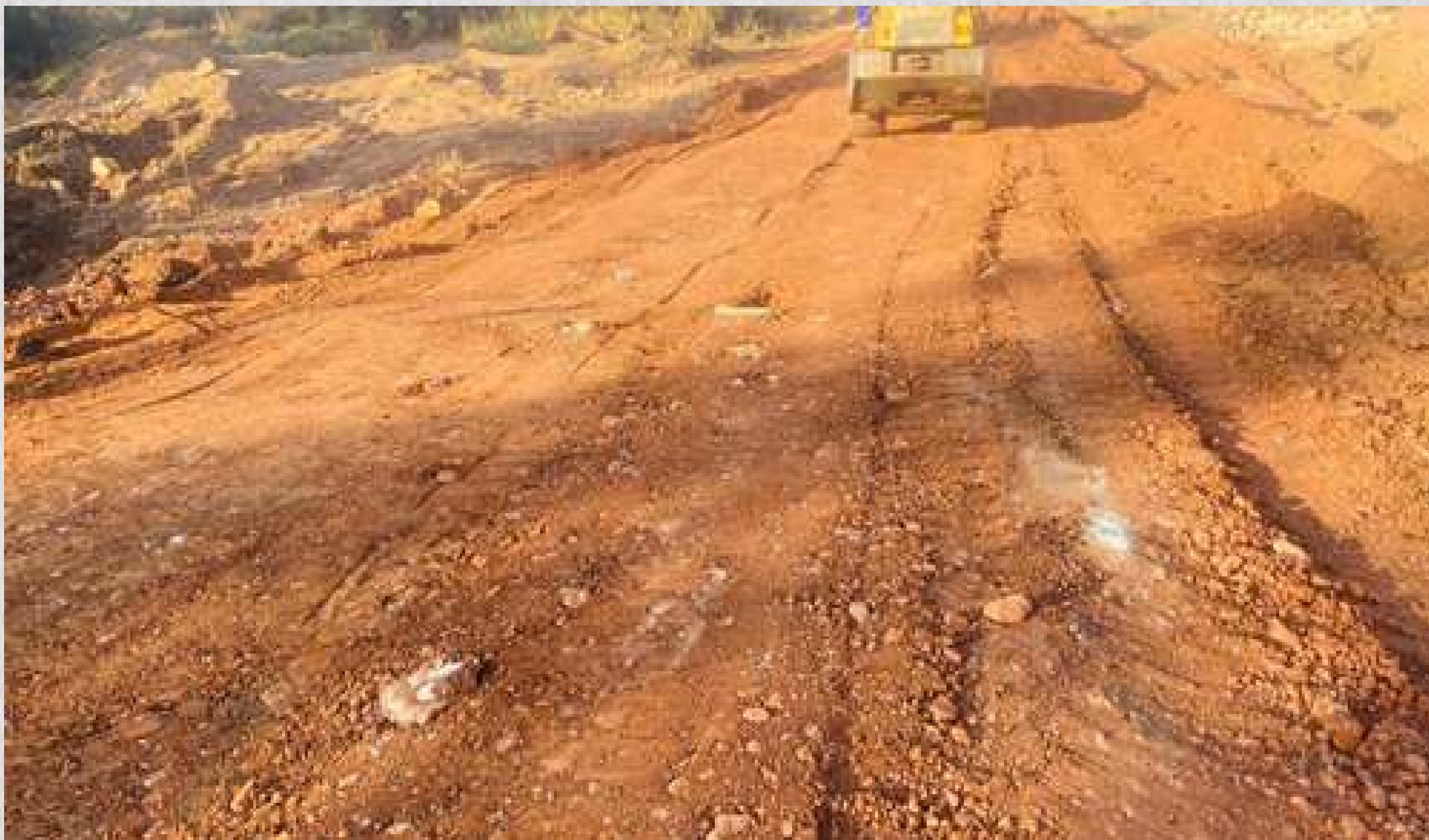
Compaction of gravel on the detour.
