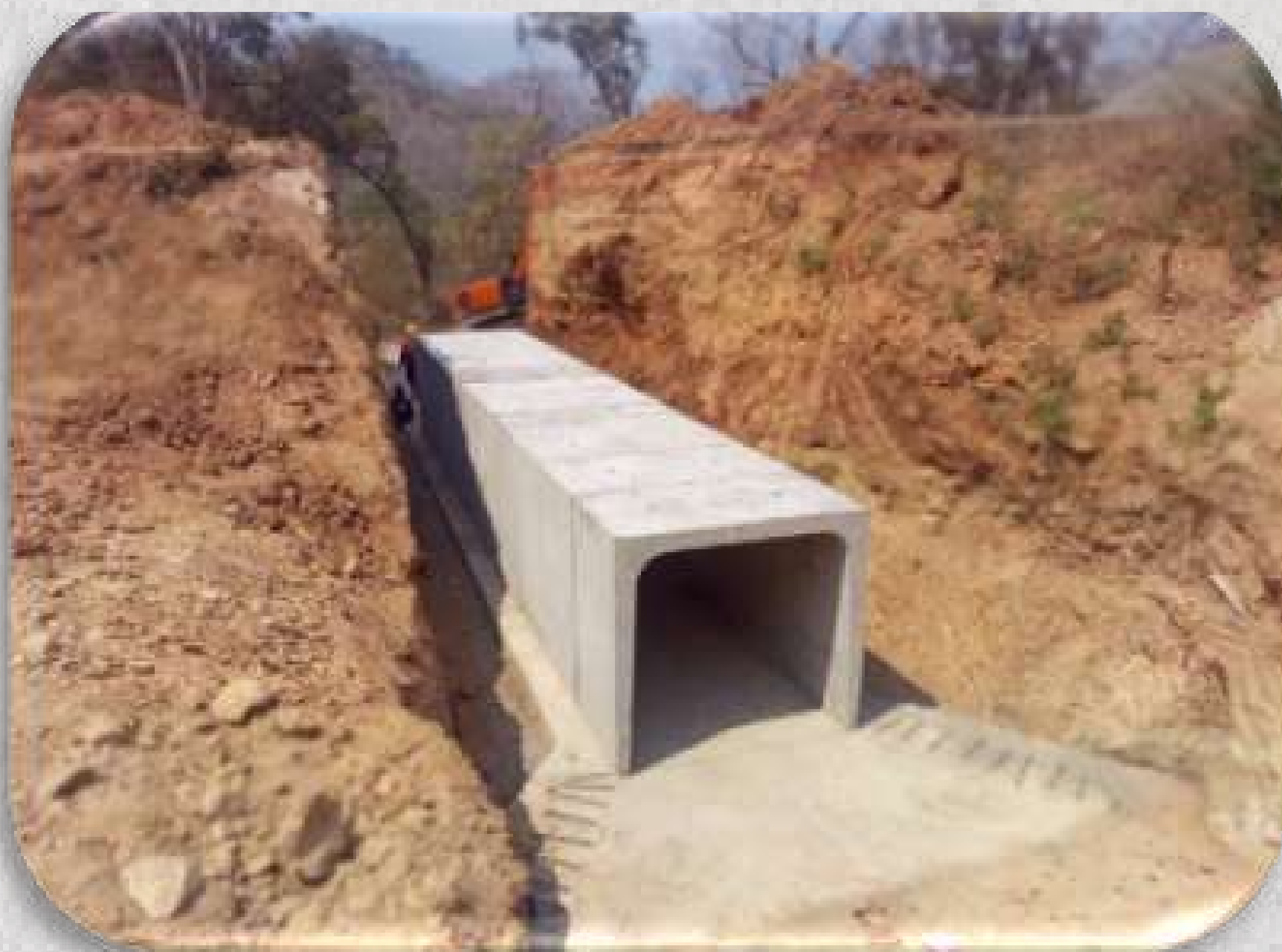
Installation of the 1.8m x 1.8m Box Culverts.
