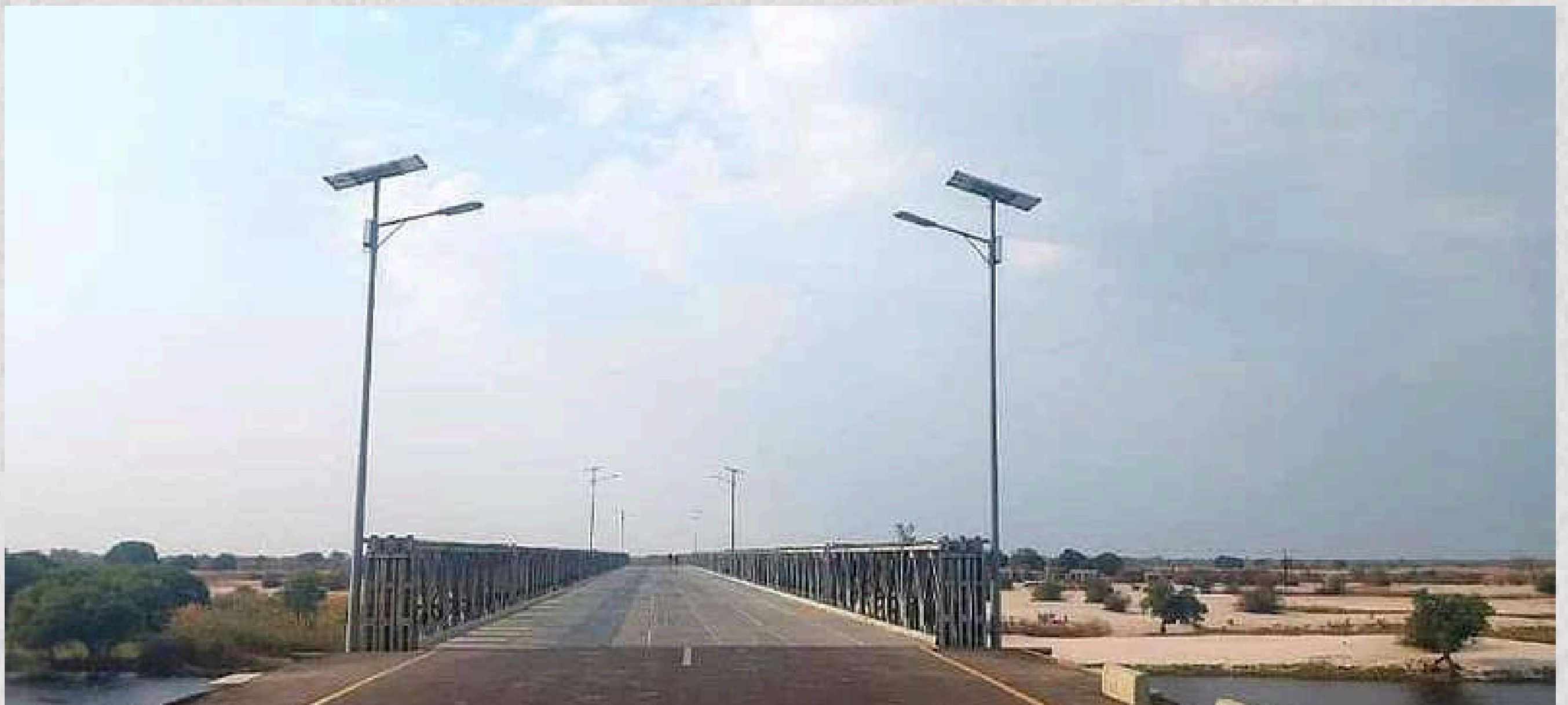
Silanda Bridge in Kalabo District, Western Province.
