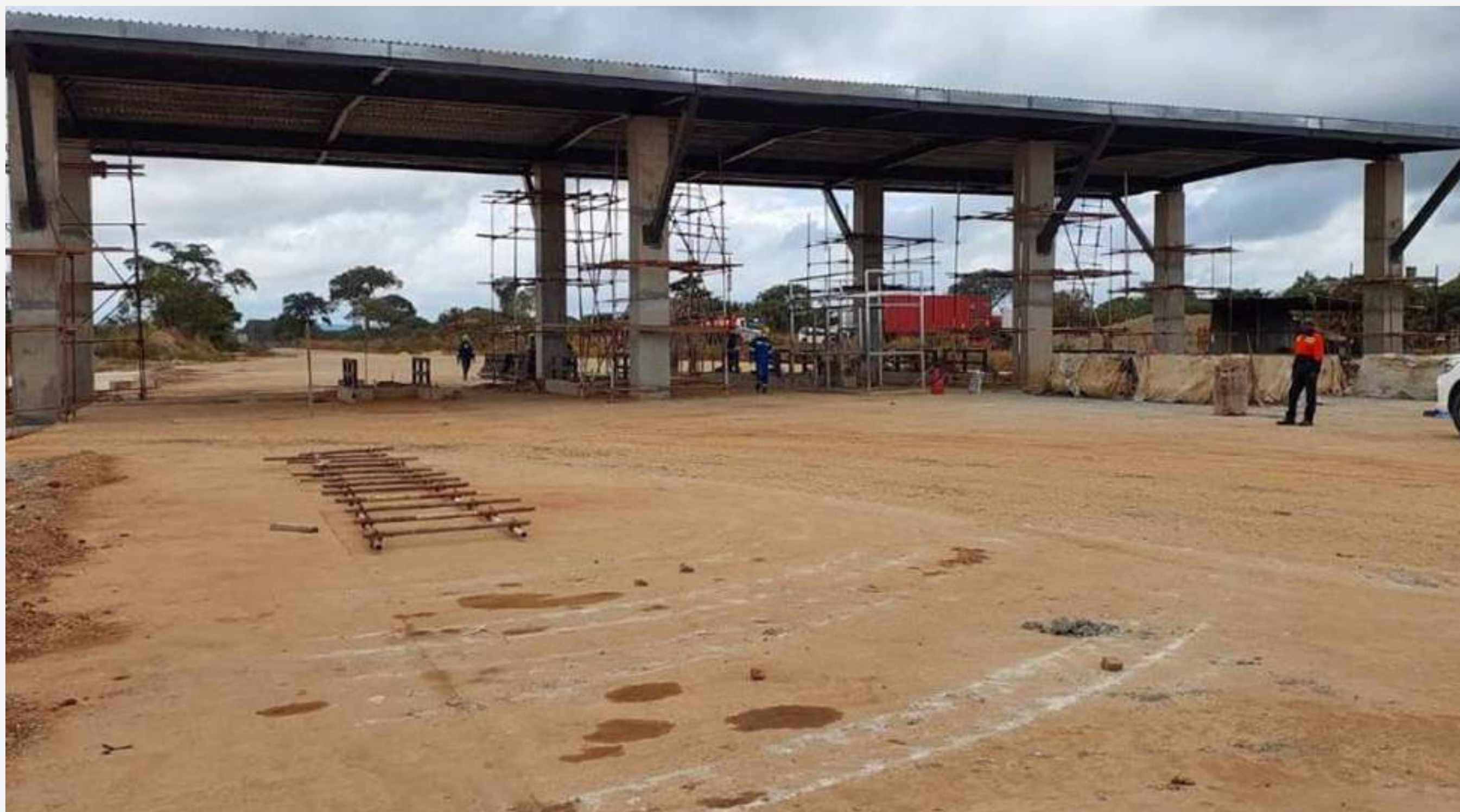
Chinsali Toll Plaza under construction.
