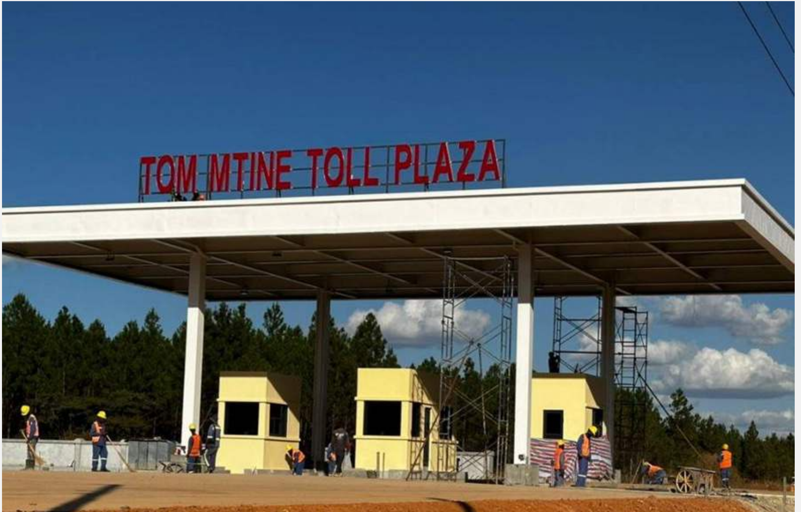
Ongoing construction works of a Toll Plaza along Ndola-Sakania-Mufulira Road.
