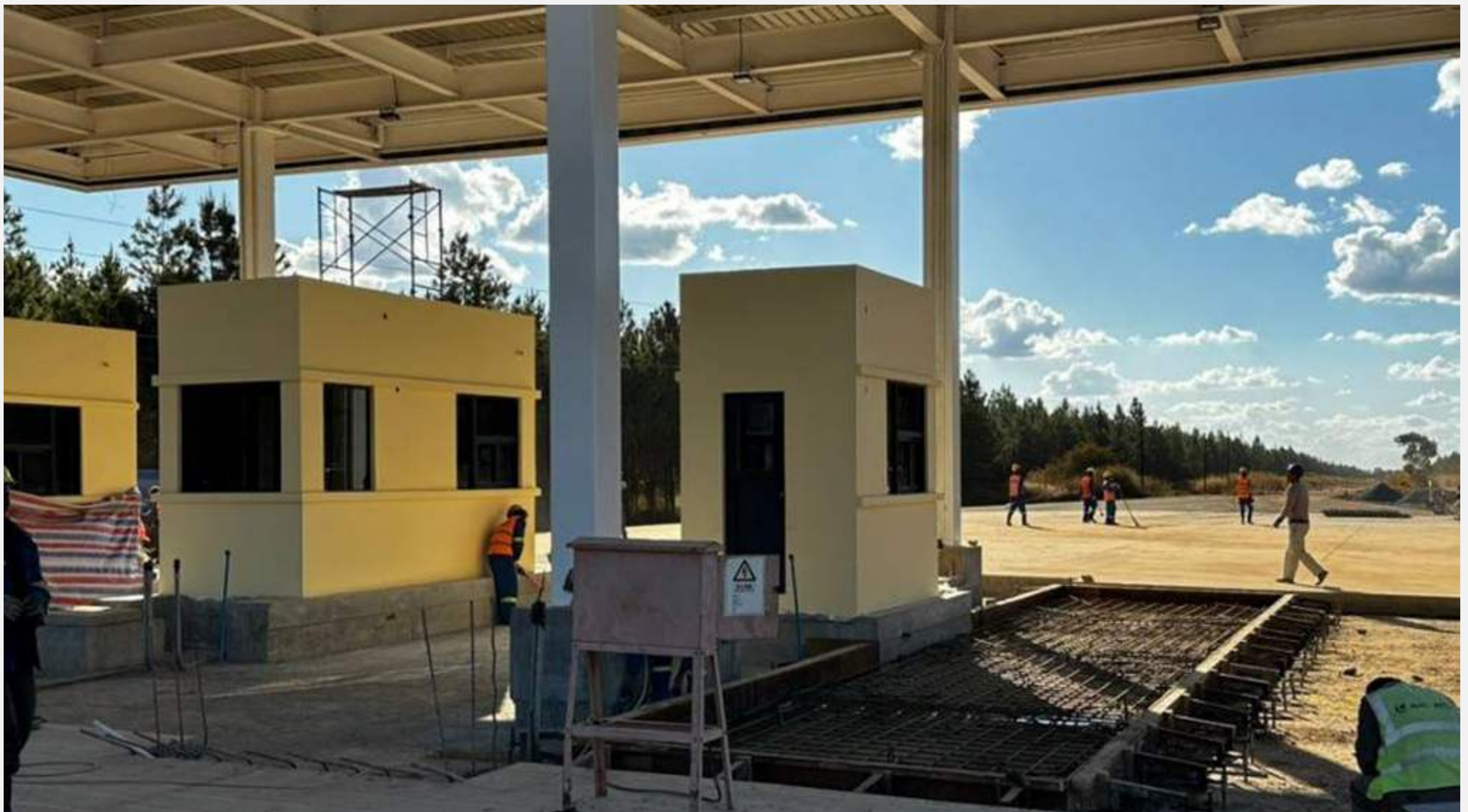
Ongoing construction works of a Toll Plaza along Ndola-Sakania-Mufulira Road.
