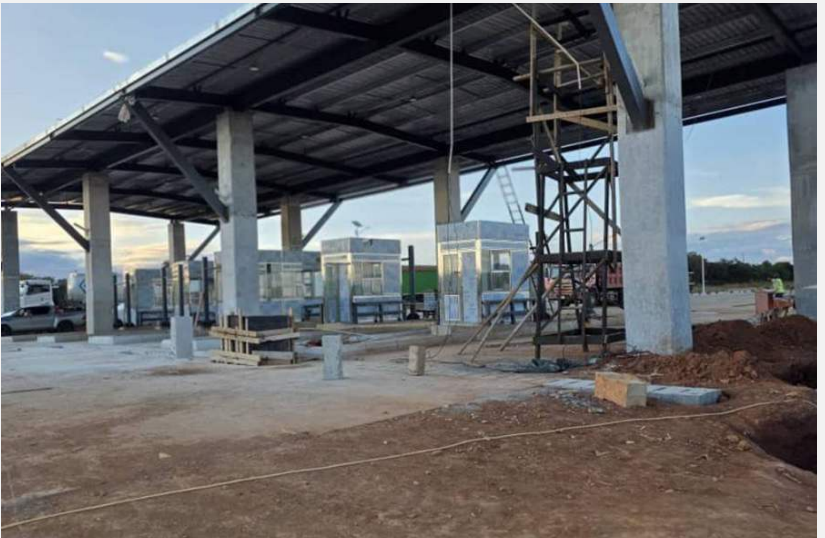
Chinsali Toll Plaza booths under construction.
