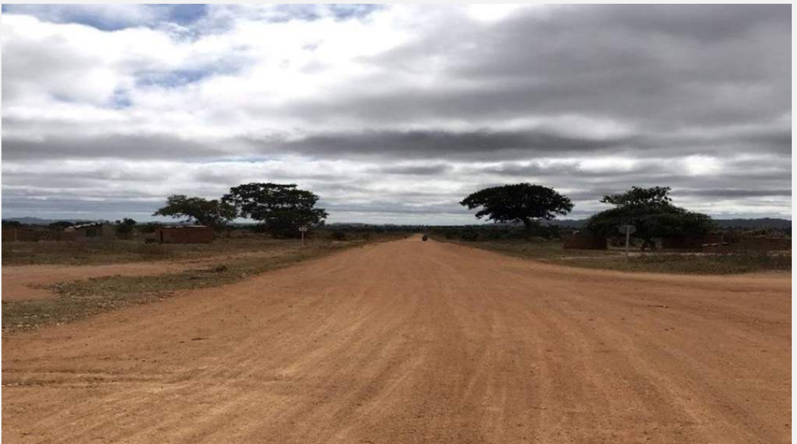
One of the rehabilitated roads under IRCP in Eastern Province.
