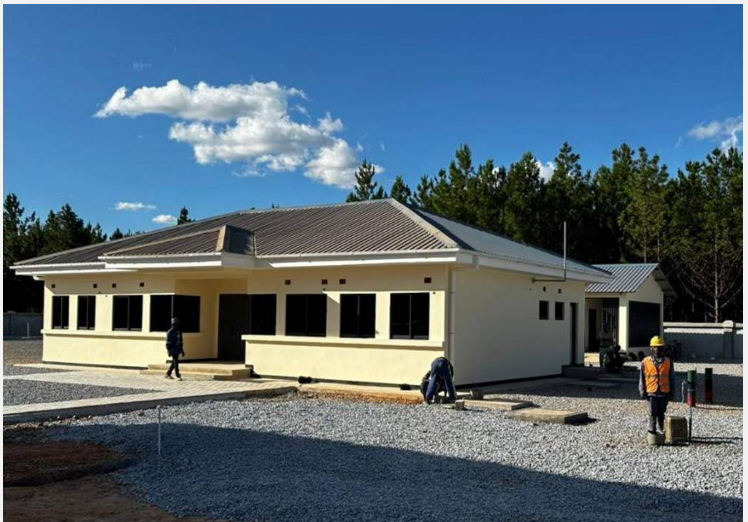
Ongoing construction works of the Toll Plaza office along Ndola-Sakania-Mufulira Road.
