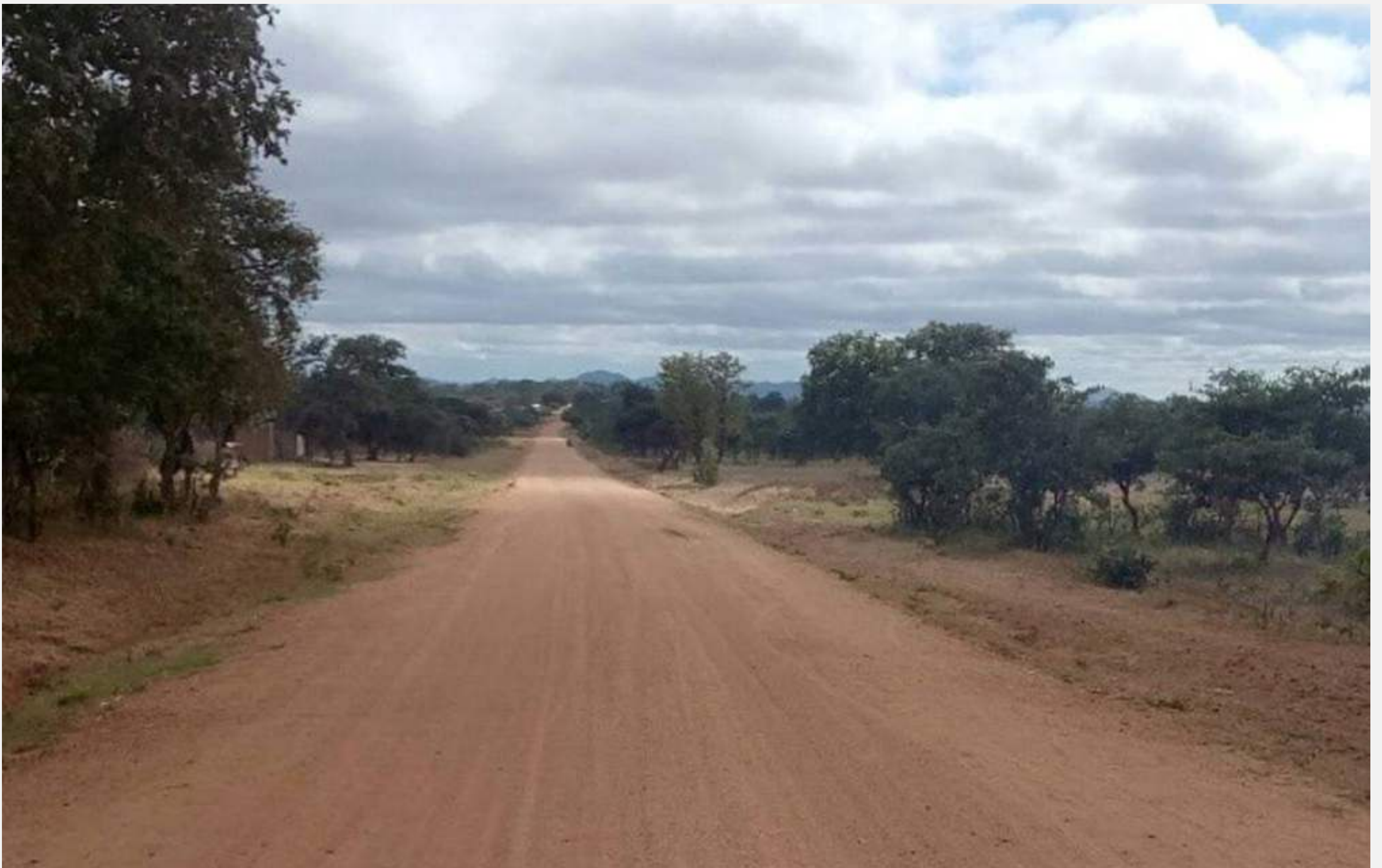
One of the rehabilitated roads under IRCP in Eastern Province.
