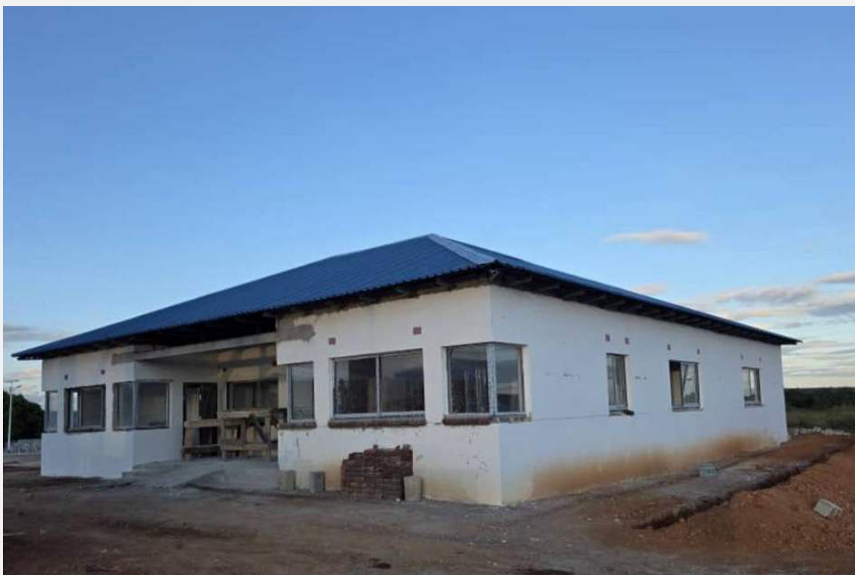
Chinsali Toll Plaza Office under construction.
