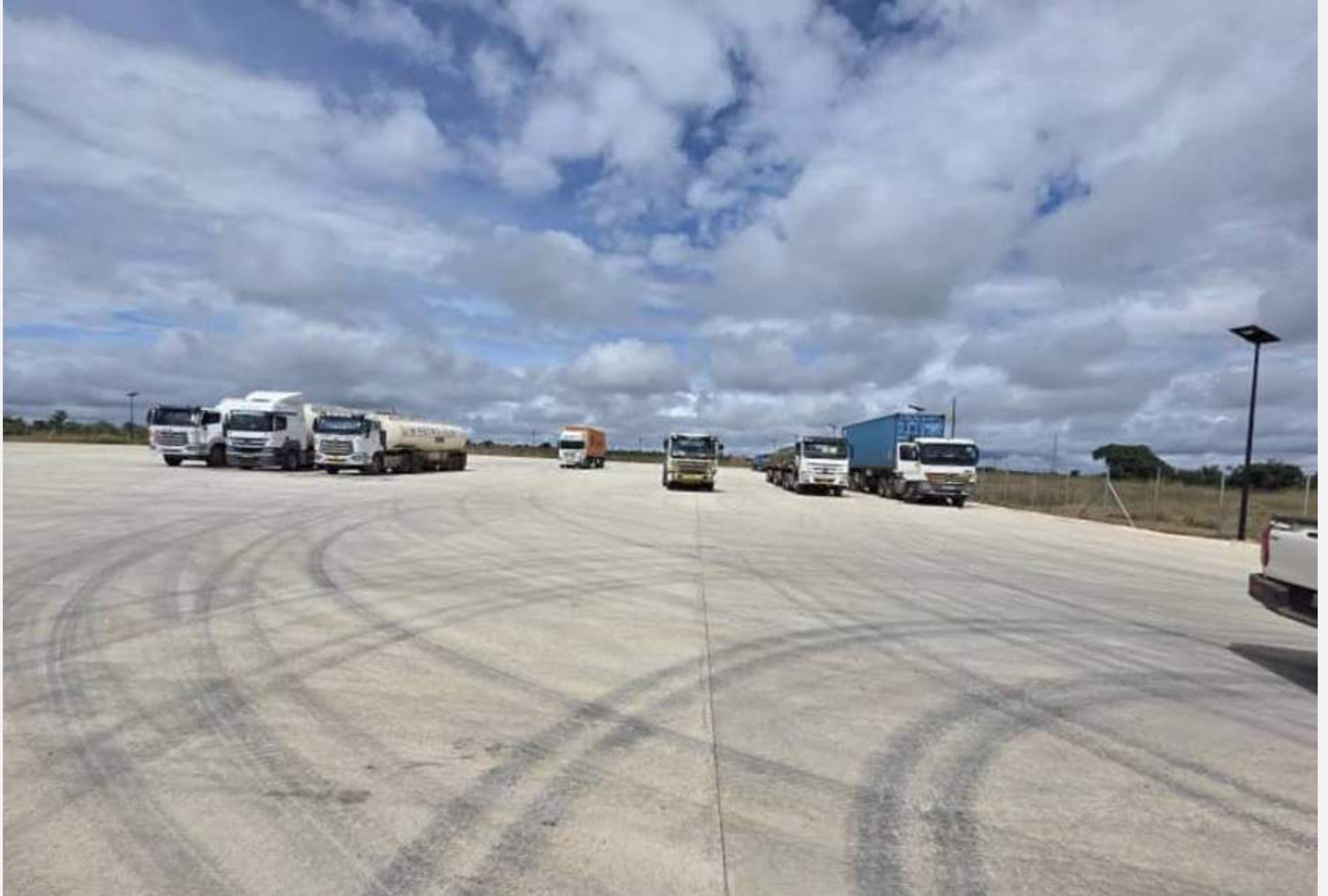
A newly constructed truck park.
