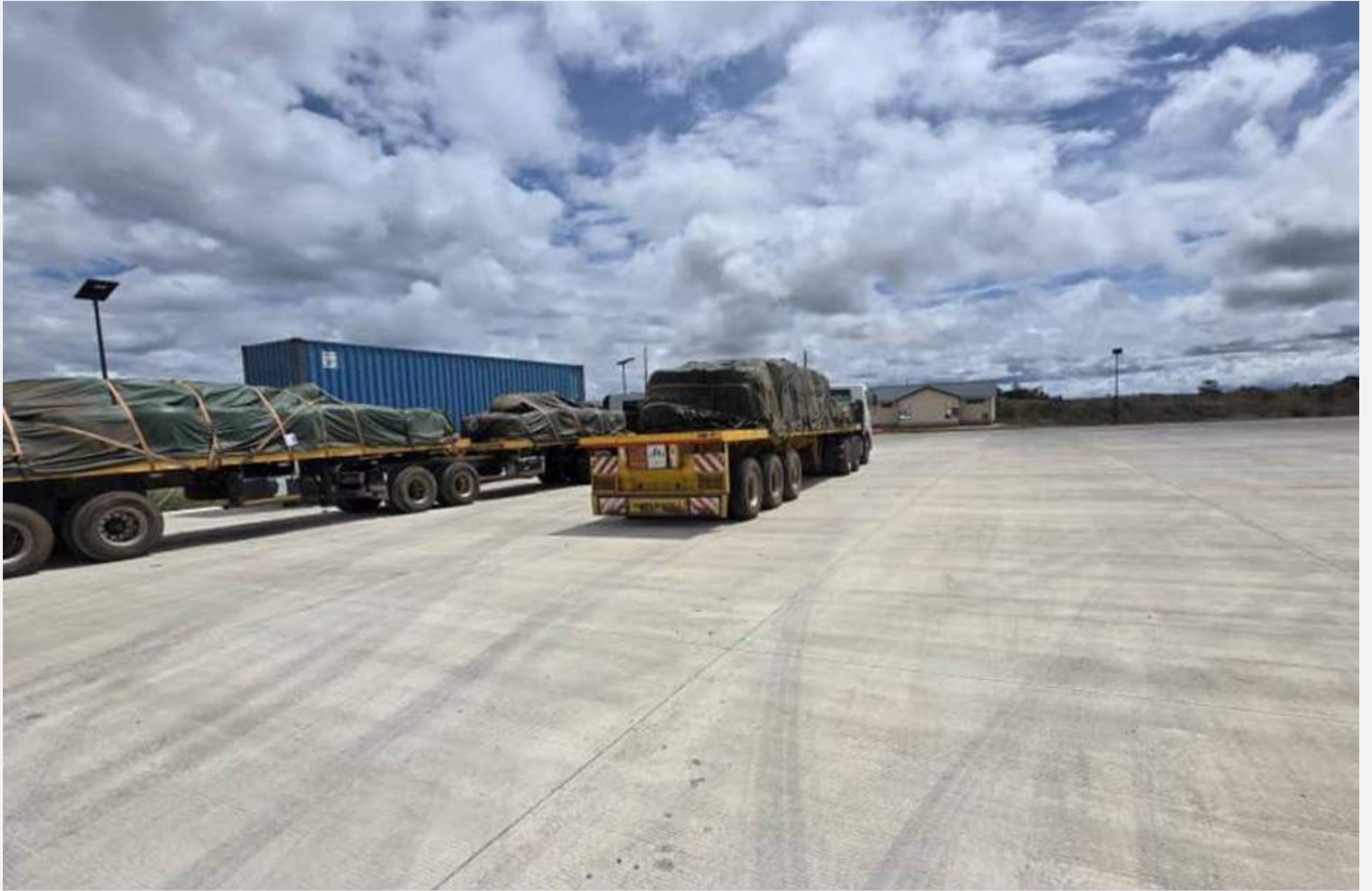
Newly constructed truck park
