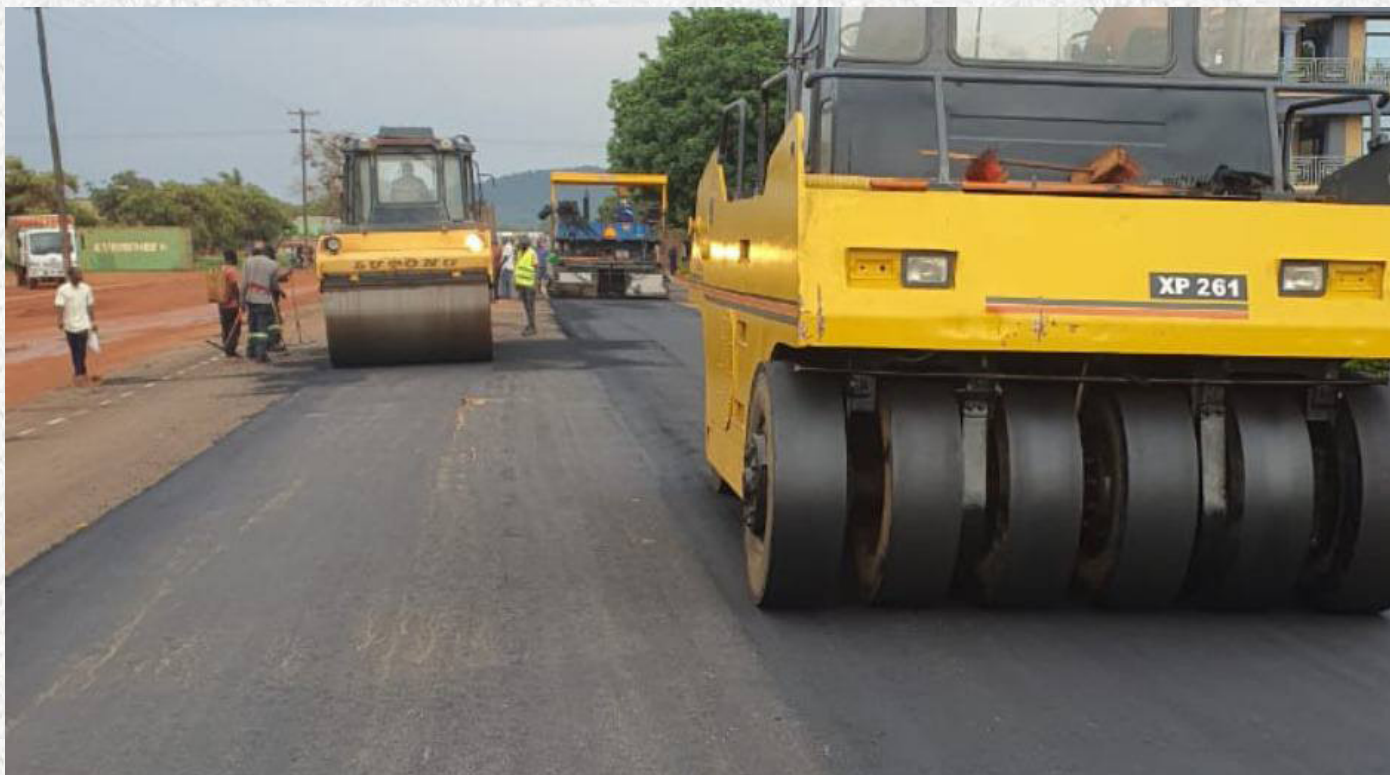
Rehabilitation works on Katete-Chanida Road in Eastern Province.
