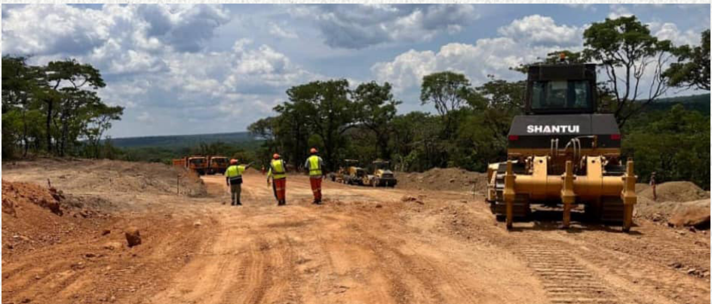
Lumwana-Kambimba Road works have commenced in North Western Province.
