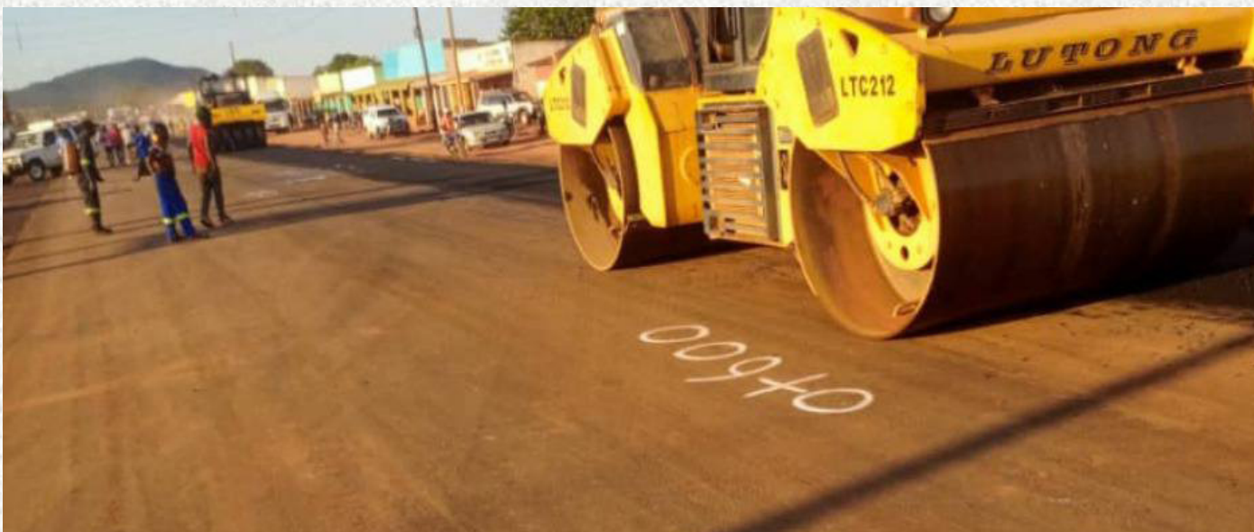
Ongoing works on the Katete-Chanida Road.
