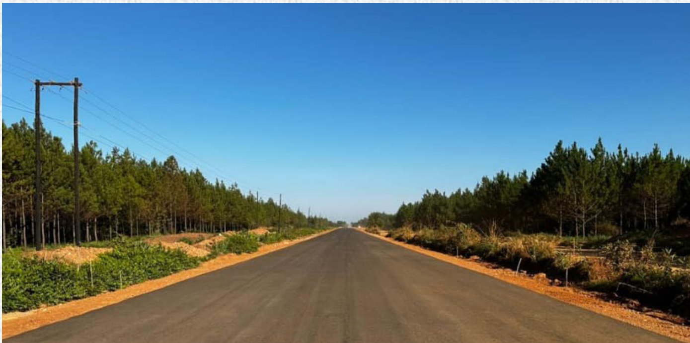
Ndola-Sakania-Mufulira Road works.
