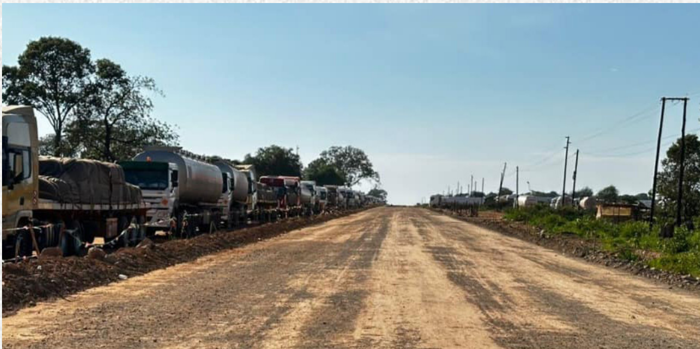
Civil works on the Ndola-Mufulira Road.
