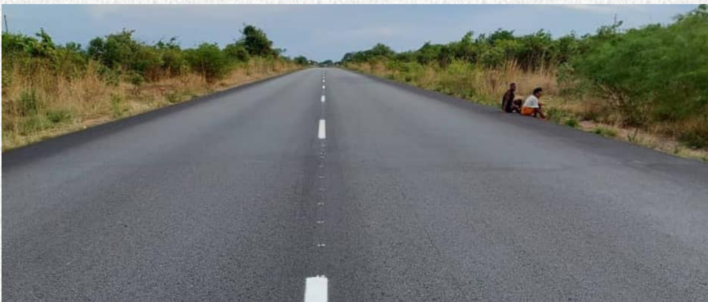
The newly rehabilitated Chinsali-Nakonde Road.
