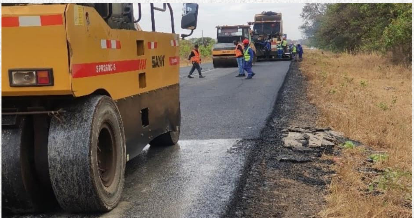
Periodic maintenance works on the Mazabuka-Monze Road.
