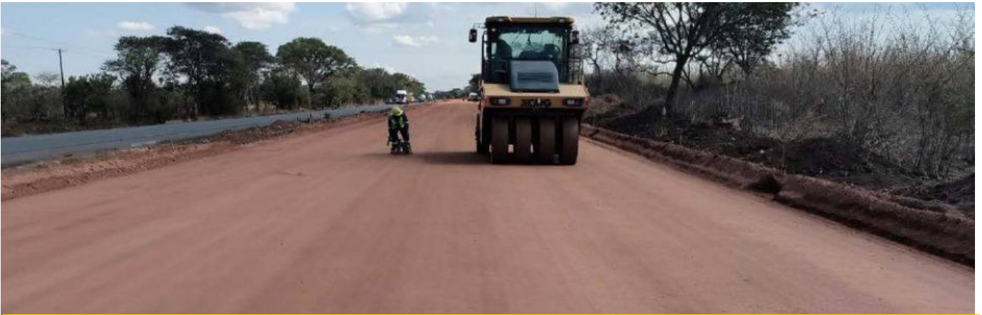
Subbase works on the Lusaka-Ndola Dual Carriageway Project.
