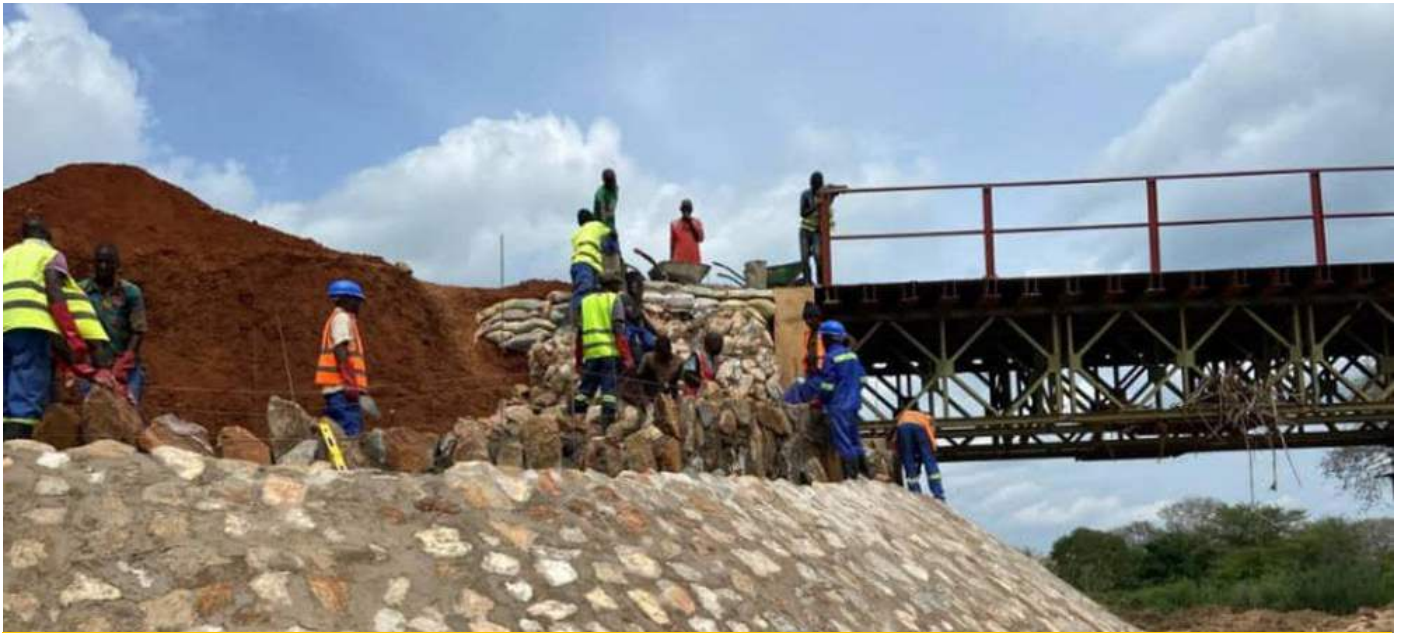
Works on the approach embankment in progress.
