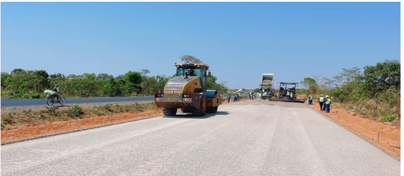
Ndola Road Dual Carriageway works.
