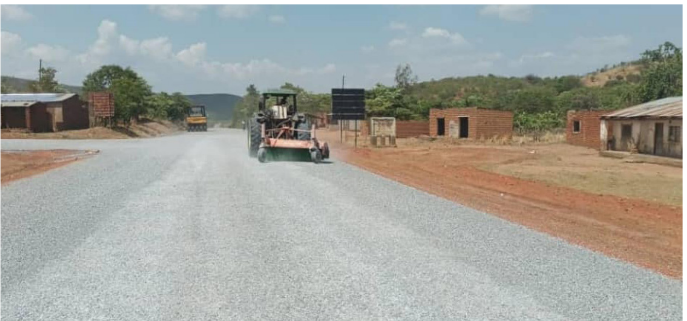
Holding maintenance works on the Chipata-Lundazi Road in Eastern Province.
