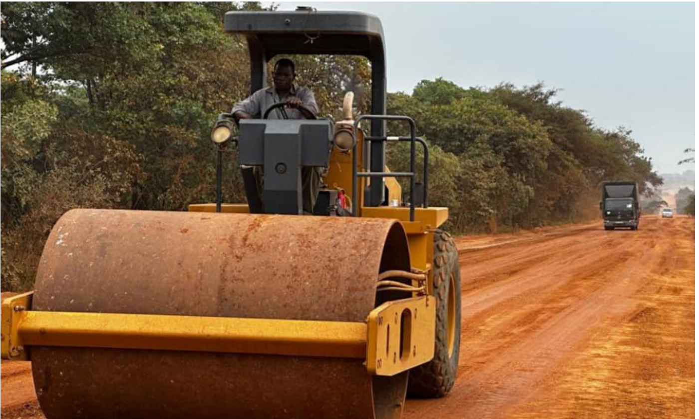
Holding maintenance works on the Mufulira-Mokambo Road on the Copperbelt Province.
