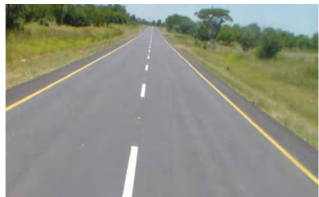
Figure 13: Completed Section of Livingstone to Sesheke road (M10)
