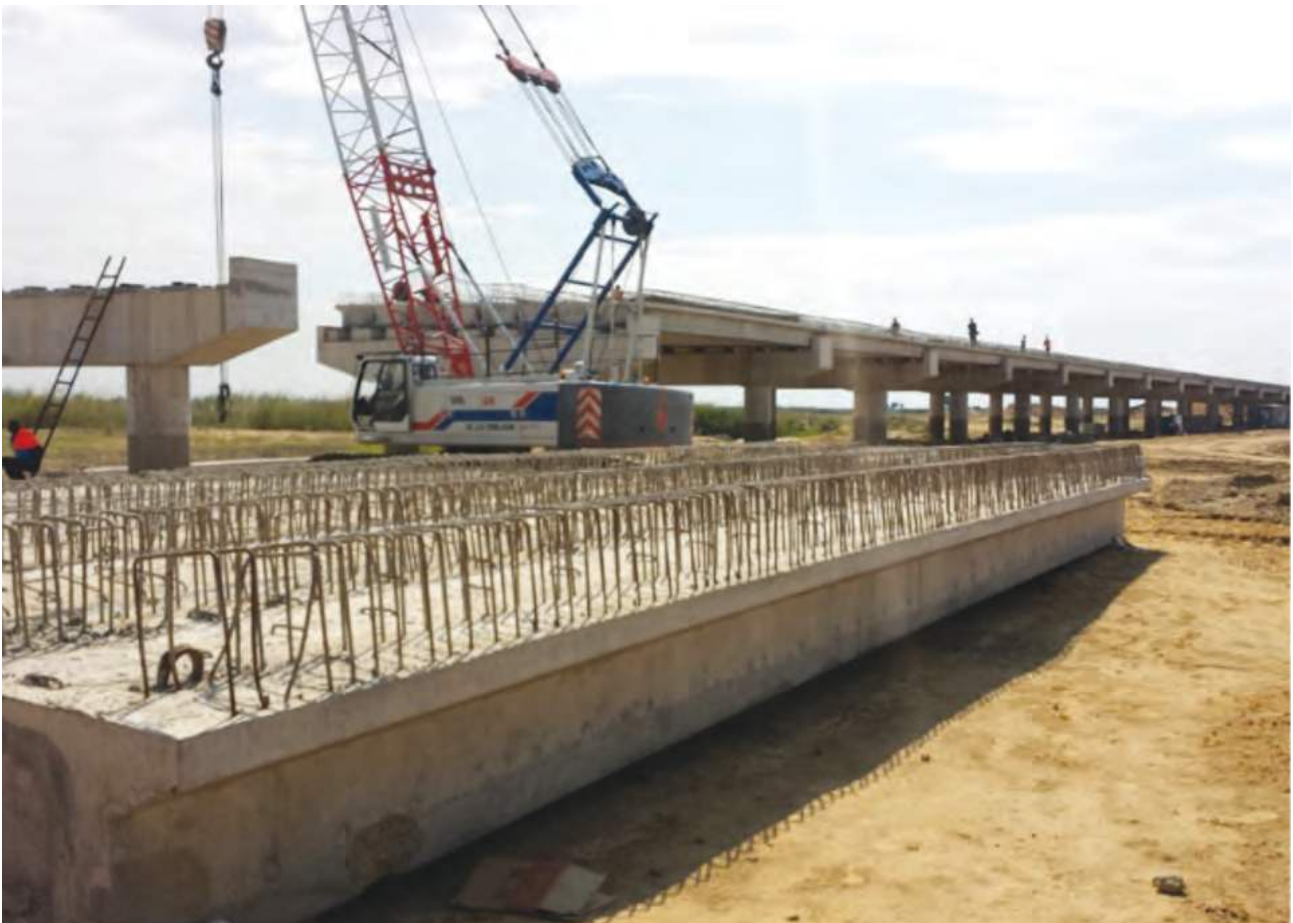
Figure 11: Bridge works in progress-Mongu-Kalabo Road
