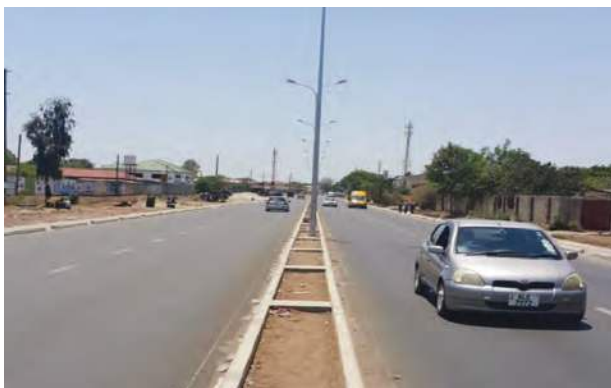
Figure 12: Newly constructed Chilimbulu Road
