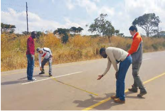
Figure 9: Pavement width measurement
