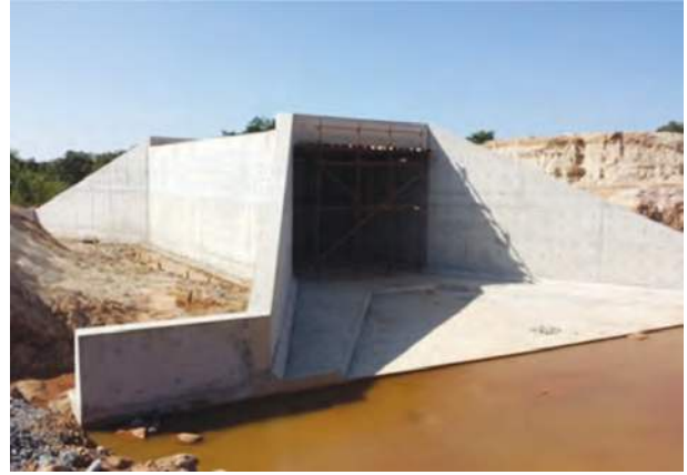
Figure 10: Box culvert under construction
