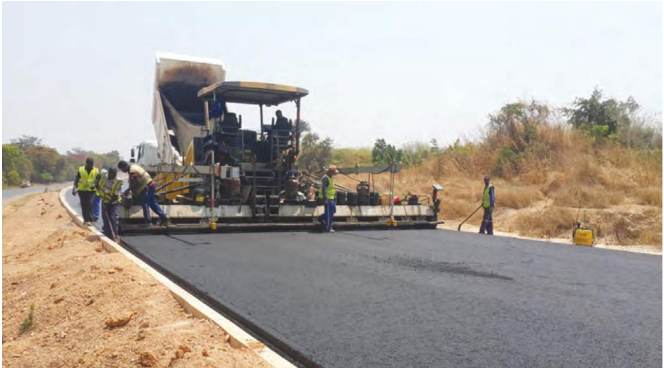
Figure 8: Asphalt Paving on the Kitwe–Chingola dual carriageway project
