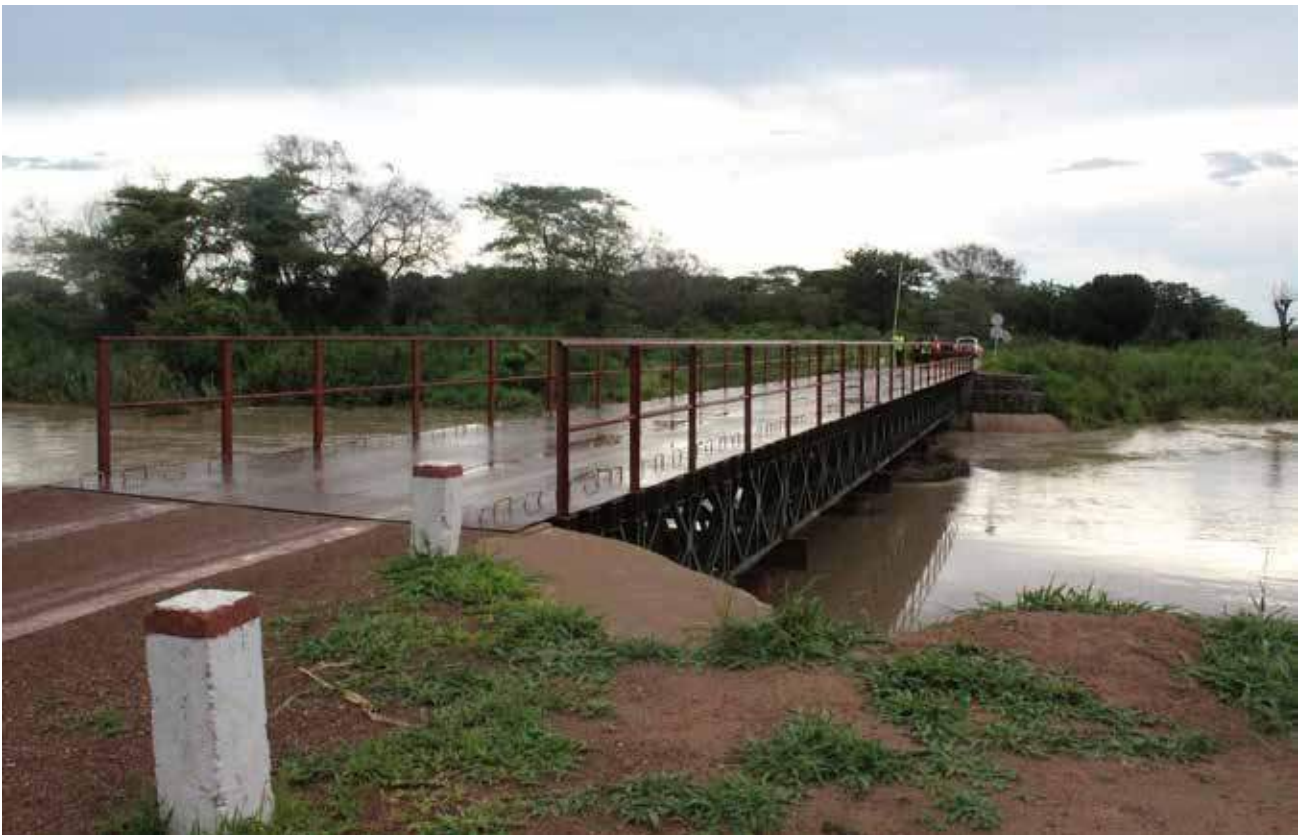
Figure 5: Completed Temporal bridge on Luangwa Matumbo Road
