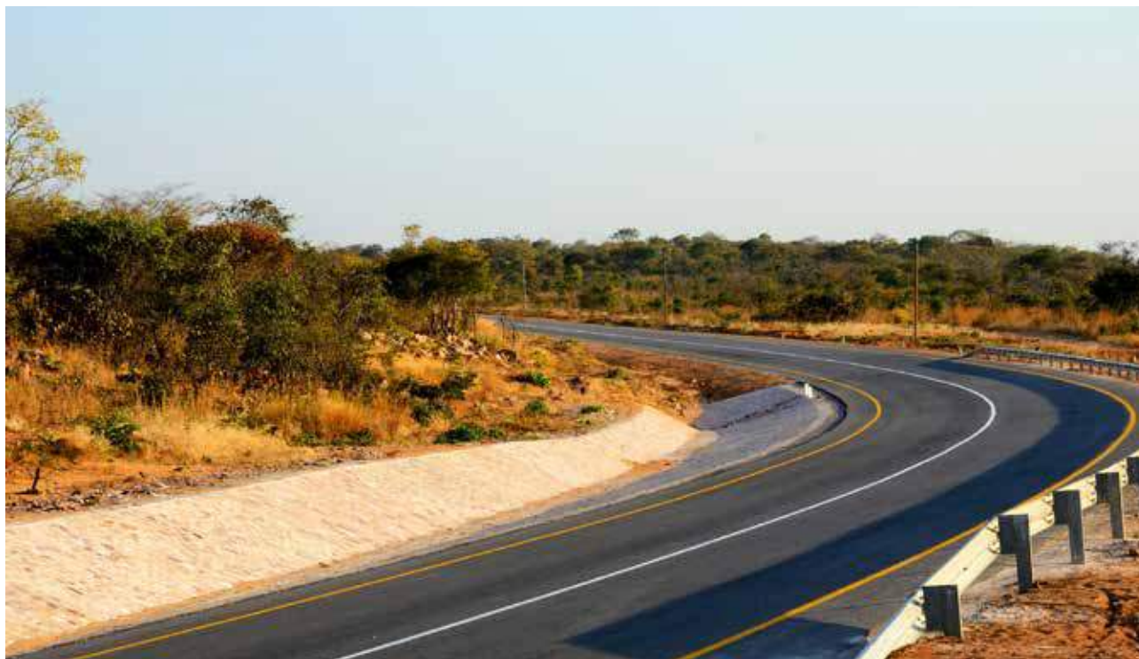
Figure 16: Rehabilitated Mansa-Luwingu road
