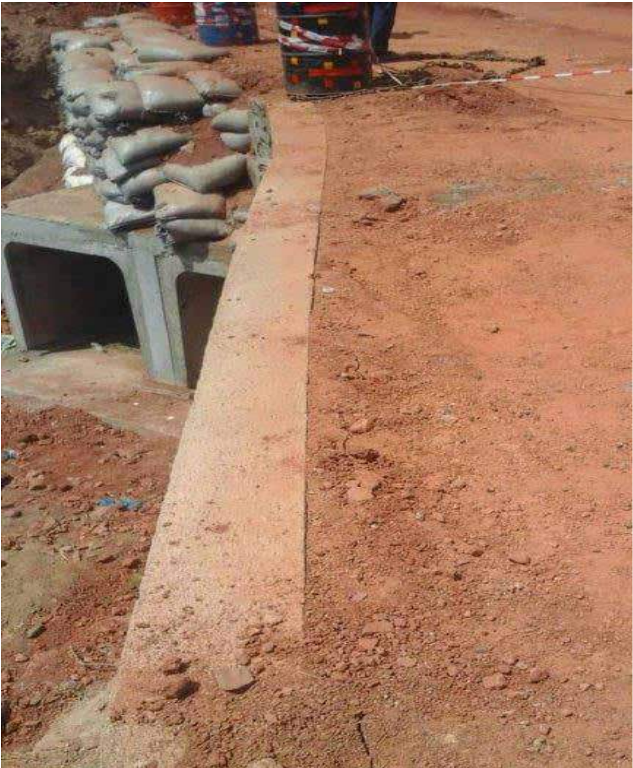
Figure 11: Final culverts at Ngozi
