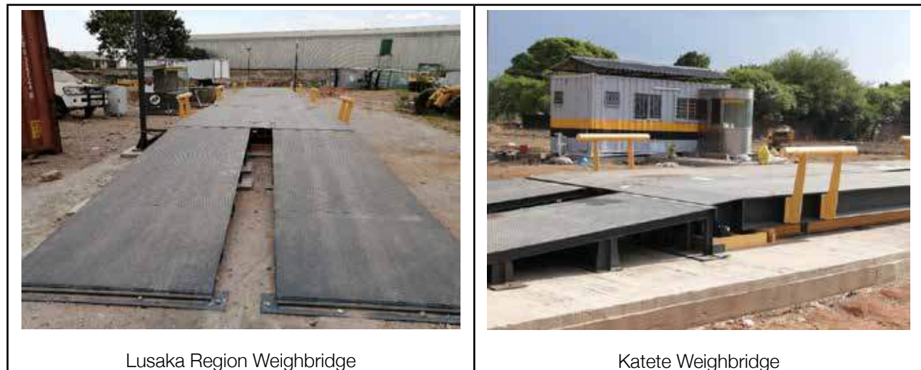
Figure 10: Weigh Bridges at two Locations
