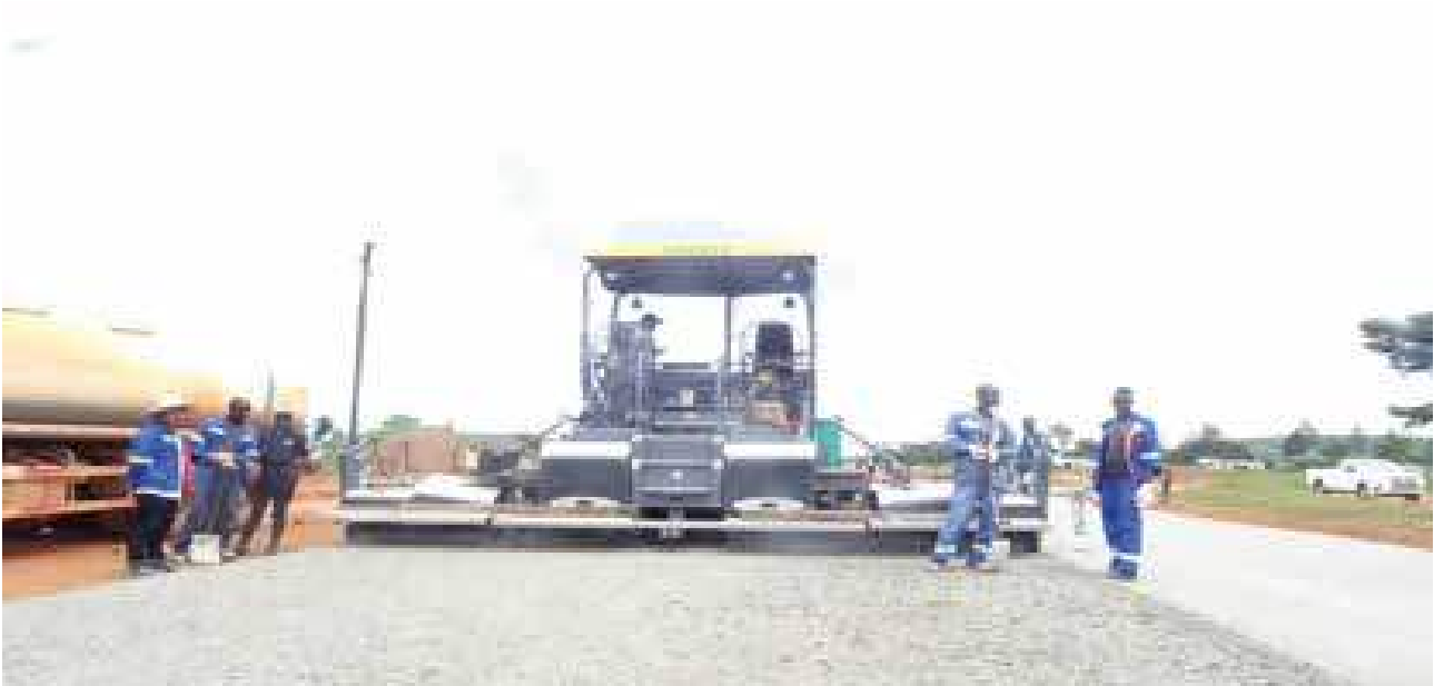
Figure 6: Rehabilitation works on the Chinsali-Nakonde road
