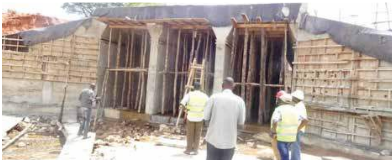
Figure 8: Lufune Box culvert under construction
