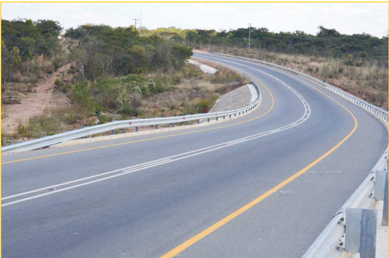
A section of the completed Leopards Hill – Katoba Road
