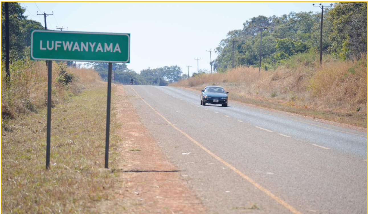
Completed section of the Kalulushi-Lufwanyama Road
