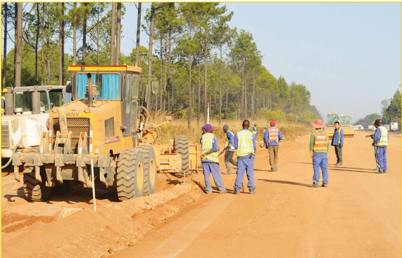
Construction works on Kitwe-Chingola dual carriageway
