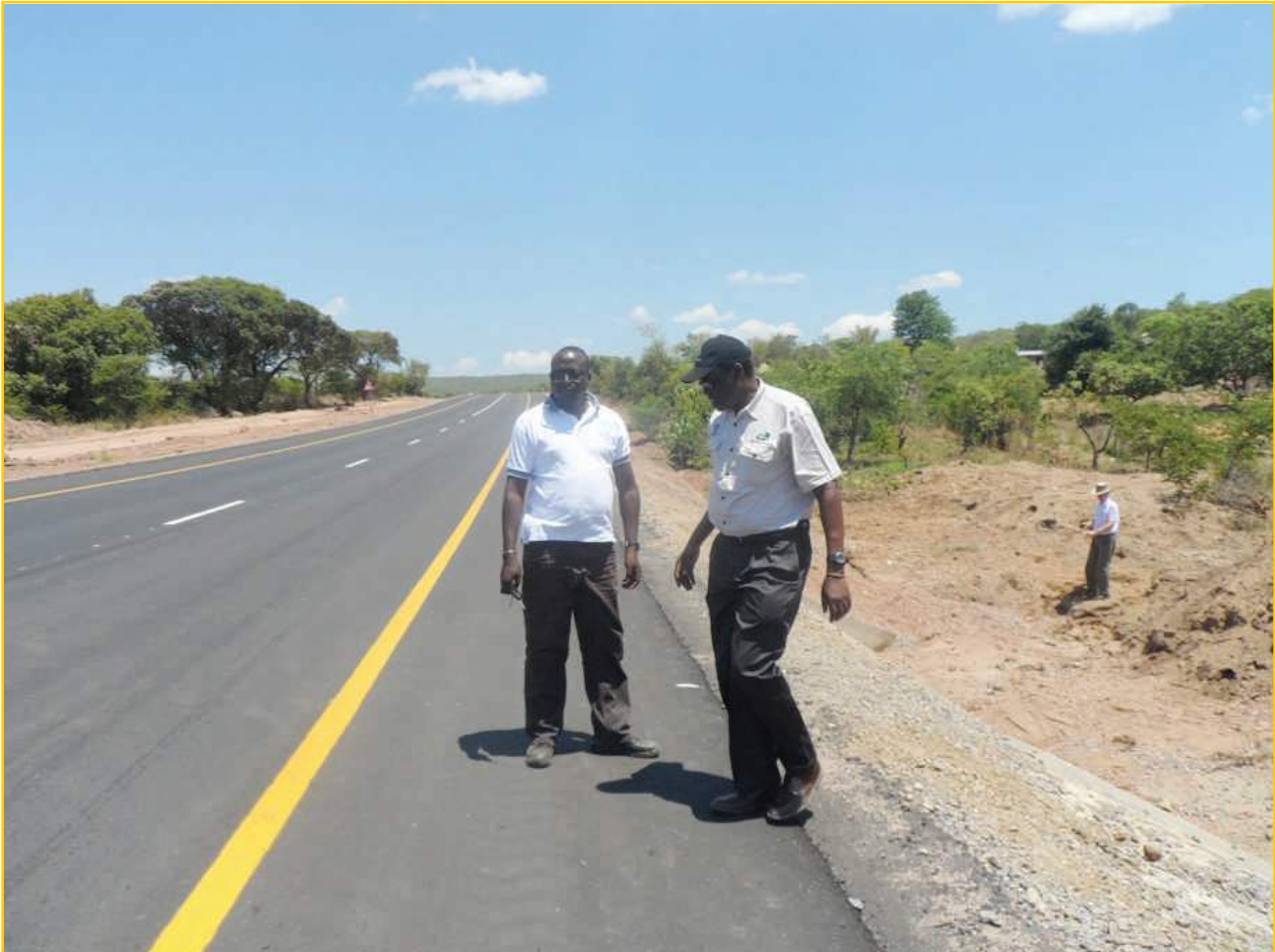
Inspection of Lusaka – Chirundu Road works
