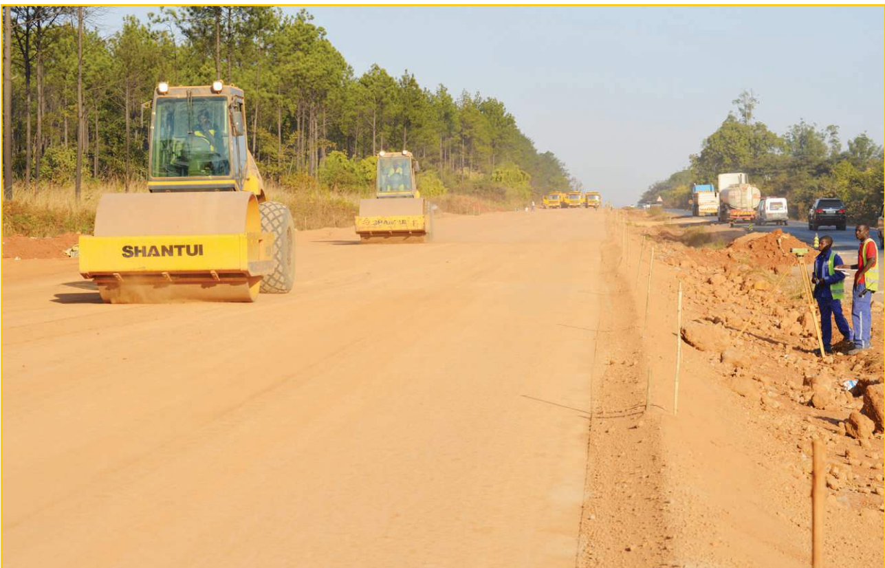
Construction works on Kitwe-Chingola dual carriageway
