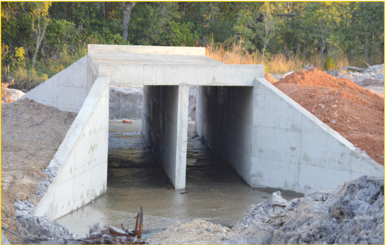
Box Culvert under construction
