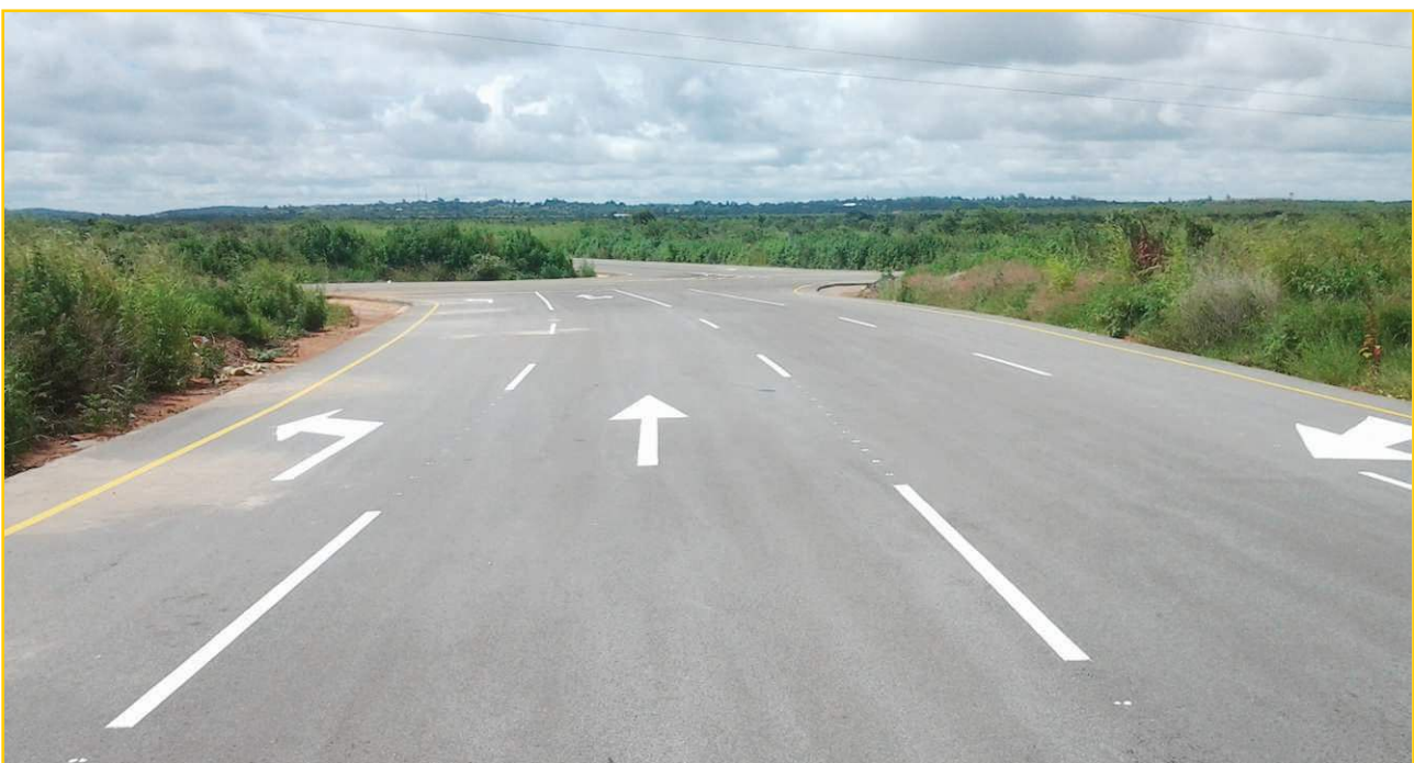
Completed roads at the Multi Facility Economic Zone in Lusaka South
