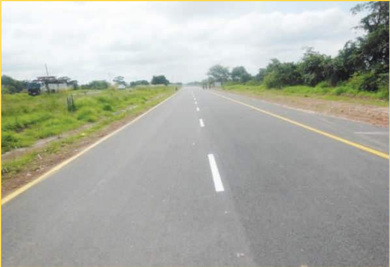
Completed section of the Ndola-Kitwe Dual Carriageway
