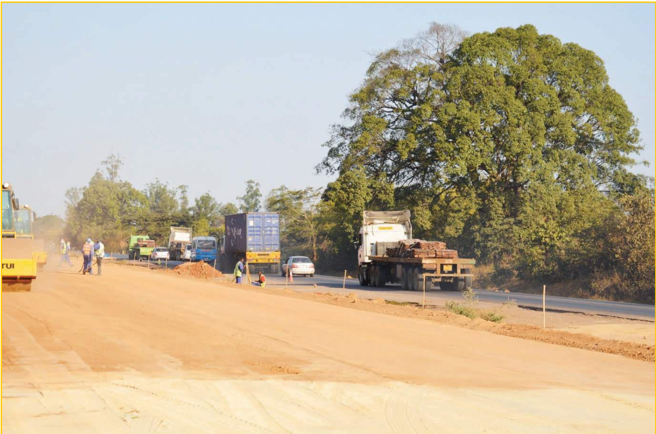
Works on Chingola – Kitwe dual carriageway
