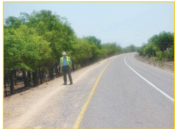
Completed section of Mansa Nchelenge
