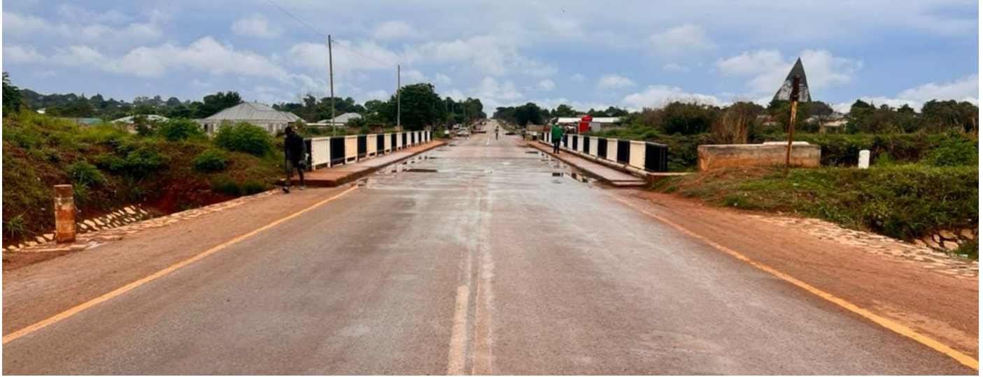
Lukashya Bridge in Kasama District.
