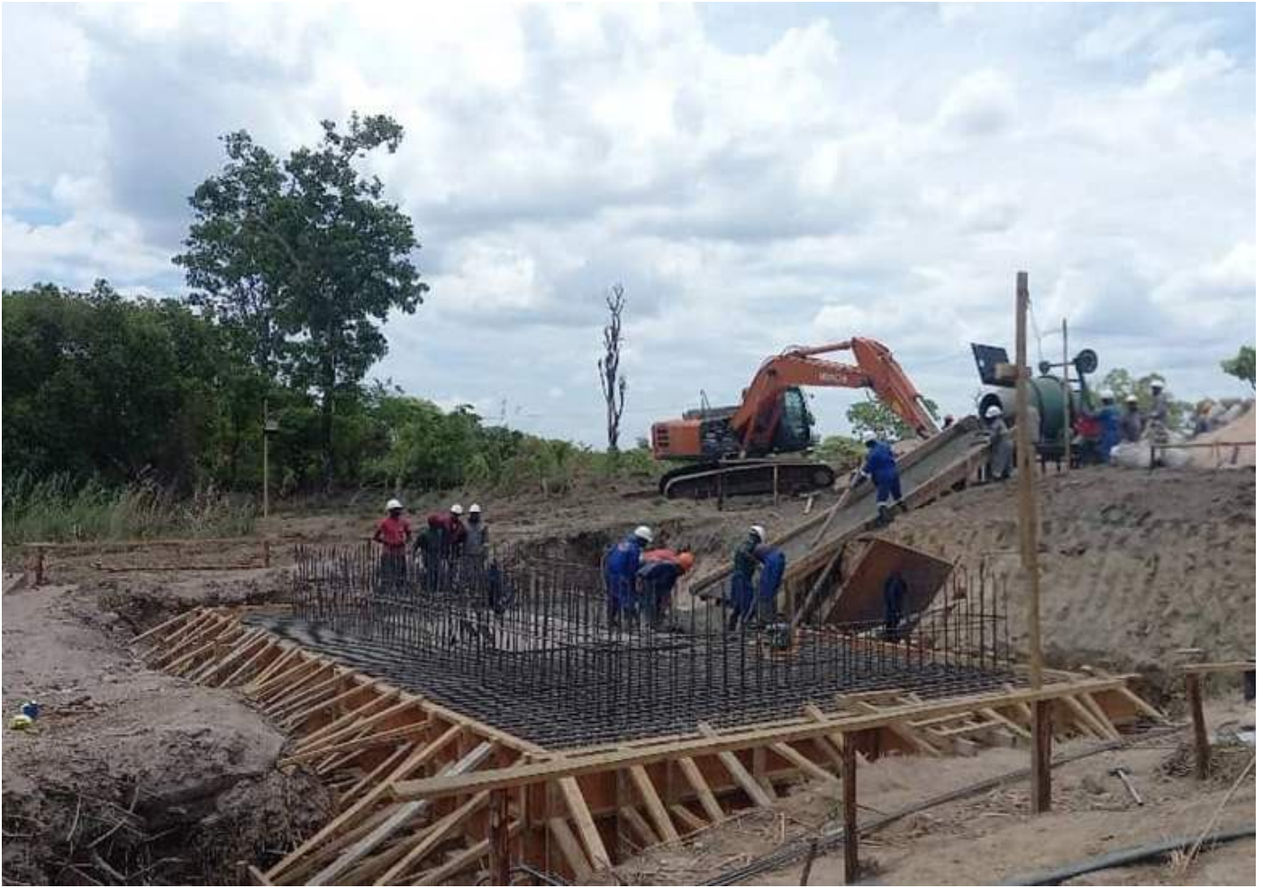
Construction works of the Aluni Mulonga ACROW Bridge.
