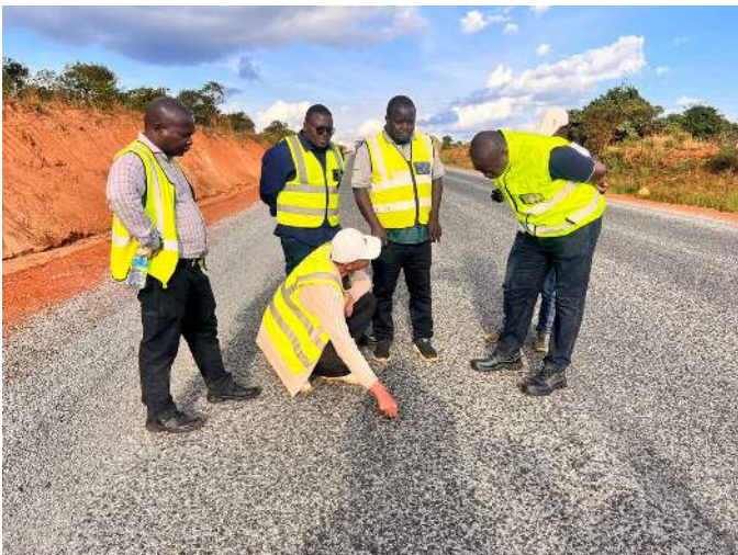
Checking on the pavement structure.
