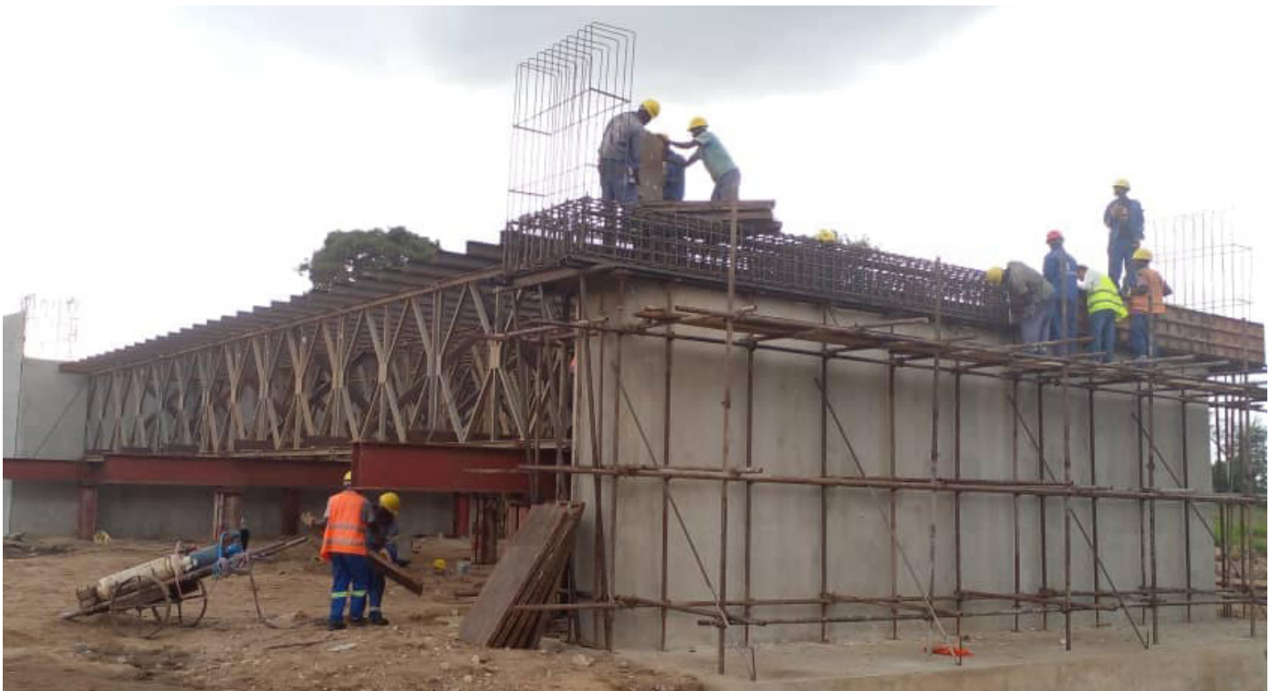
Kampemba Bridge under construction.
