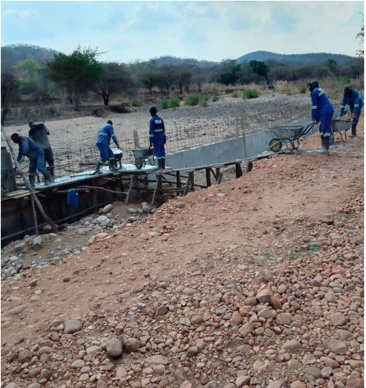
Construction of the retaining wall to protect the road embankment and Mwateshi Bridge in Rufunsa District.
