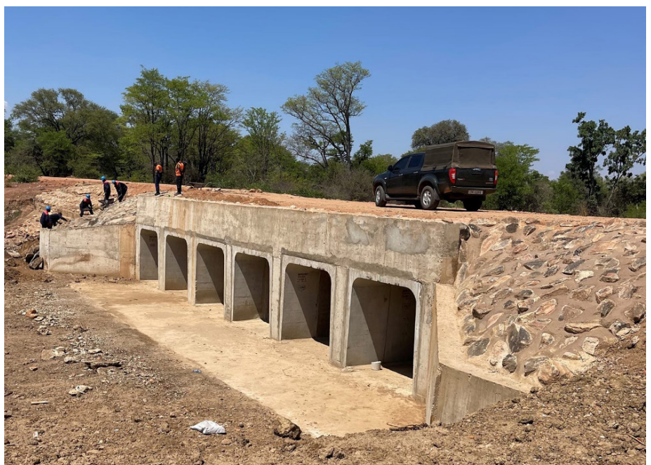
Six lines Dongo culvert along the Kalomo-Dundumwezi-Itezhi Tezhi Road in Southern Province.
