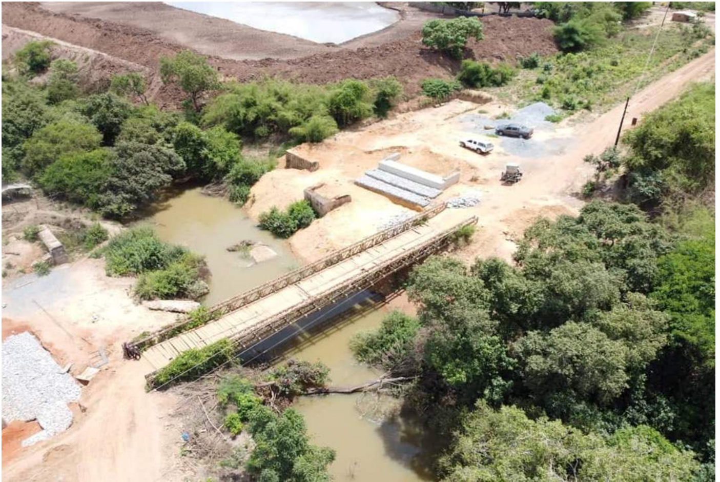
An aerial view of the 51.67 metres long ACROW Bridge being constructed across the Luombwa River in the Nasanga Farming Block of Serenje District in Central Province.
