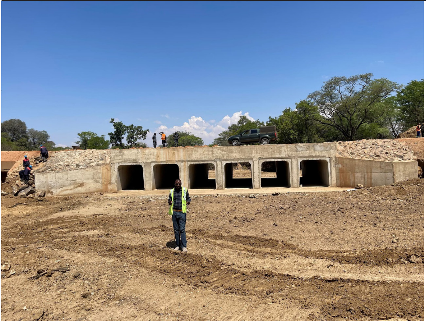
Six lines Dongo culvert along the Kalomo-Dundumwezi-Itezhi Tezhi Road in Southern Province.
