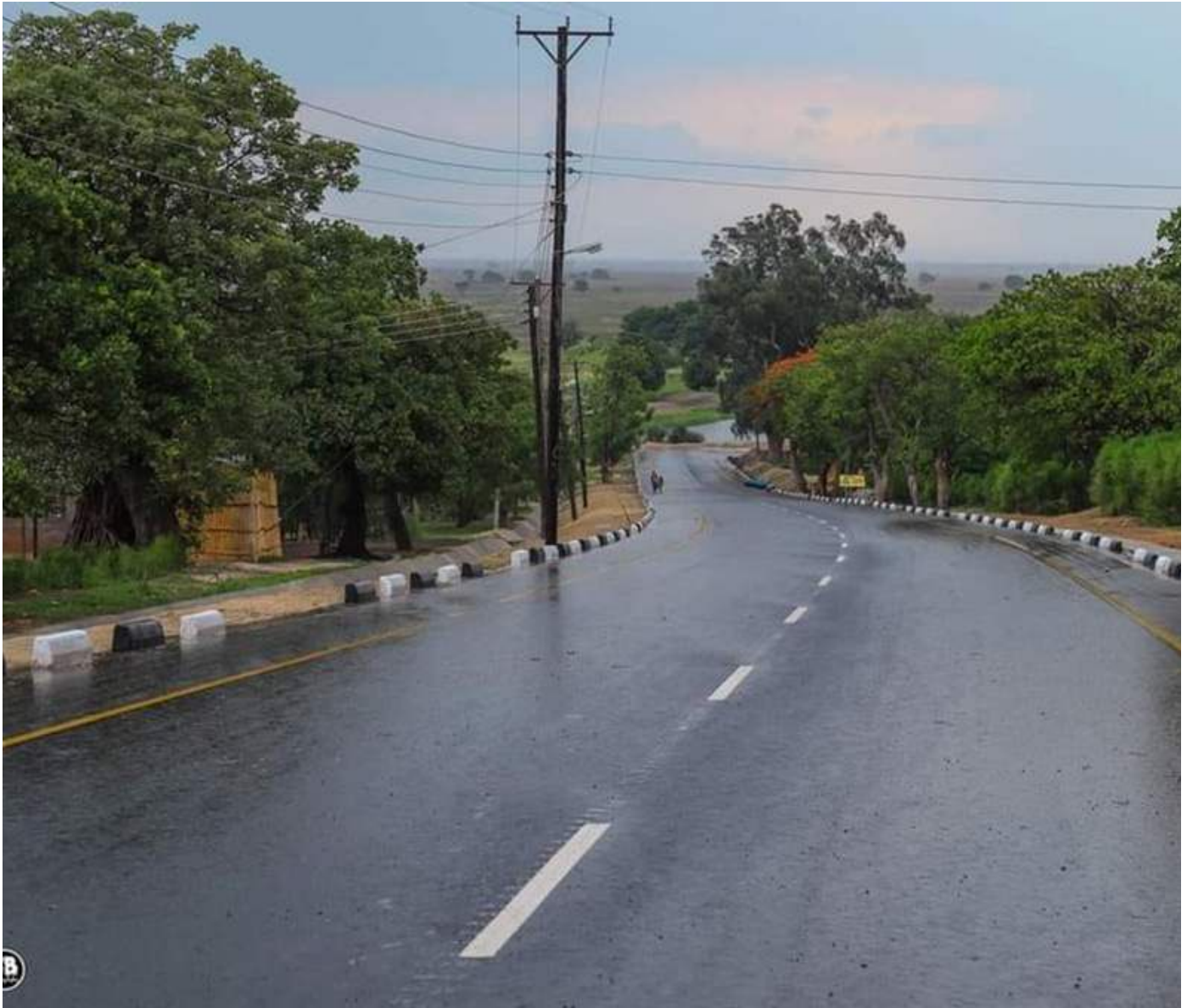
Newly rehabilitated Mongu-Limulunga Road.
