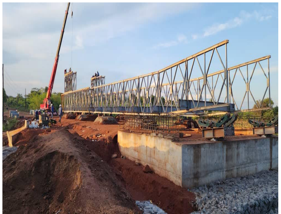
Launching of ACROW Bridge components.
