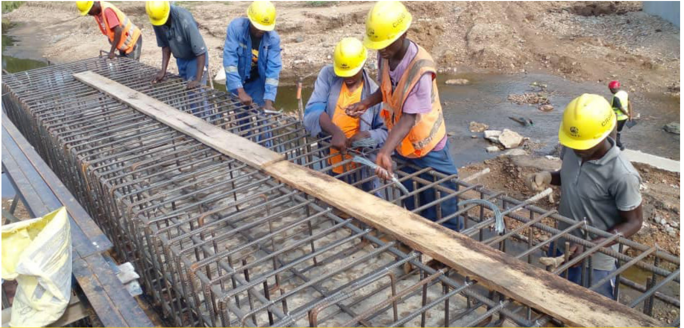
Steel works underway at Kampemba Bridge.
