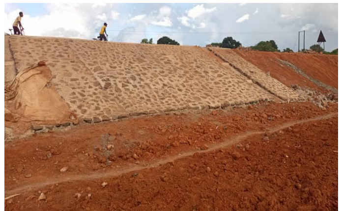
More images from Lundazi Bridge under construction.
