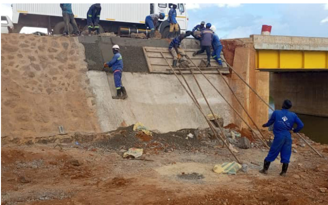
Protection works on the embankments in progress.
