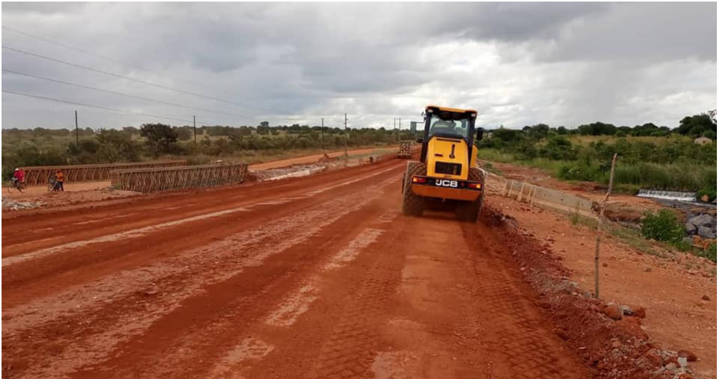
Base course stabilization works at Msuzi Box Culvert.
