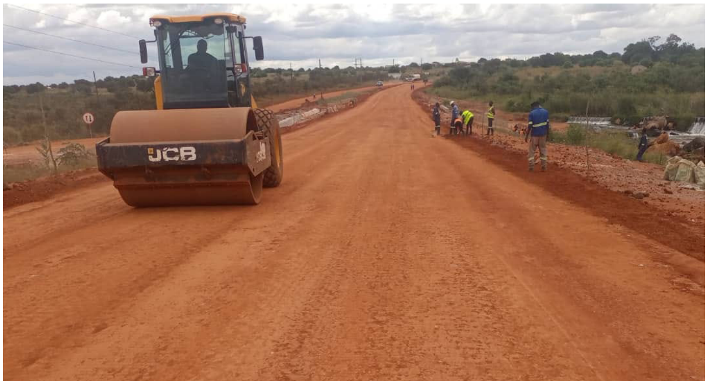
Completed base course stabilization.
