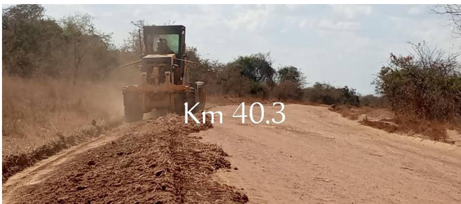
Road formation works in progress.
