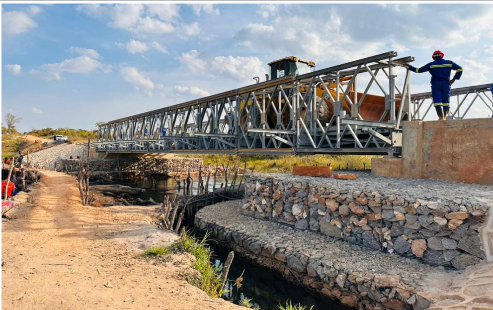
Completed Lukulu ACROW Bridge.
