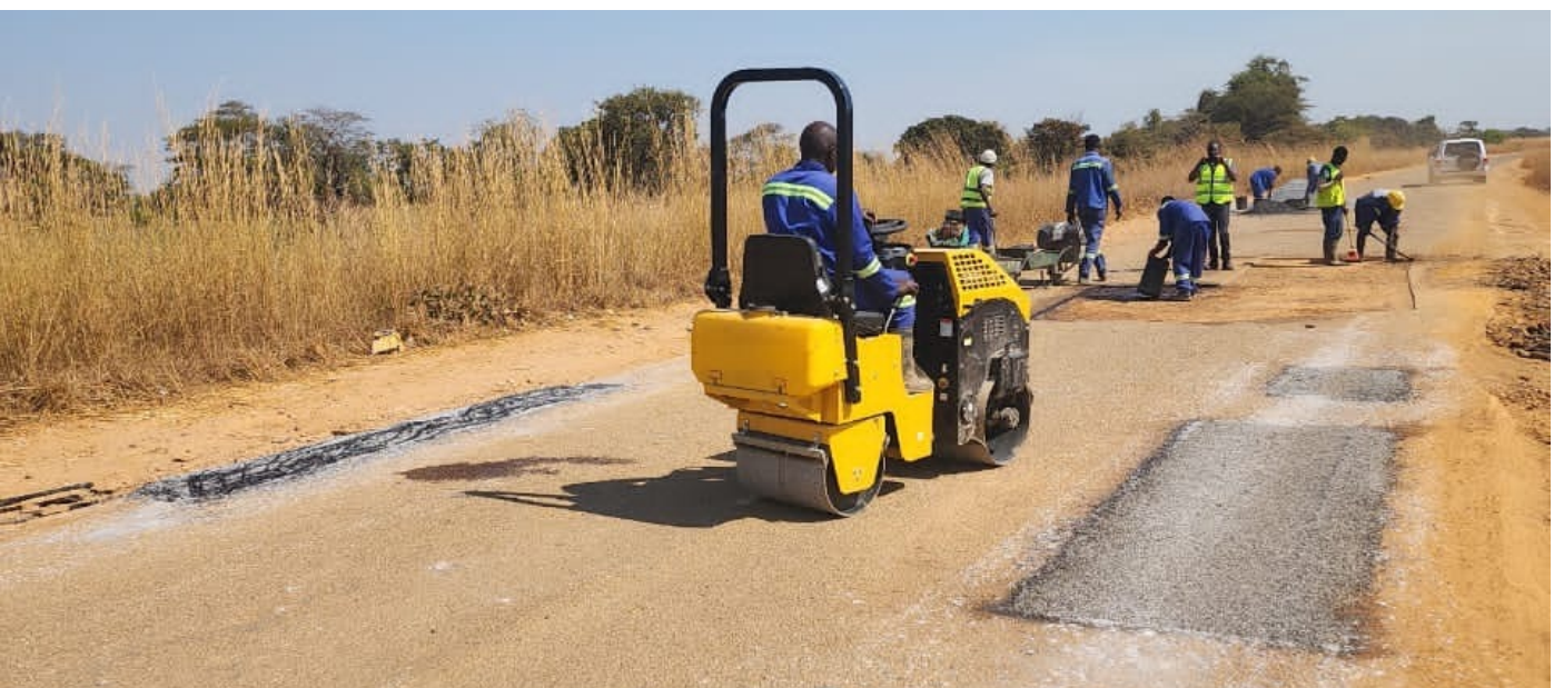
Pothole patching works in progress.
