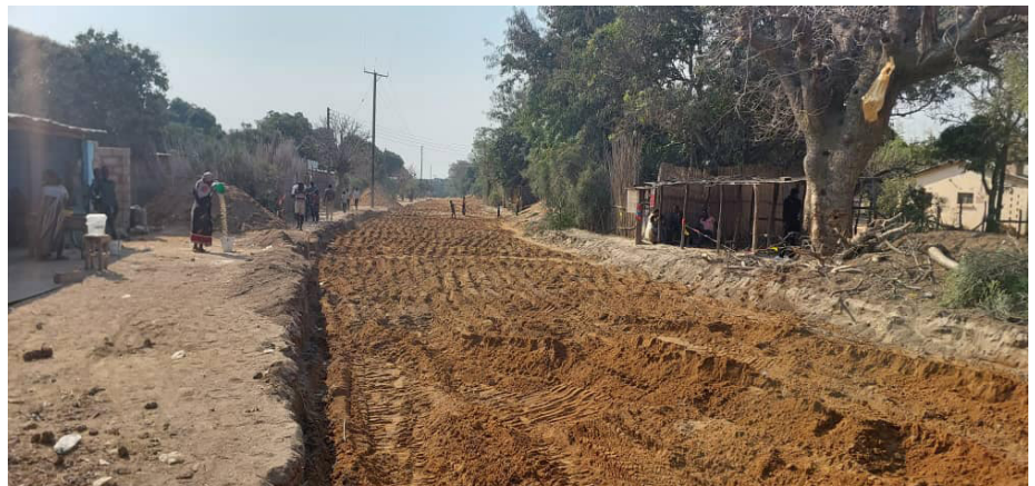
Extension works of the Mongu-Limulunga Road.
