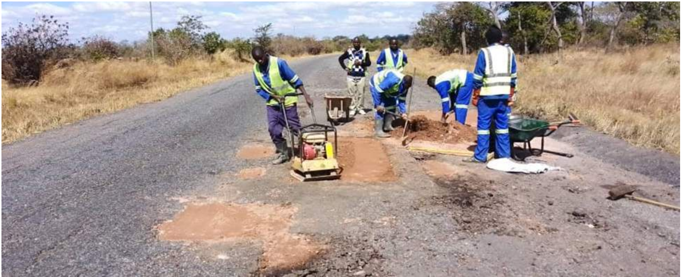
Cement stabilised gravel pothole patching works in progress.
