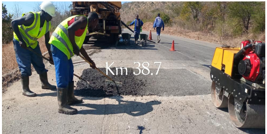
Pothole patching in progress.
