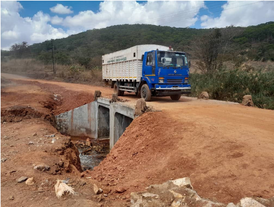
Drainage structure construction works on the Chipata-Magwero Road.
