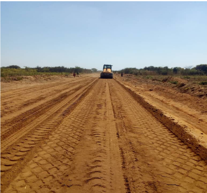
One of the access roads to a tourism site being worked on in Muchinga Province.
