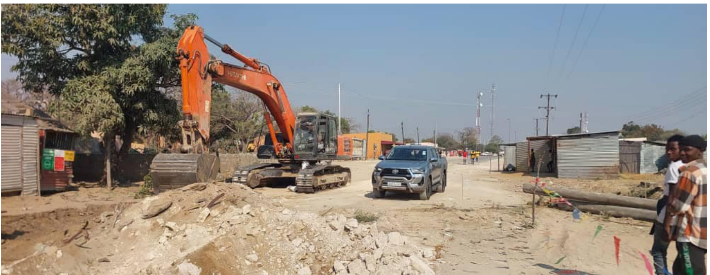
Excavation works in progress.
