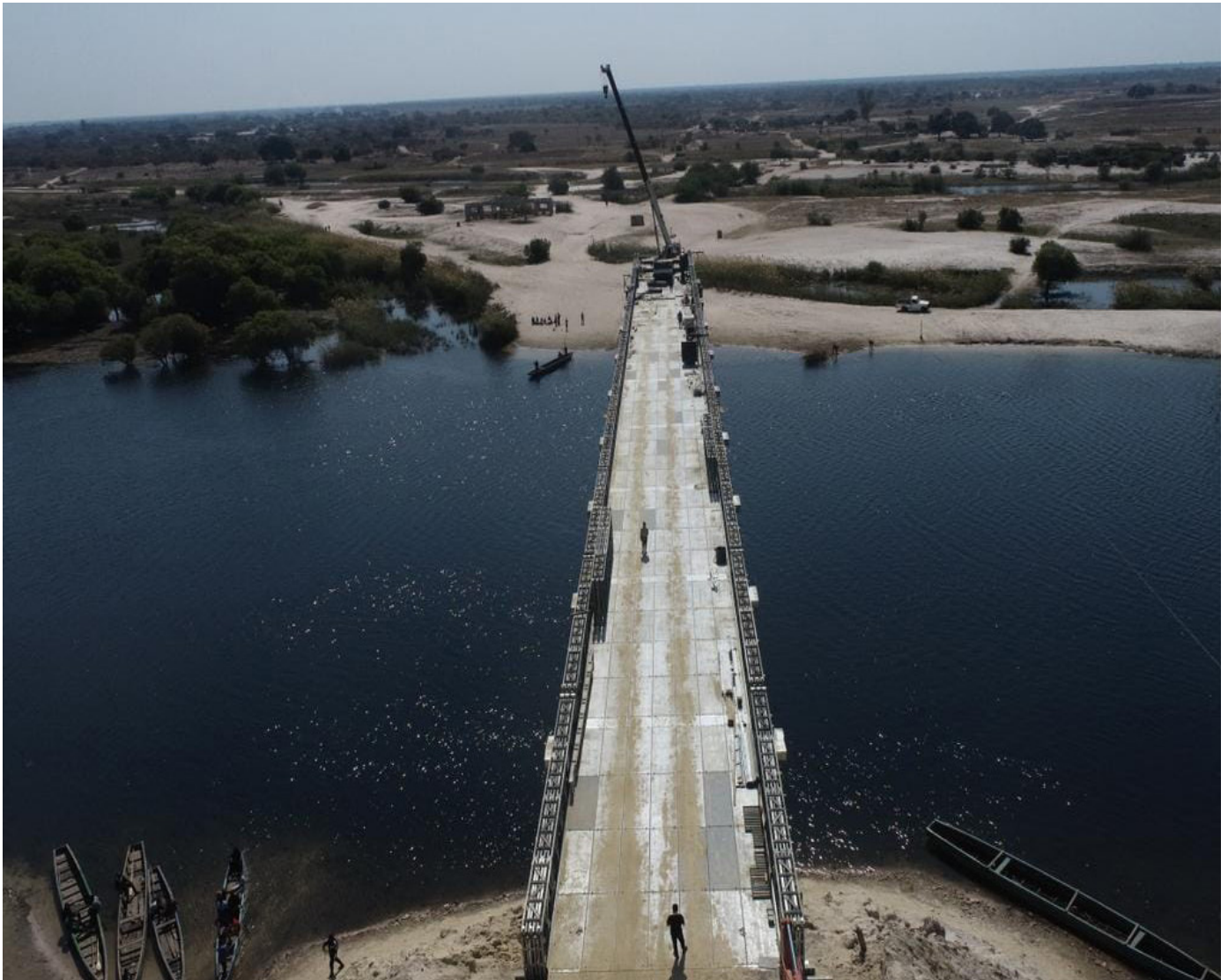
An aerial view of Luanginga Bridge under construction.
