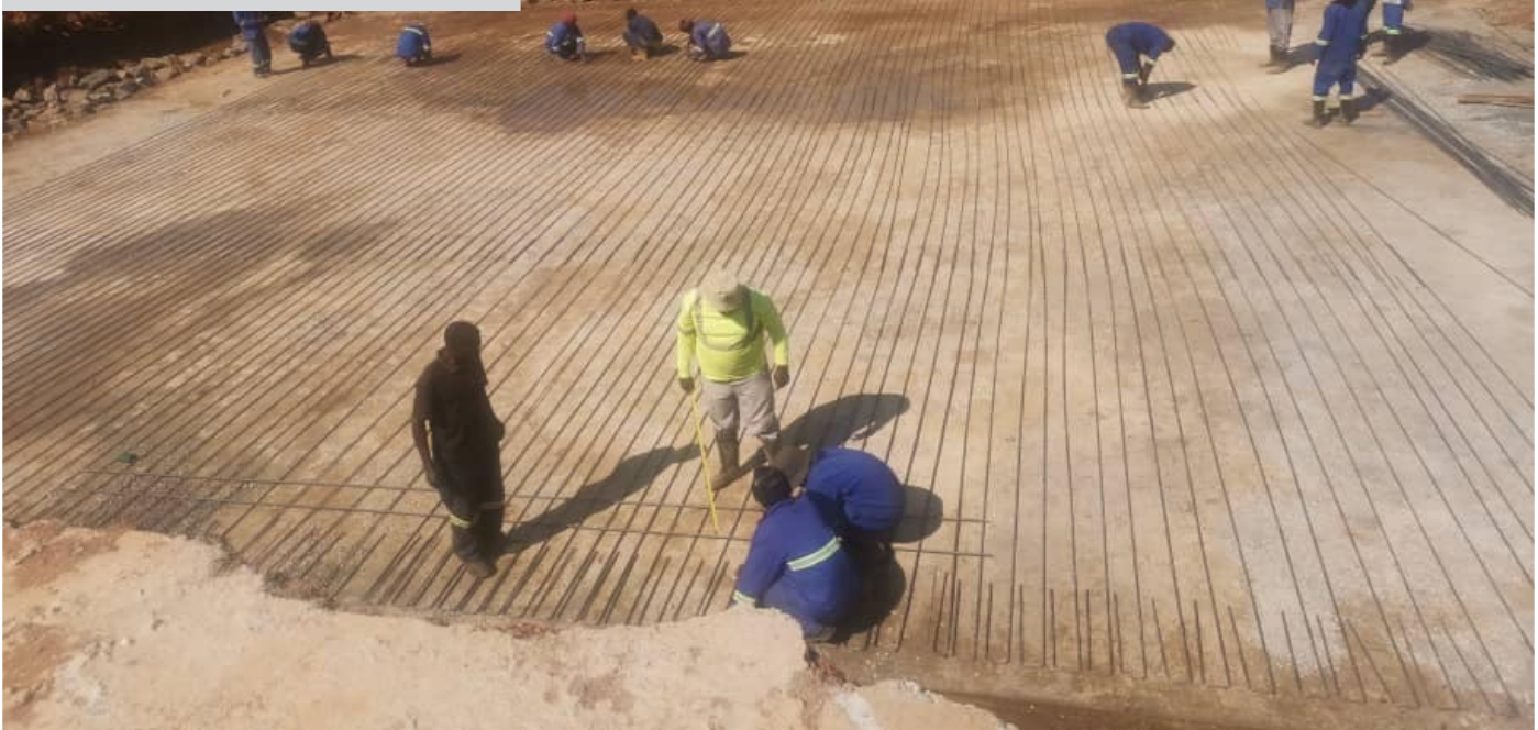
Blinding concrete works.
