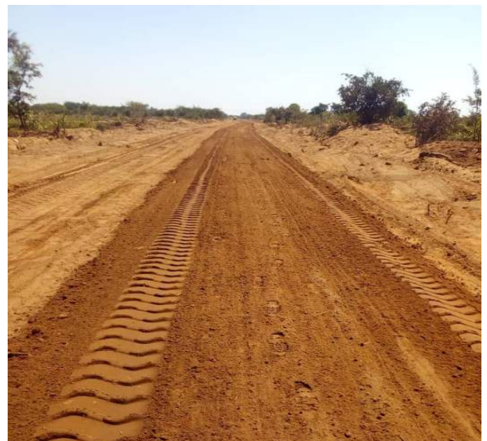
The access road to the Leshina Graveyard site.
