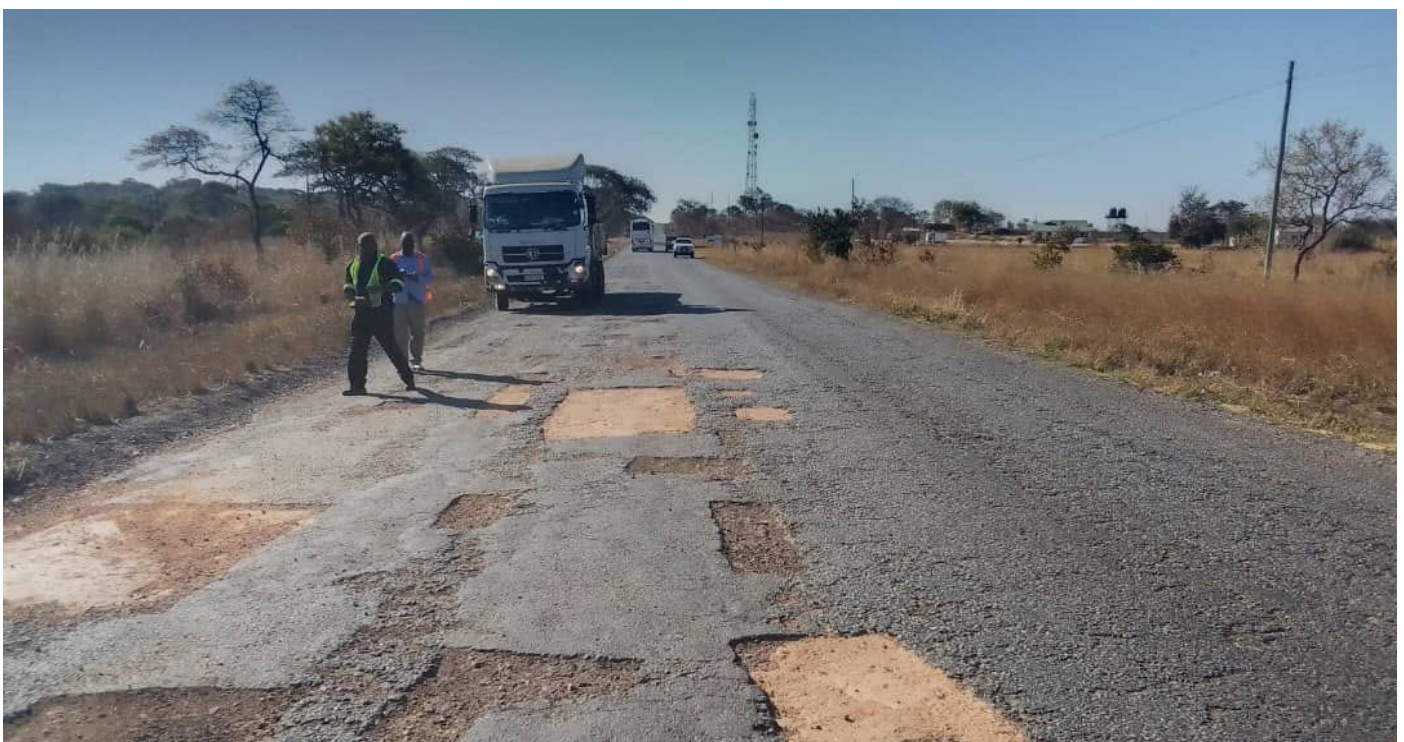
Pothole shaping works.
