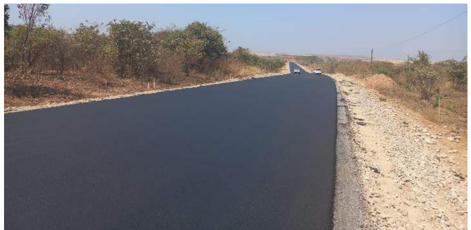
A completed section of the Chingola-Kasumbalesa Road.
