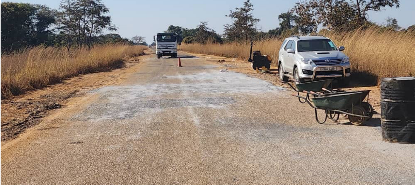
The patched section of the Tutu Road.
