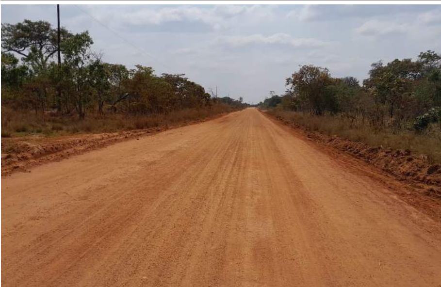
A section of the Chama-Lundazi Road.
