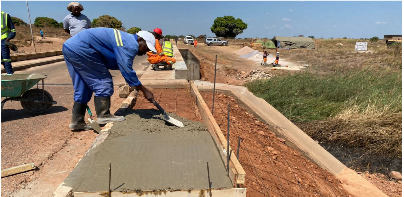
Kazembe Twin Bridges maintenance works on.
