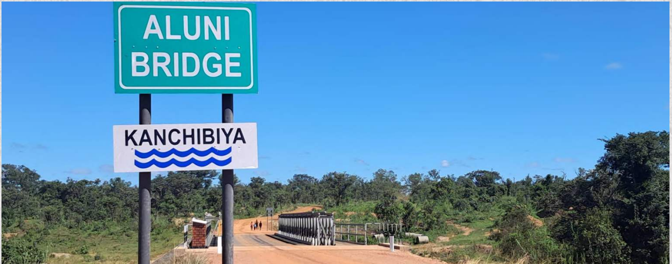
The newly commissioned Aluni-Mulonga ACROW Bridge in Kanchibiya District.
