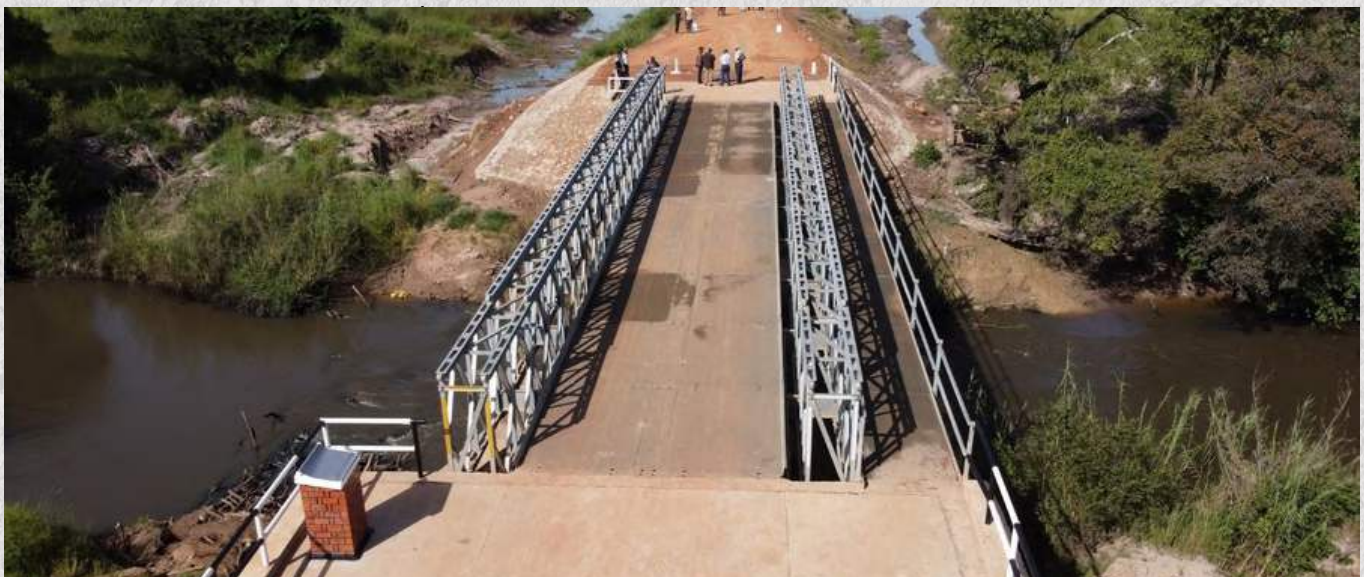
The commissioned Lwitikila ACROW Bridge.
