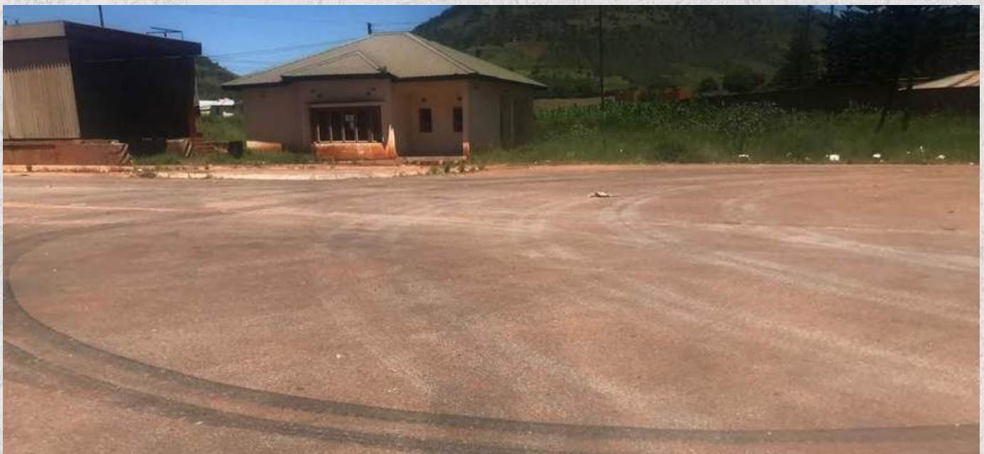
Closed Mwami Weighbridge in Eastern Province.
