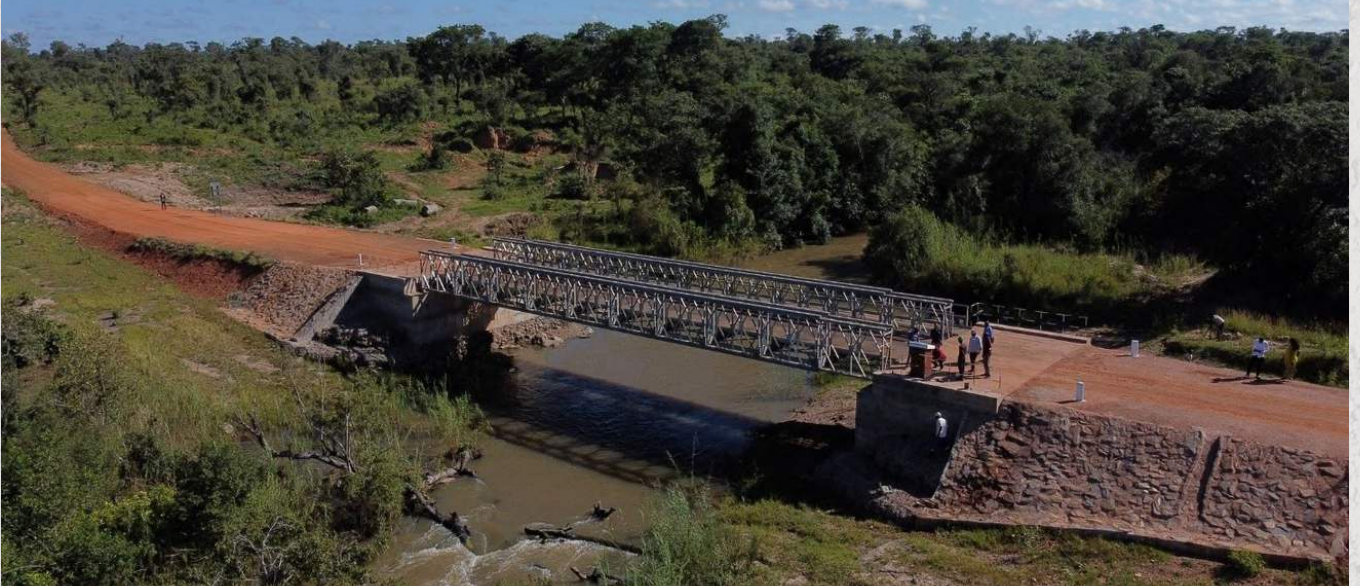
The Aluni-Mulonga ACROW Bridge at a bird's eye view.
