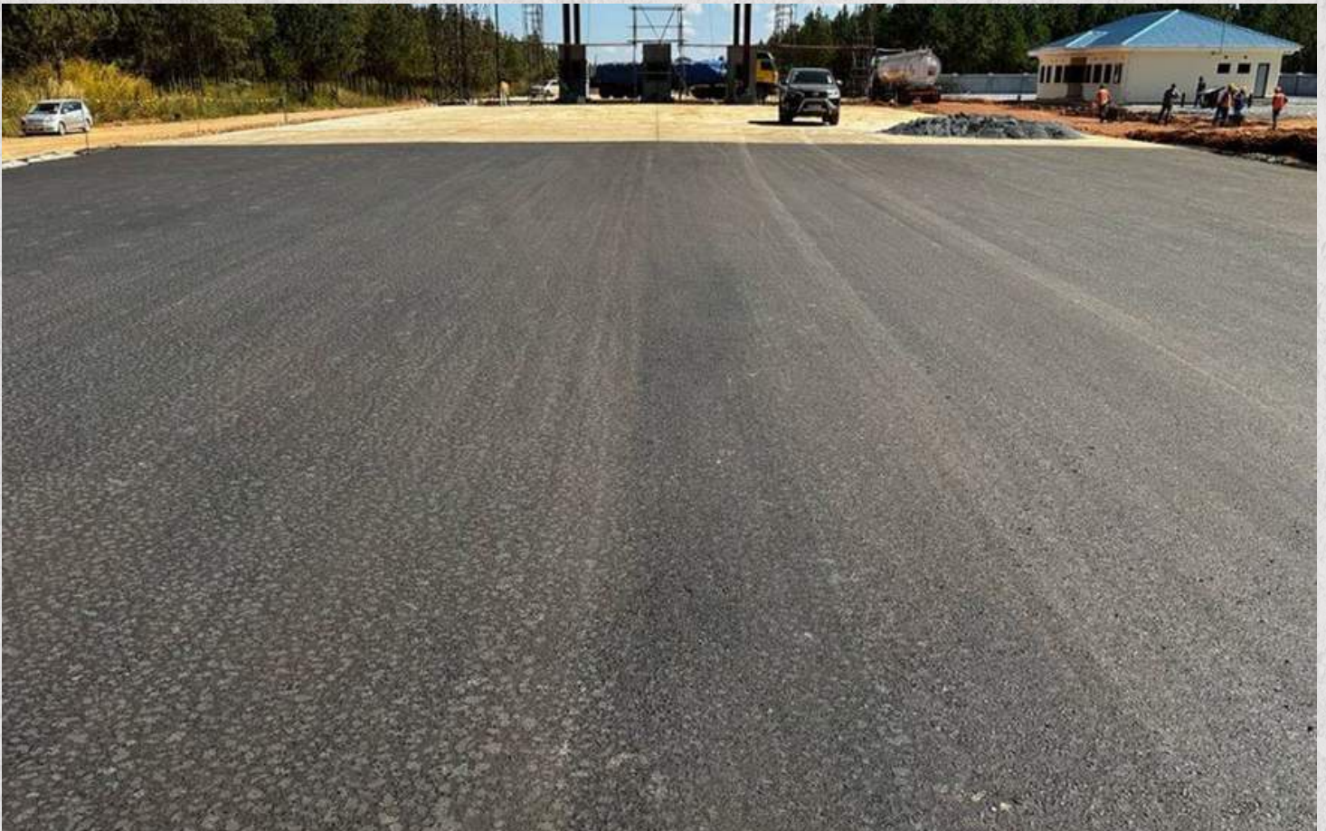
Rehabilitation works on the Ndola-Sakania-Mufulira Road.
