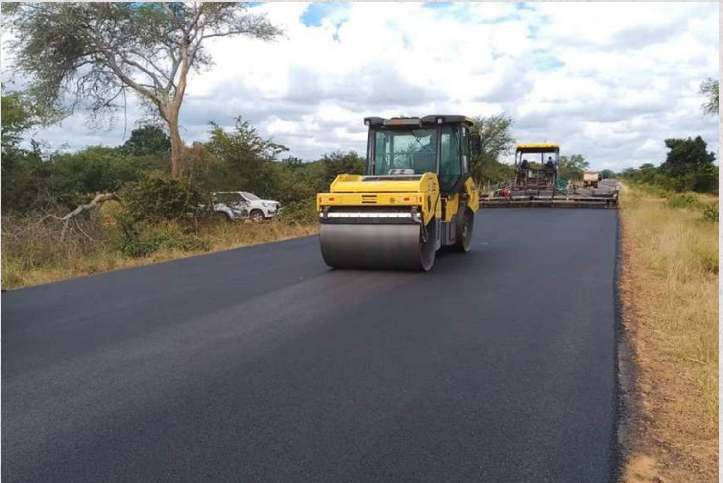
Construction works on the Monze-Niko Road in Southern Province.
