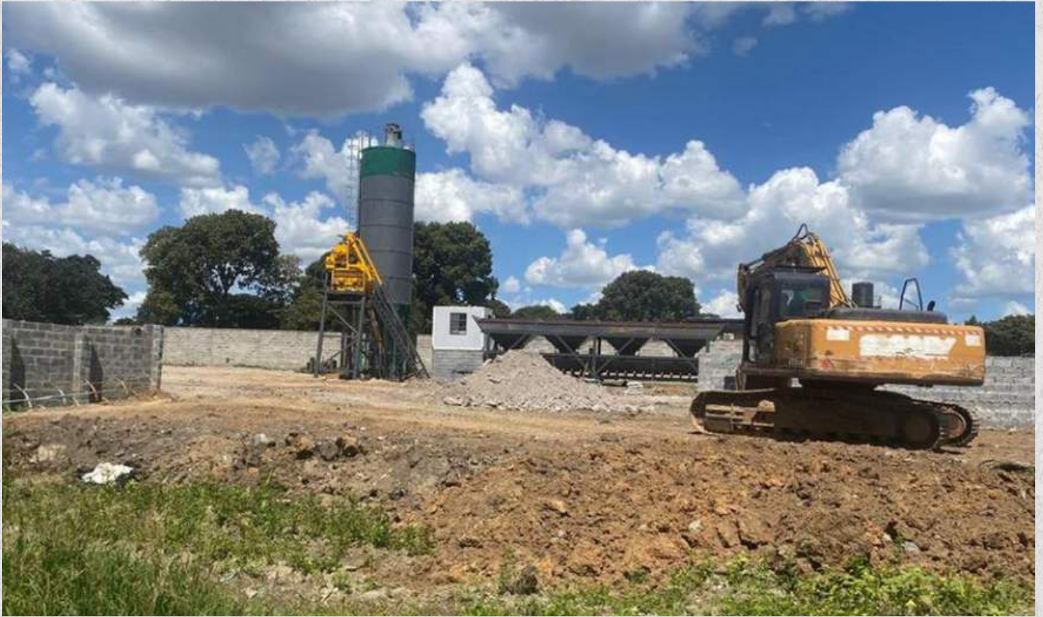
The construction camp for the Kafubu Bridge in Ndola.
