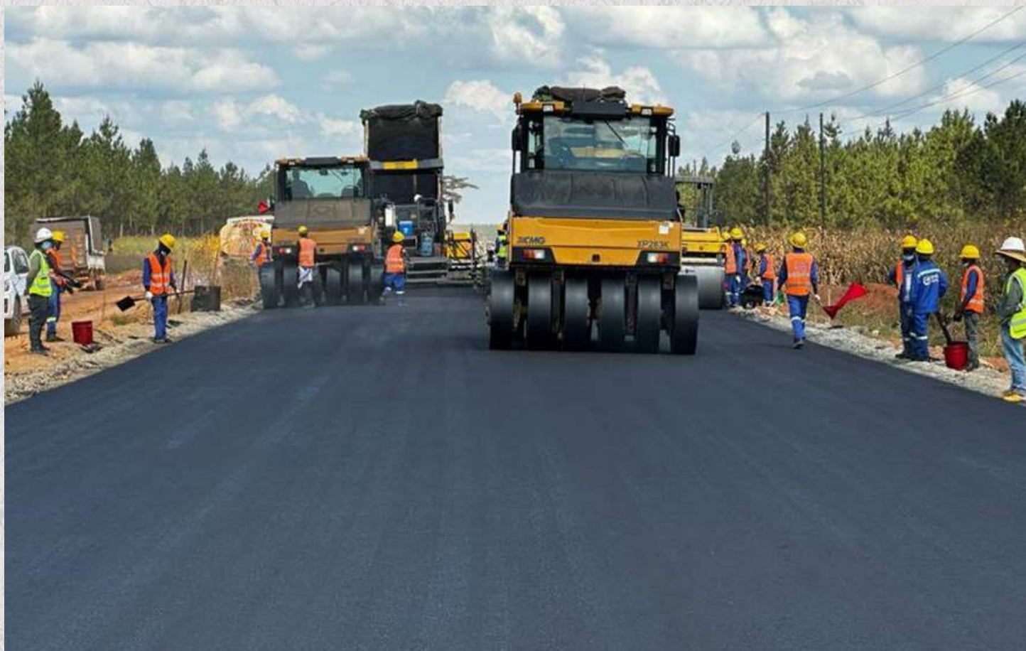
Rehabilitation works on the Ndola-Sakania-Mufulira Road on the Copperbelt.
