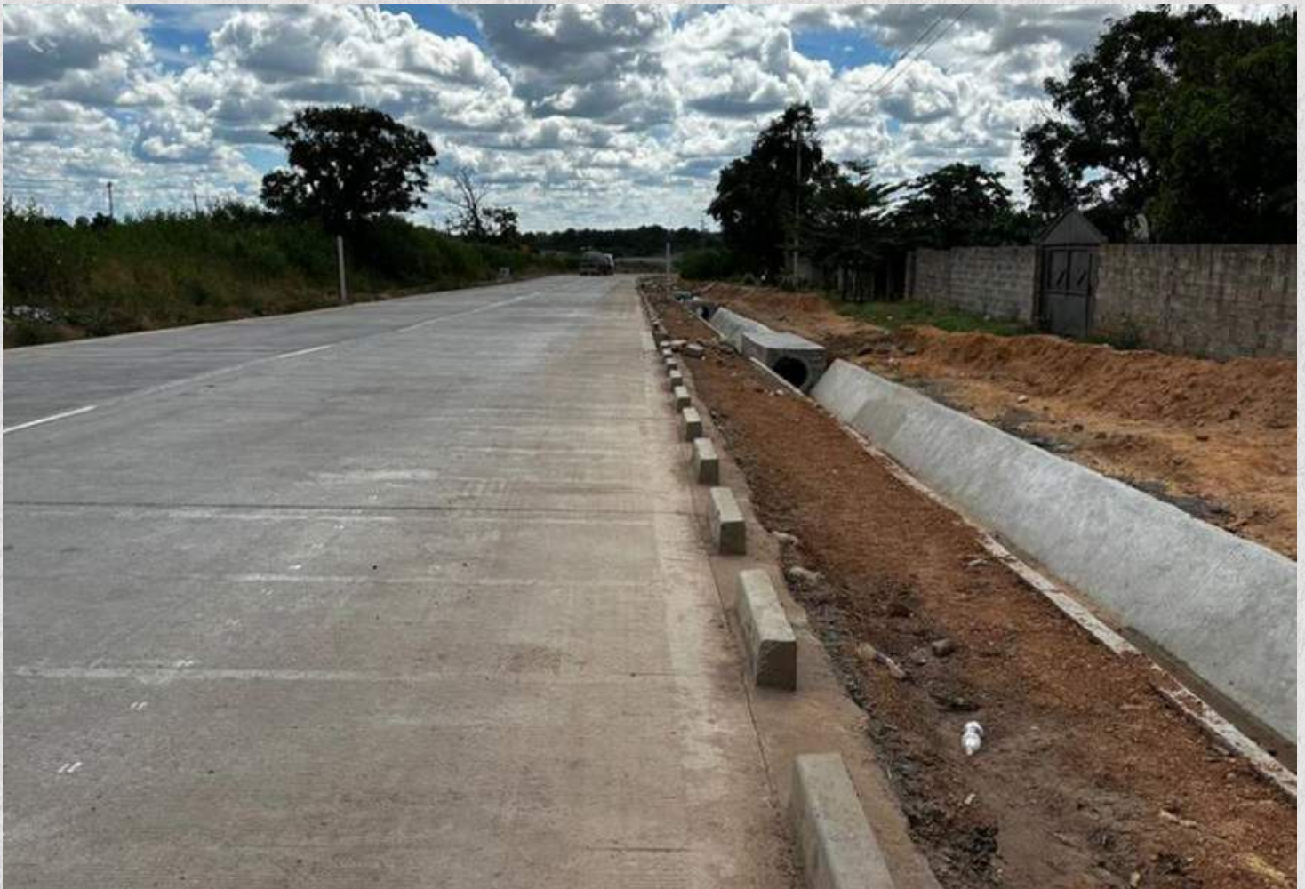
Chibuluma Road construction works.
