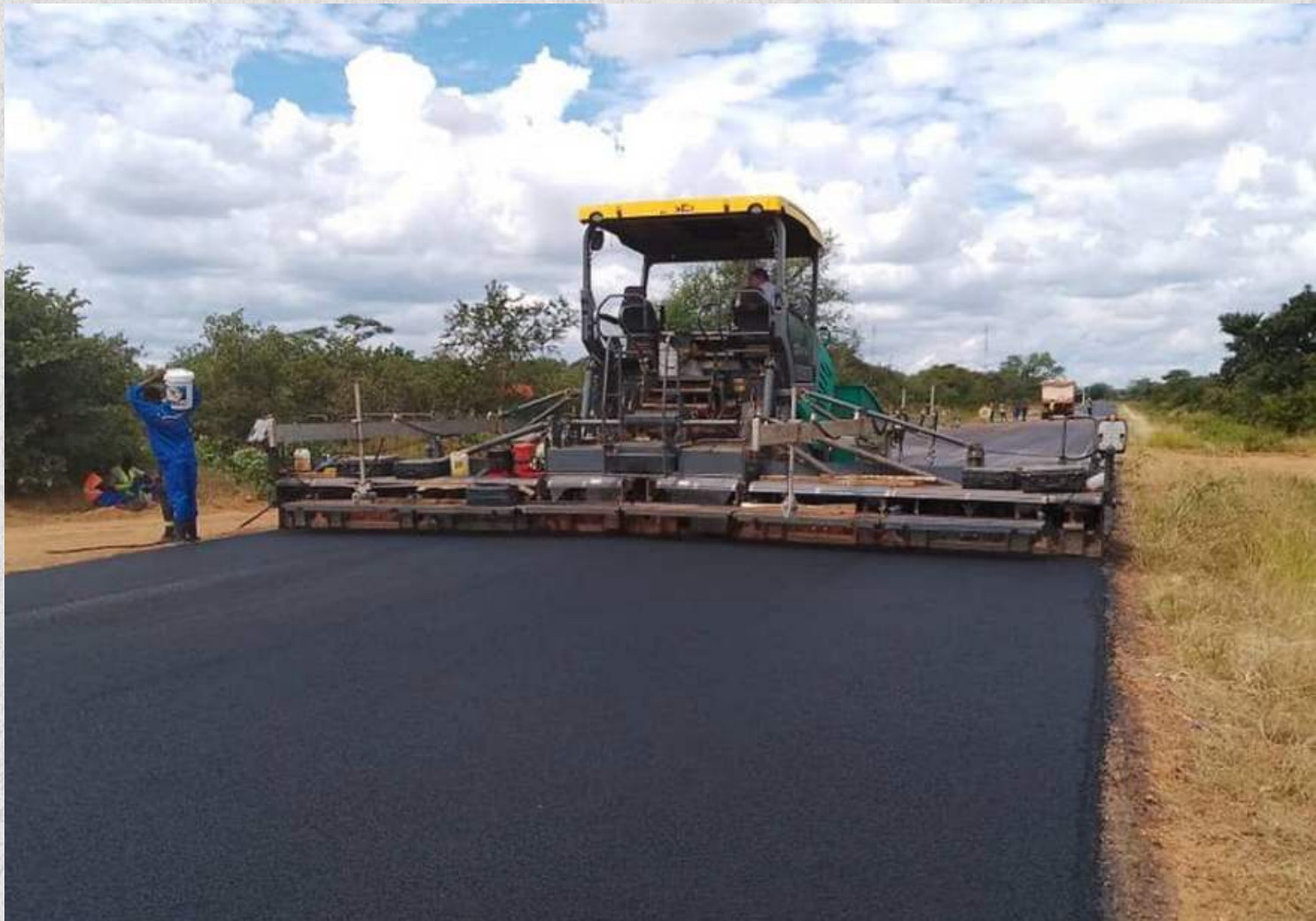
Construction works on the Monze-Niko Road.
