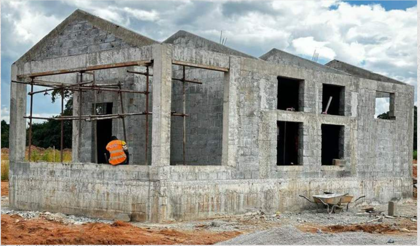
The Chingola-Chililabombwe Weighbridge under construction.
