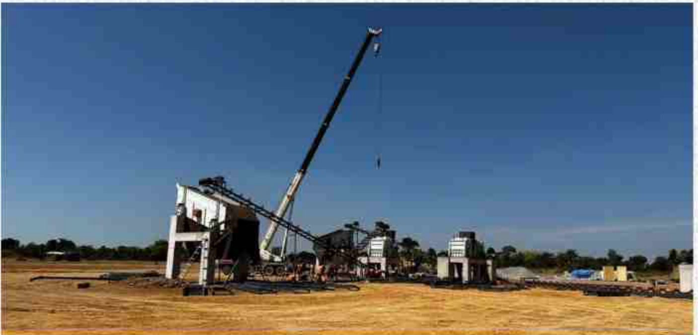
Crusher Plant installation on the Ndola-Mufulira Road Project.
