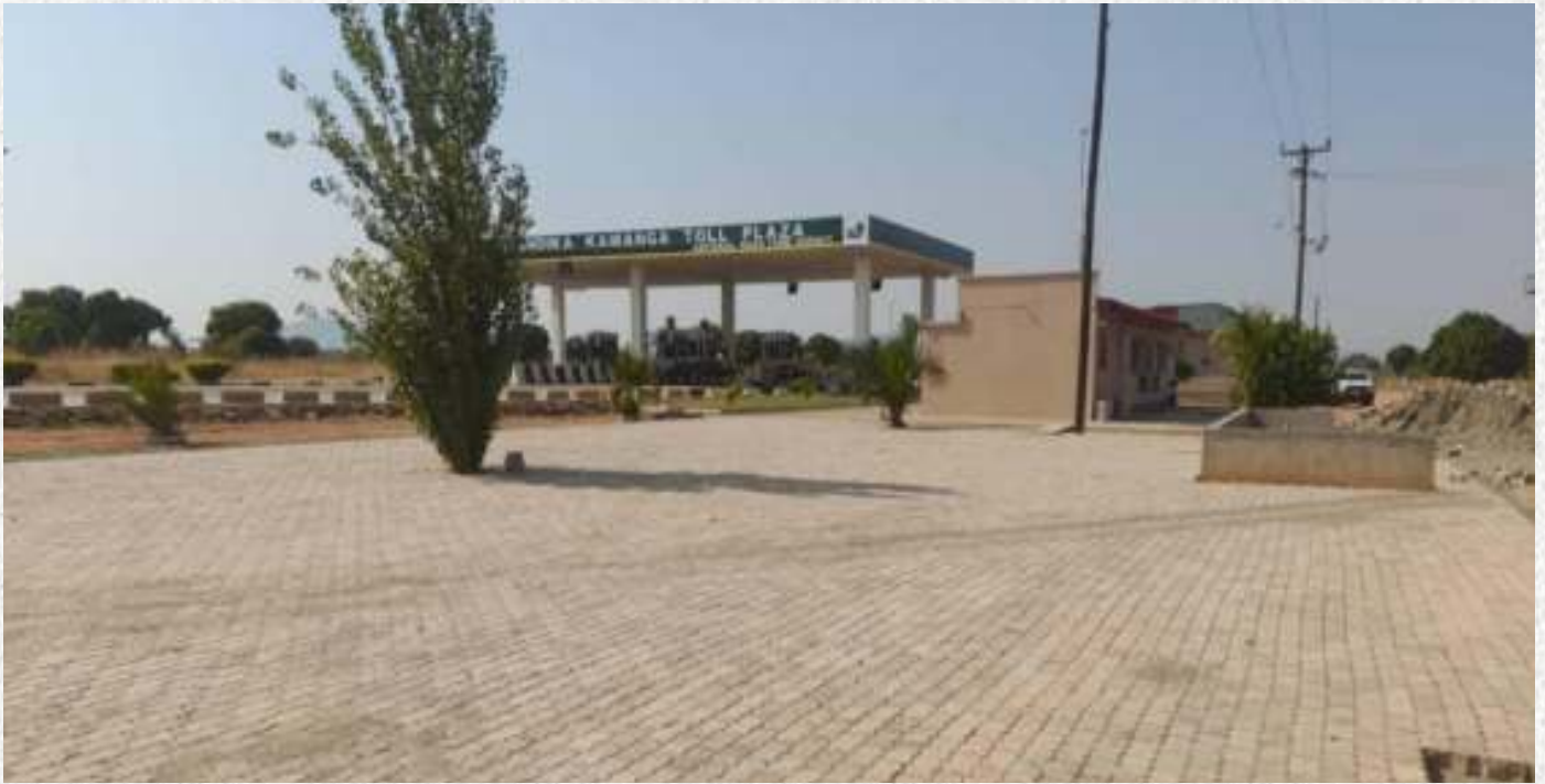
Additional works at Rueben Chitandika Kamanga Toll Station.
