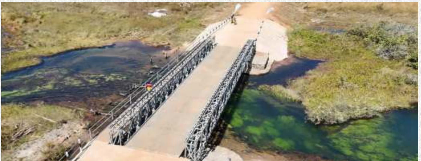
Aerial view of Lukulu ACROW Bridge.
