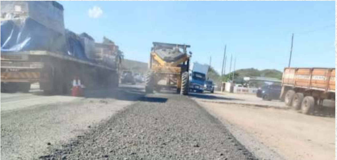
Lusaka-Chilundu Road works.
