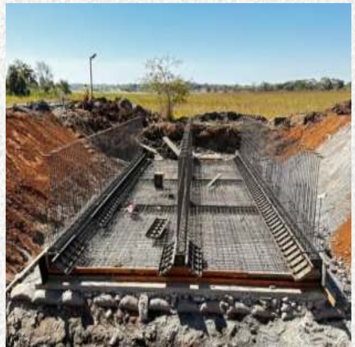
Works on the Masangano-Fisenge-Luanshya Road.
